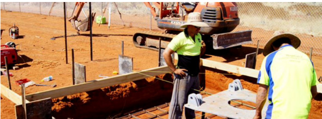
Figure 2 - Solar project under construction, providing jobs in regional Australia
