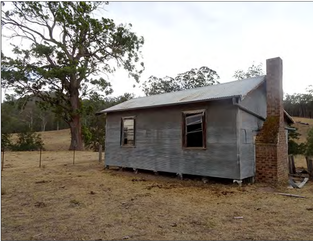
View of Hilliers Creek-HS01.
