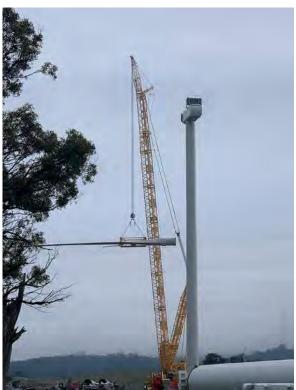
4. A view of the blades being attached to the turbine hub. Note the area needed for material laydown and construction vehicle, such as the crane, and parking (photo source: Vestas, Collector Wind Farm, NSW). This page has intentionally been left blank.
