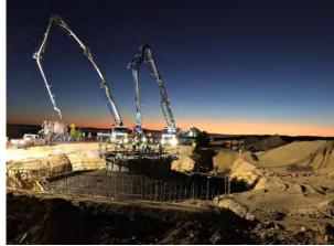
Construction of the turbine foundations involves a localised impact including the area of foundations, as well as soil stockpiles and construction vehicle parking areas (photo source: Vestas, Collector Wind Farm, NSW).
