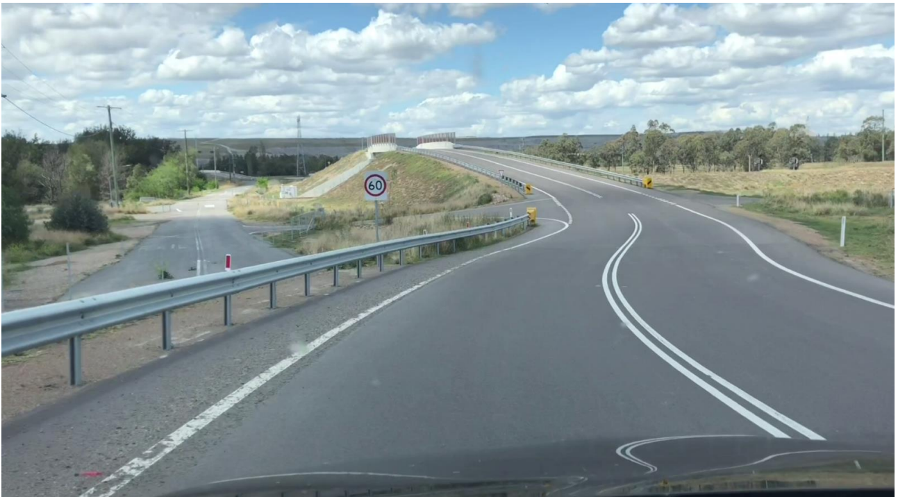
Photo 2 – Looking east on Hebden Road at bridge over ARTC line
