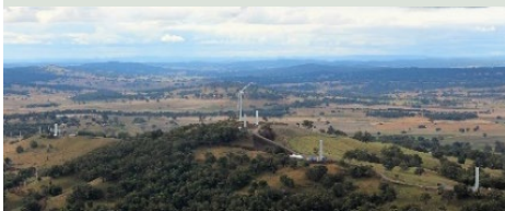
White Rock NSW – 175MW Stage 1 In operation. Stage 2 about to go to construction (CECEP/Goldwind)
