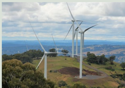
White Rock Wind Farm
