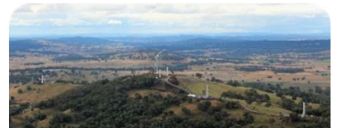
White Rock Wind Farm
