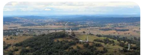
White Rock – 175MW Stage 1 Construction Complete (Goldwind)
