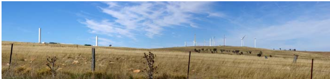
Plate 12 - Illustrating general construction activities at the Capital wind farm site, including views toward cranes, partial construction of towers and laydown areas.
