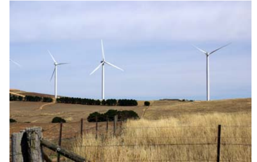
Photo 4 - View toward operational Capital wind turbines.
