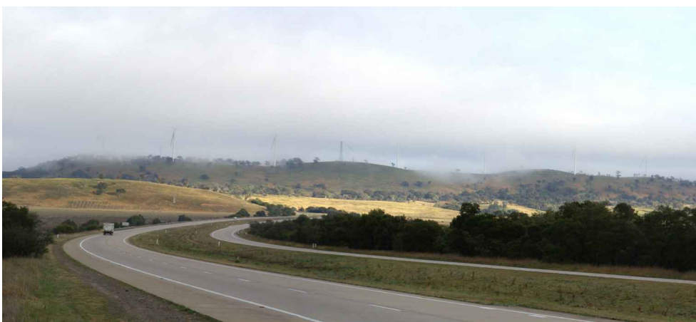
PHOTOGRAPH C - DAY TIME VIEW FROM HUME HIGHWAY TOWARD CULLERIN WIND FARM AT AROUND 3.5KM (7th July 2010)
