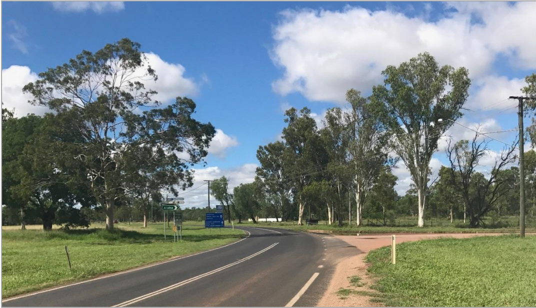
Figure 3 Clermont Connection Rd / Clermont Alpha Rd / Tropic St Intersection
