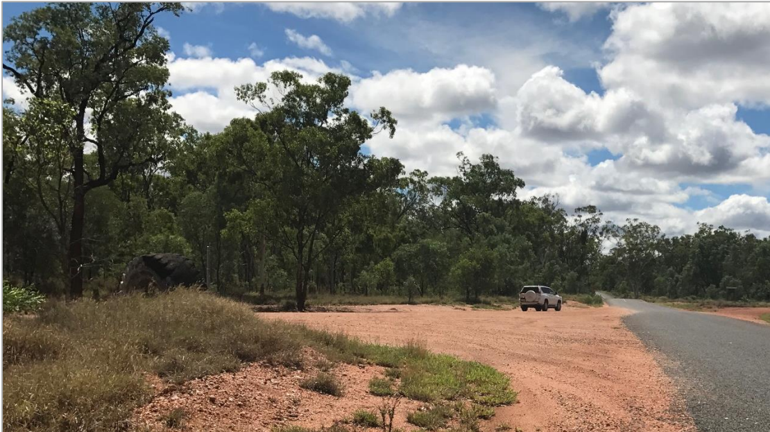
Figure 5 Clermont Alpha Rd / Alpha Bypass Rd Intersection
