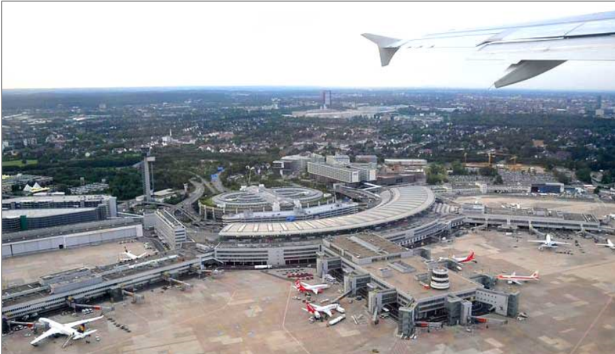
Figure 22 – 8,400 solar panel array on roof of Dusseldorf International Airport, 2011 Source: Solar Choice, www.solarchoice.net.au/blog/solar-panels-near-airports-glare-issue , 2013
