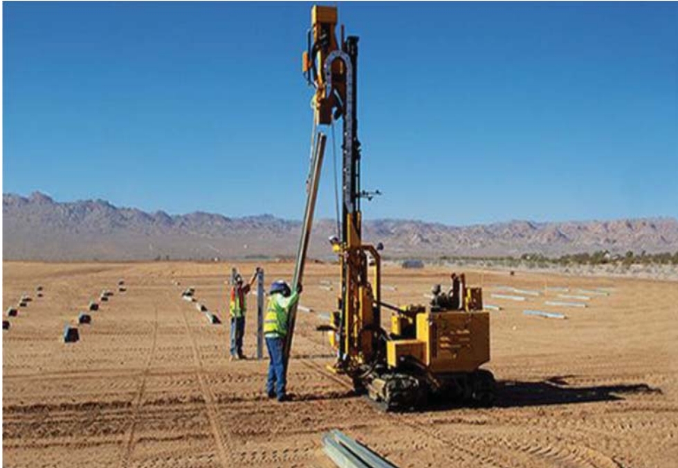
Figure 3-7 Example of poles driven into the ground
