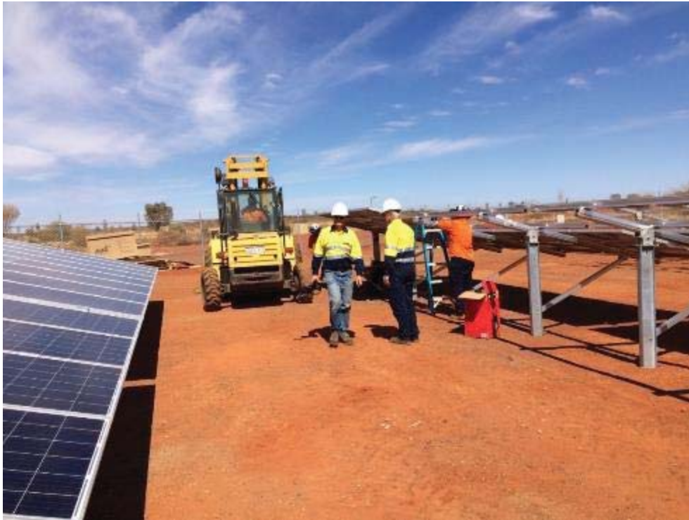
Figure 3-9 Example of module assembly
