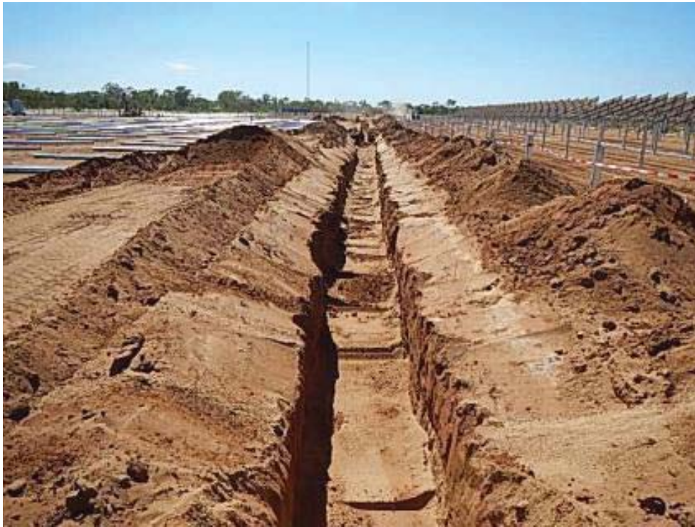
Figure 3-14 Example of cable trench
