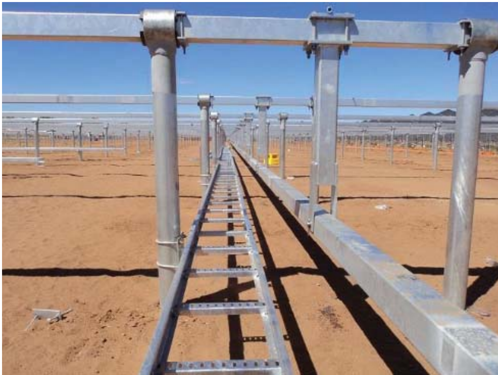
Figure 3-8 Example of tracker mounting system installation
