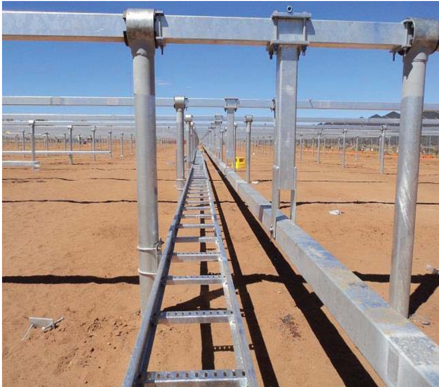
b) Example of tracker mounting system installation
