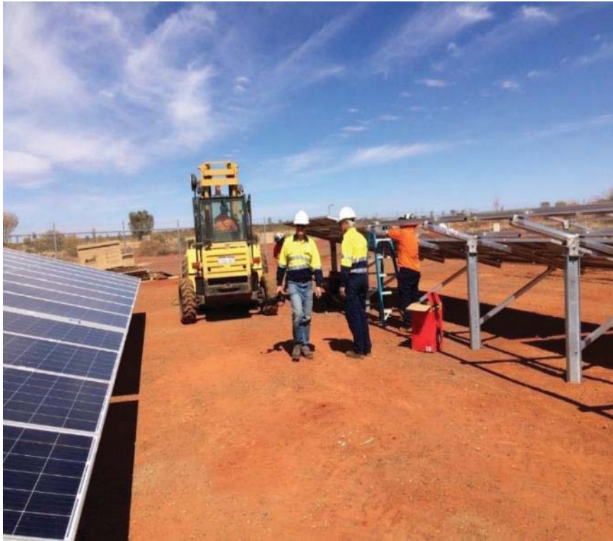
c) Example of array module assembly.
