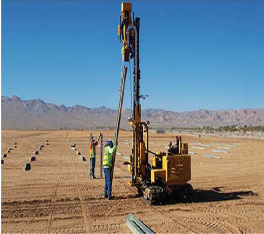
a) Example of poles driven into the ground
