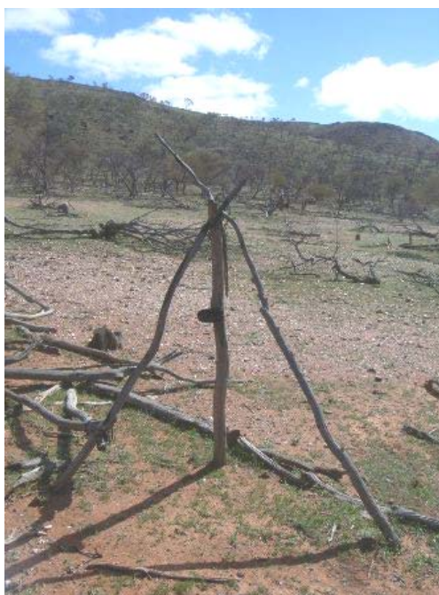
Detail of woodwork structure with tin tacked to post
