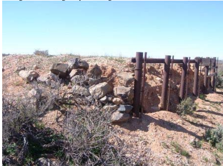
Looking 105° along siding embankment with STW embankment on right
