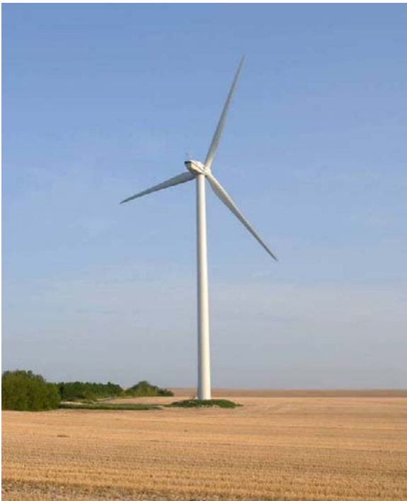
Figure 3.3 Typical wind turbine (82m rotor installed on an 80m tower)
