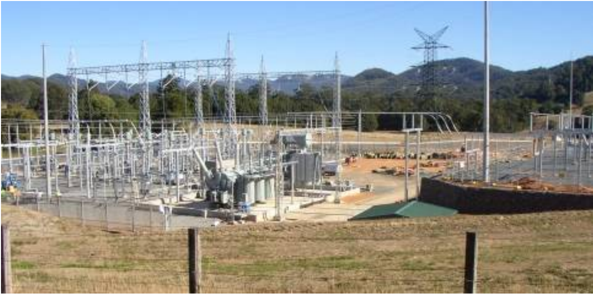
Figure 3.9 Coffs Harbour 330/132kV substation under construction
