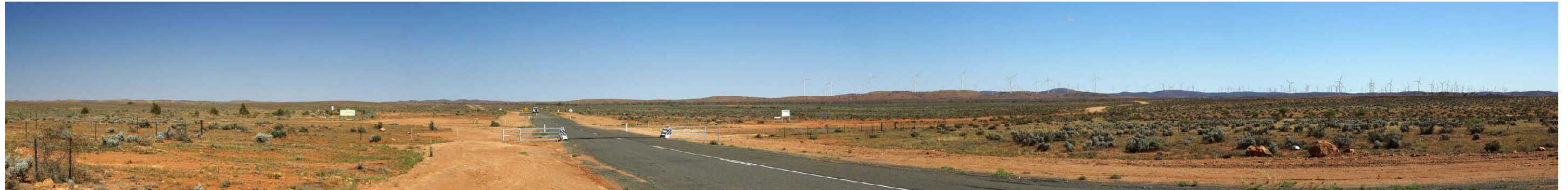
Silverton Road, Daydream Mine Entrance
