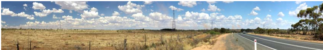
Plate 25 View east as existing 220kV transmission line crosses Sturt Highway around 2km west of Gol Gol.
