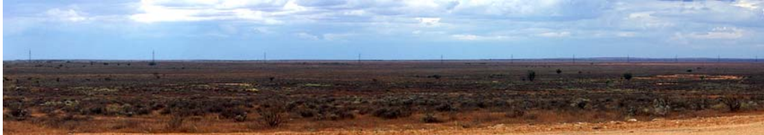
Plate 24 Typical view south around 20km south of Broken Hill illustrating pylons above horizon on generally level ground.
