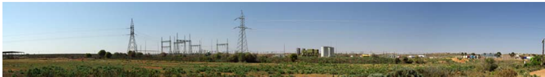
Plate 21, View north toward existing Broken Hill substation within Landscape Unit 9.
