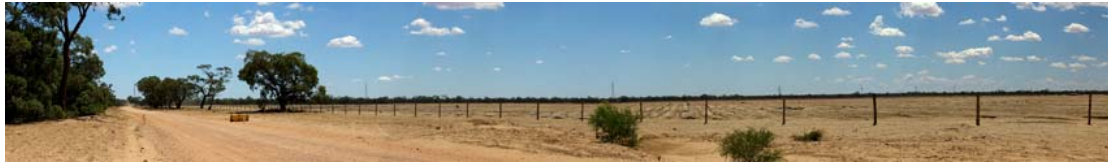
Plate 27 View west along the Lower Darling Road with transmission line extending across agricultural fields.
