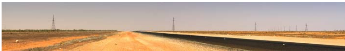
Plate 19, View south toward existing 220kV transmission line crossing Silver City Highway around 16 km south of Broken Hill.
