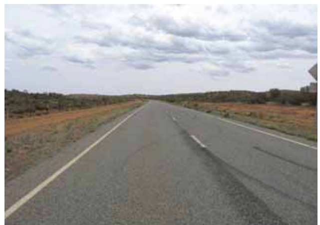
PLATE 24 Nine Mile Road (sealed section)
