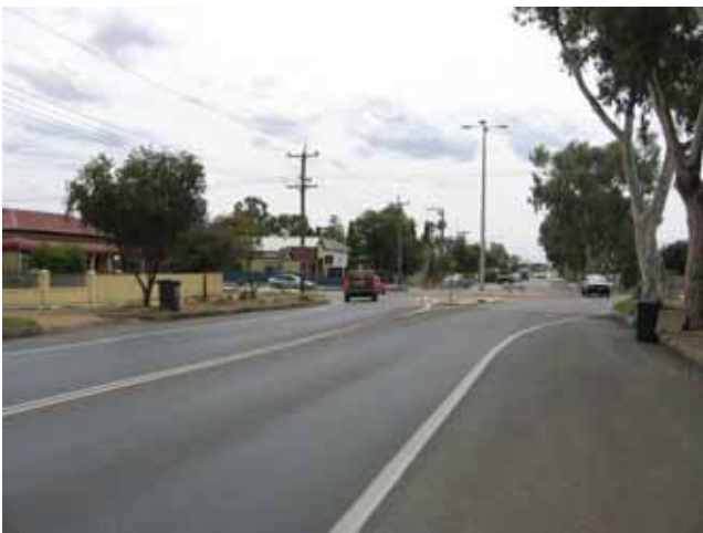
PLATE 21 Kaolin Street roundabout looking northeast
