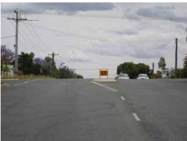
PLATE 23 Pedestrian refuge in Kaolin Street
