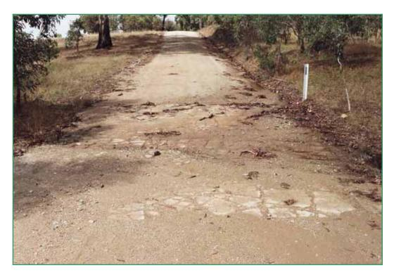
Figure 3.3 Lerida Road North – concrete causeway.
