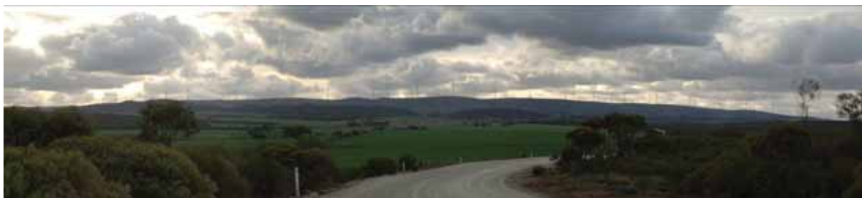
Figure 10.4 Mt Millar Wind Farm at dusk
