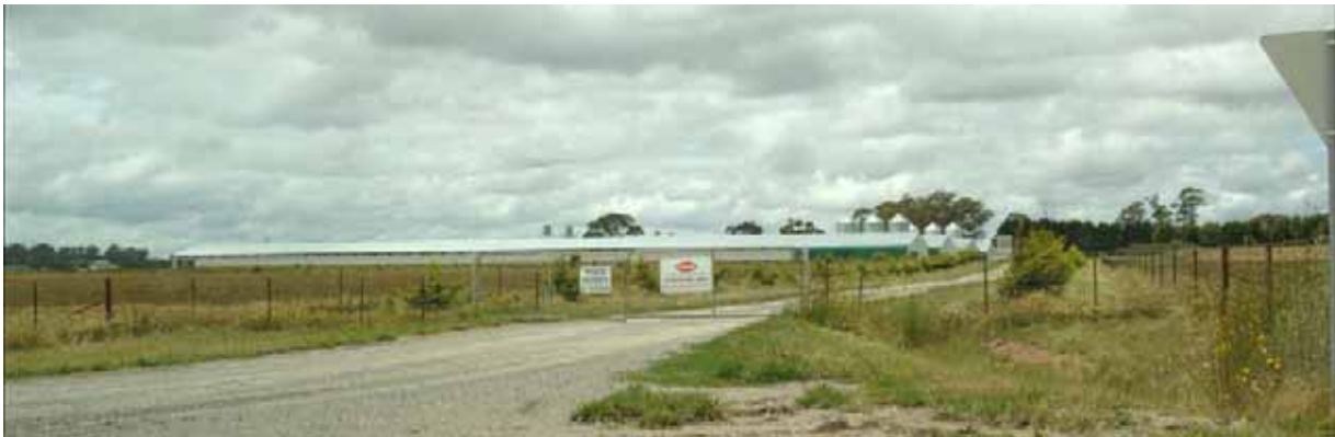
Figure 7.17 View looking east towards the chicken farm
