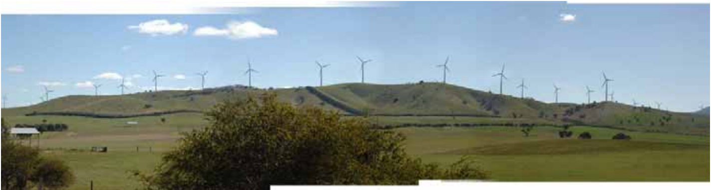
VIEW SHOWING THE ACTUAL AS-BUILT WIND TURBINES.
