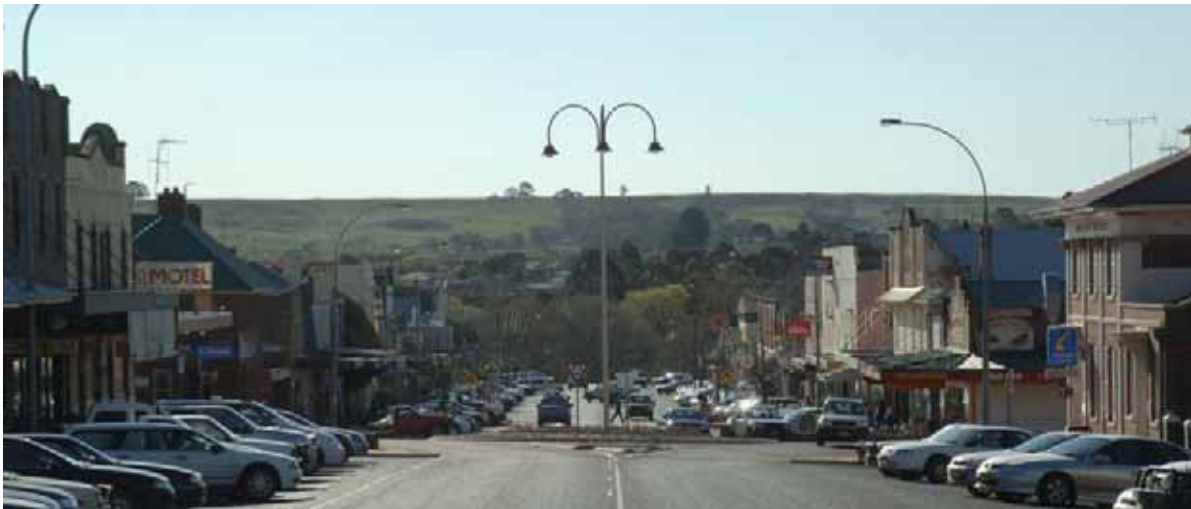
Figure 7.34 Crookwell, looking north west on Goulburn Street
