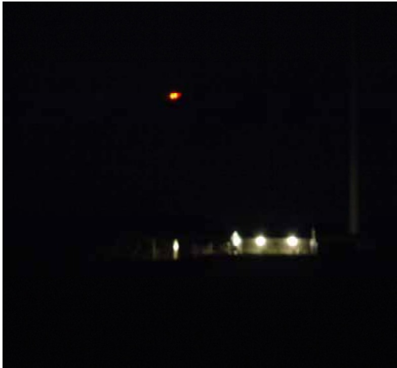
Figure 10.6 Lighting on the substation and a turbine in the background
