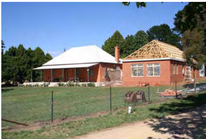
Original cottage and a new extension
