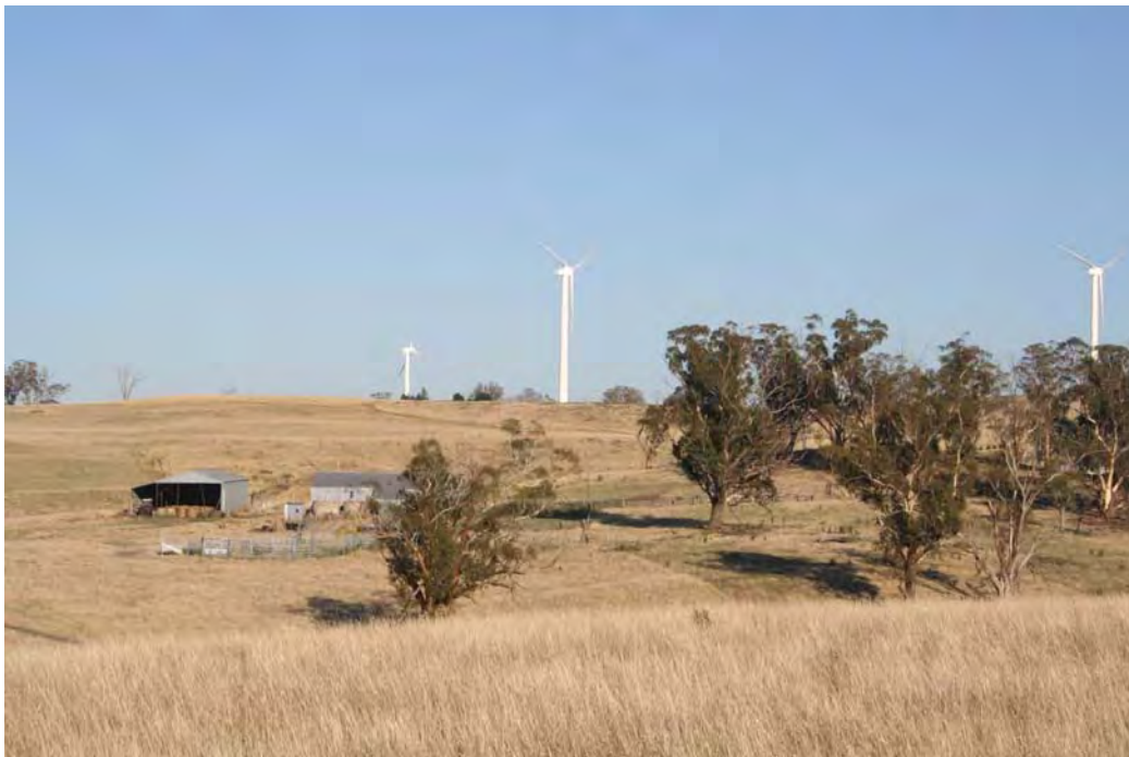
Crookwell wind farm from the viewing area on Goulburn Road
