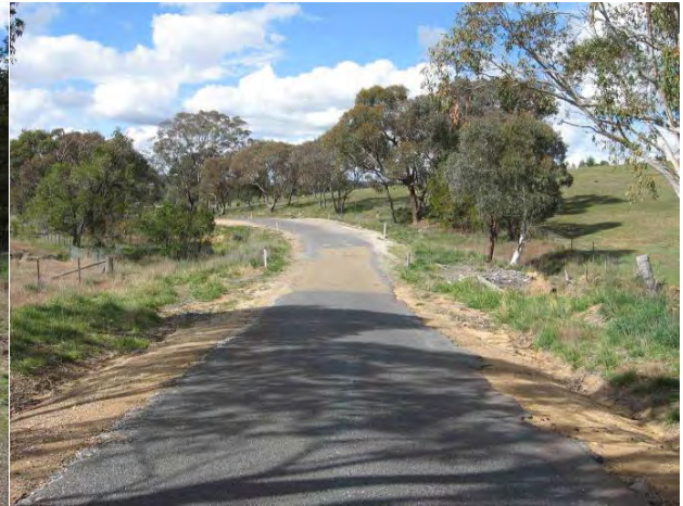
PLATE 34 Gurrundah Road at approx 20km.
