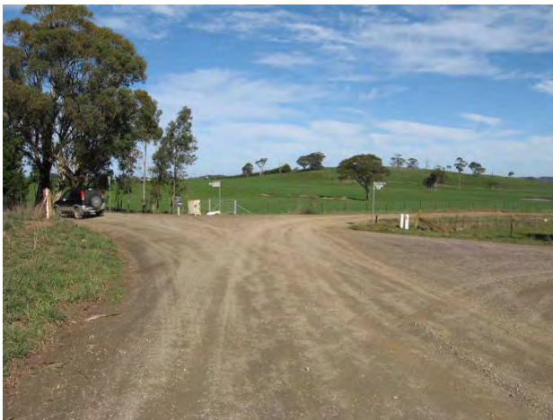
PLATE 47 Prices Lane Junction with Bannister Lane looking south.
