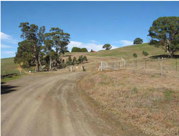
PLATE 45 Storriers Lane at 1.2km.
