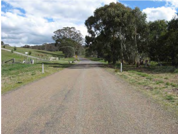
PLATE 33 Gurrundah Road at approx 19km.
