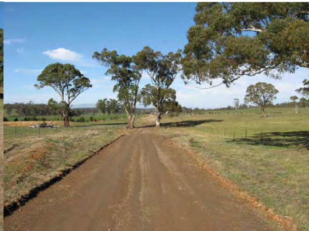
PLATE 46 Storriers Lane at 2.4km.
