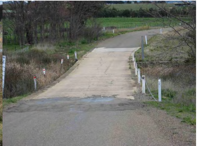
PLATE 32 Gurrundah Road, Concrete Causeway at 15.7km.
