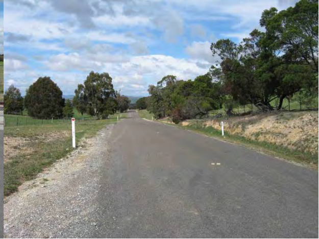
PLATE 44 Breadalbane Route showing width of bitumen.
