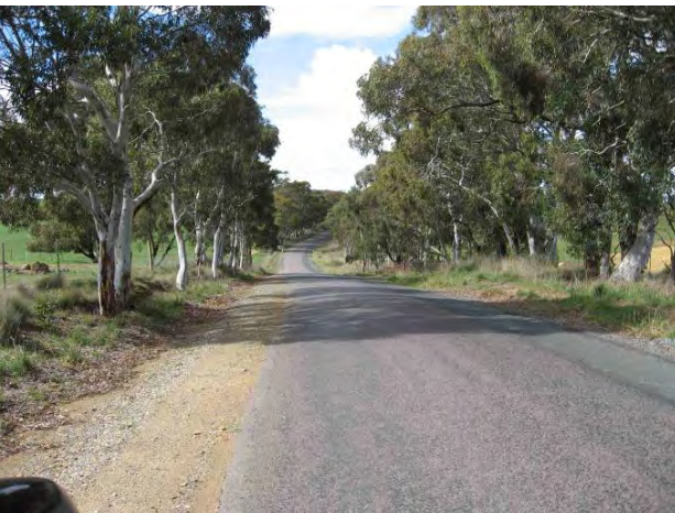
PLATE 41 Gurrundah Road at 28.4km.
