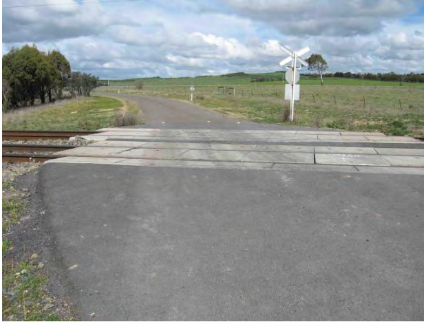
PLATE 43 Breadalbane Route, railway level crossing looking north.
