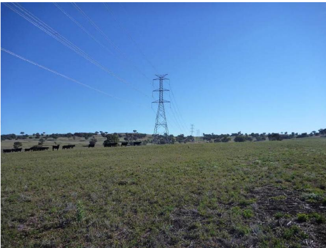
Plate 3-1 - Alternative substation location adjacent to TransGrid 330kV transmission line
