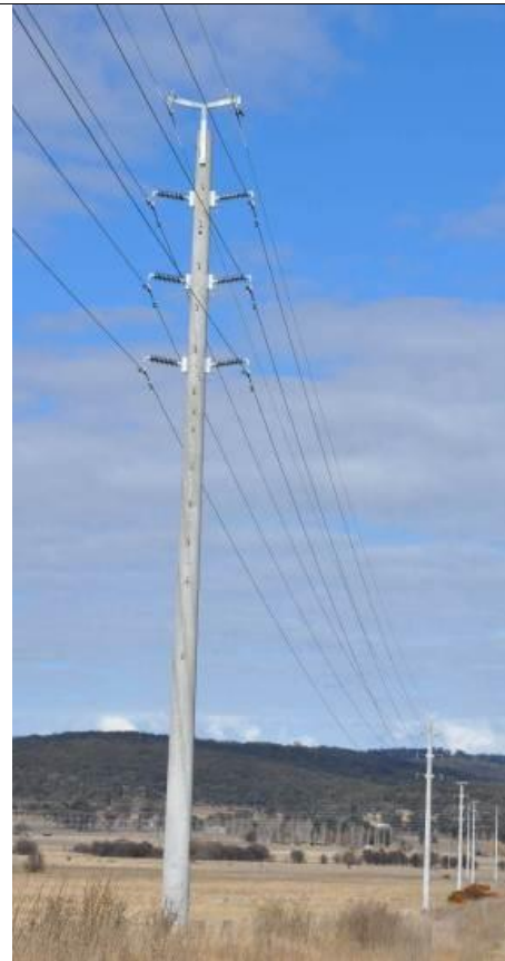
Plate 1.2 Typical double circuit, single pole line
