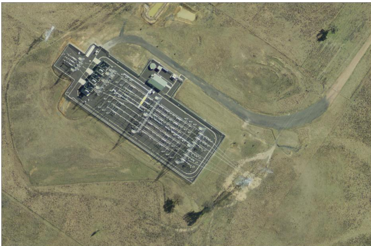
Plate 3.3 – Aerial view of Example Single Transformer Substation in a rural location
