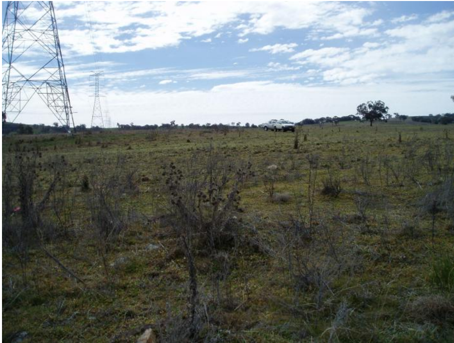
Plate 1-Section 1 -View of the approximate location of the proposed substation and switchyard site within Section 1 of the study area. This site is totally cleared of all indigenous vegetation. This area also forms part of a cultivation area namely for lucerne crops. This site locale is the western extremity of the study area with the alternative grid connection linking to the adjacent 330kV powerline lattice tower facilities conspicuous within the photo.
