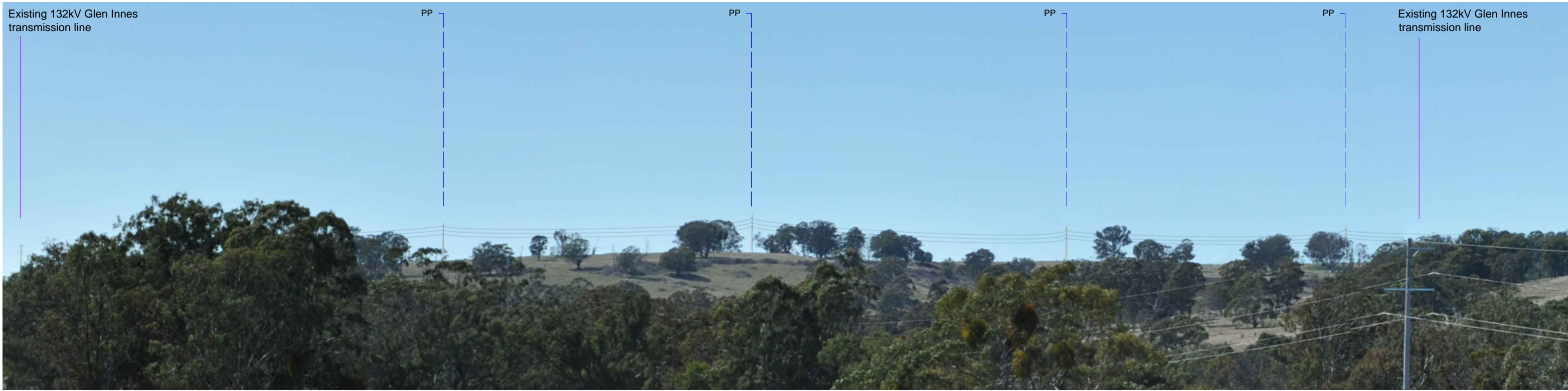
Image 2b Photomontage location Gwydir Highway - view toward the modified 132kV transmission line route
