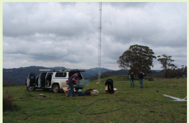
Installation of new site wind monitoring mast
