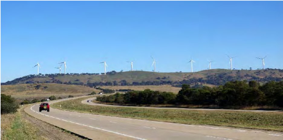
DAY TIME VIEW FROM HUME HIGHWAY TOWARD CULLERIN WIND FARM AT AROUND 3.5KM (13th June 2010)
