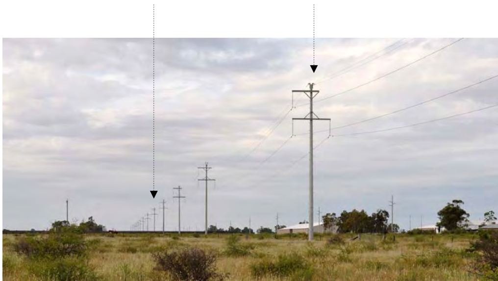
Plate 9 - Existing typical 132kV single pole supporting structure
