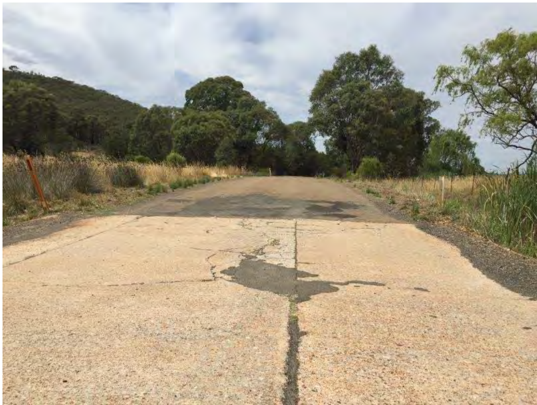
S012 – View to North
