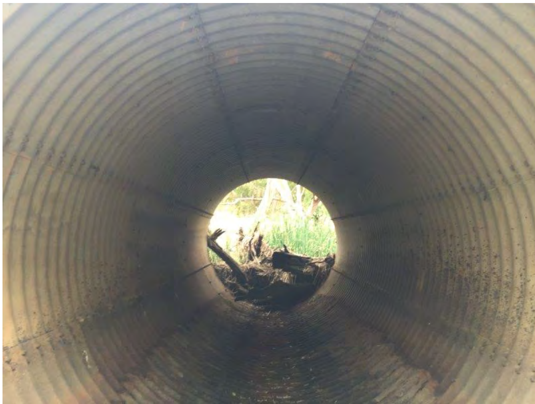
S006 – Internal View
