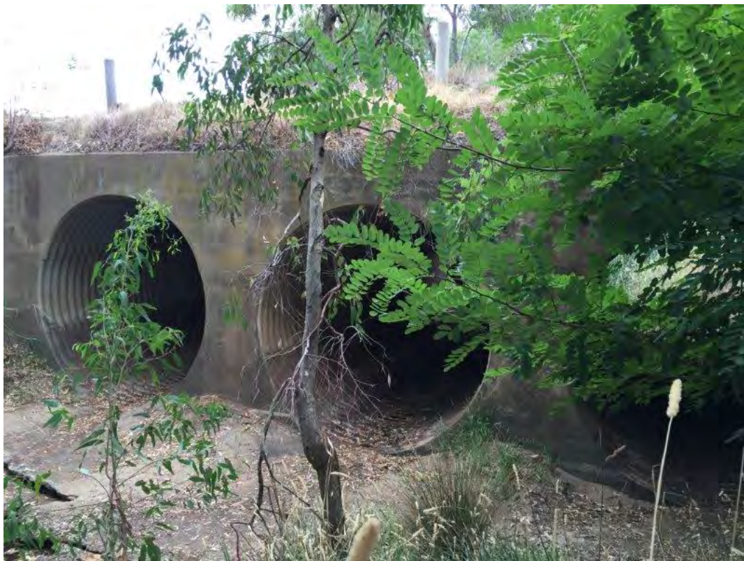
S006 – View from North
