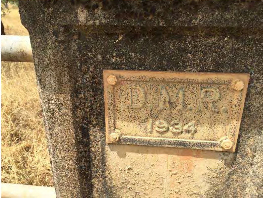
S010 – Bridge Label
