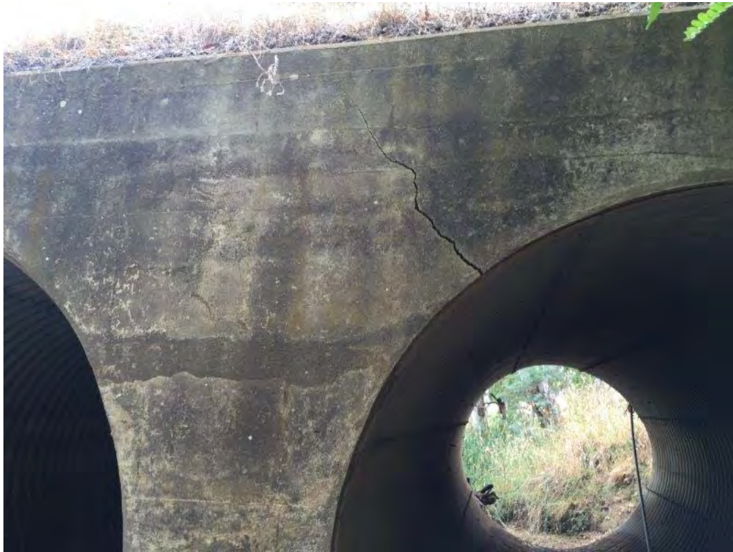
S006 – Northern Headwall
