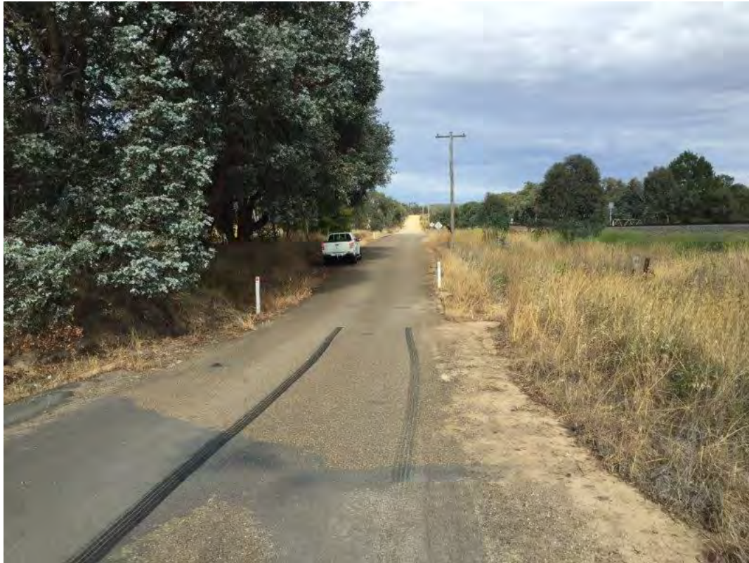
S002 – Causeway, View to West
