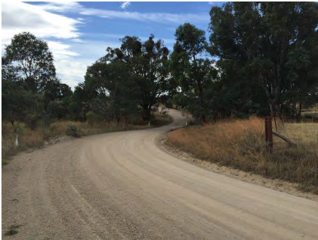
S003 – View from North
