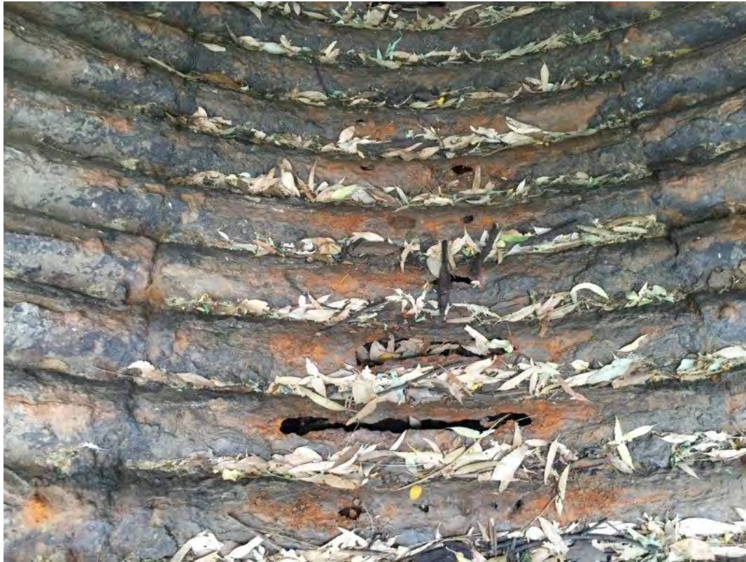
S006 – Invert Condition - Typical
