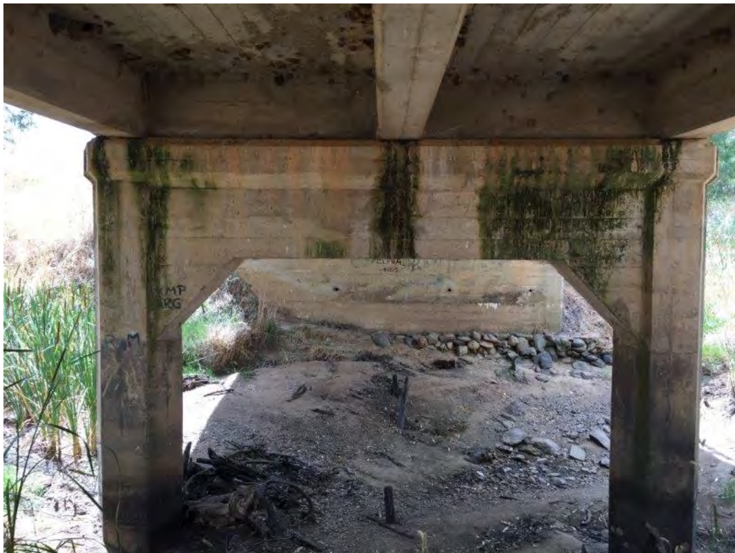
S010 – Bridge Soffit View
