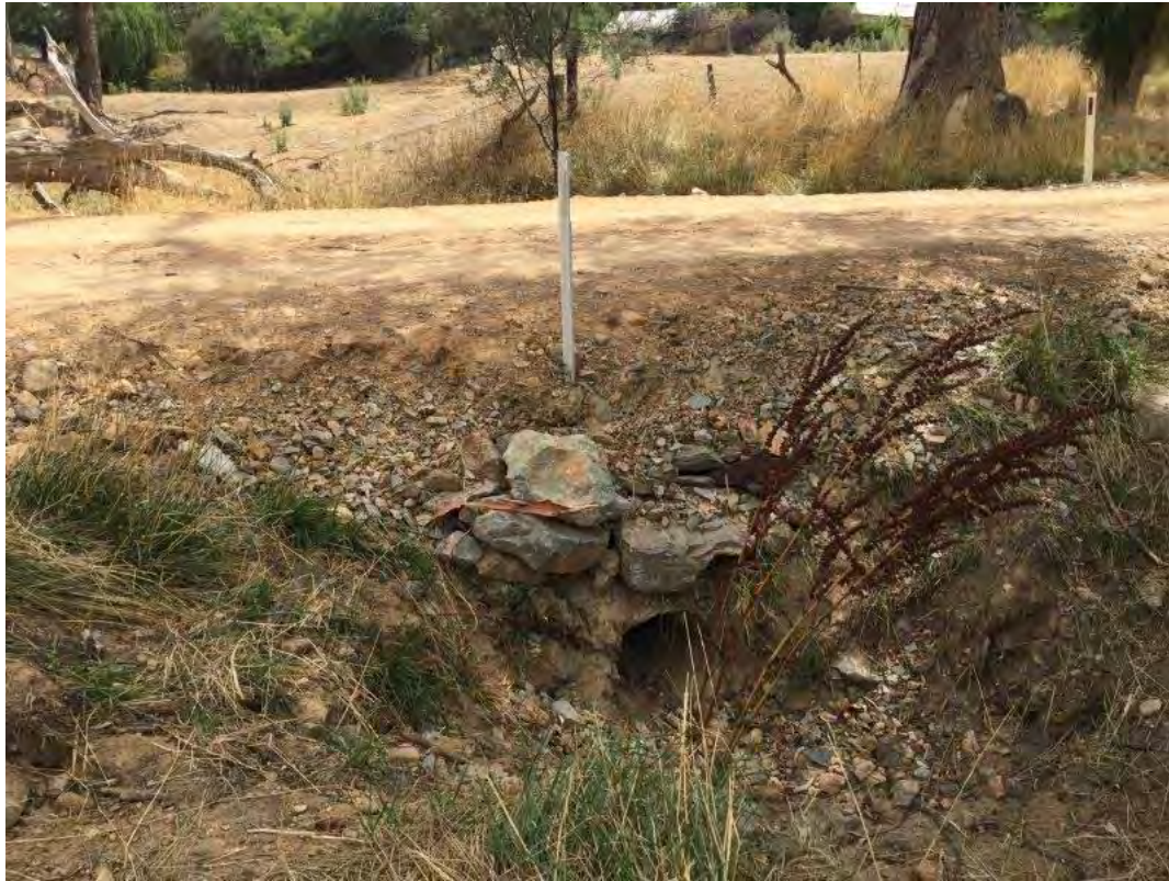
S013 – View from North
