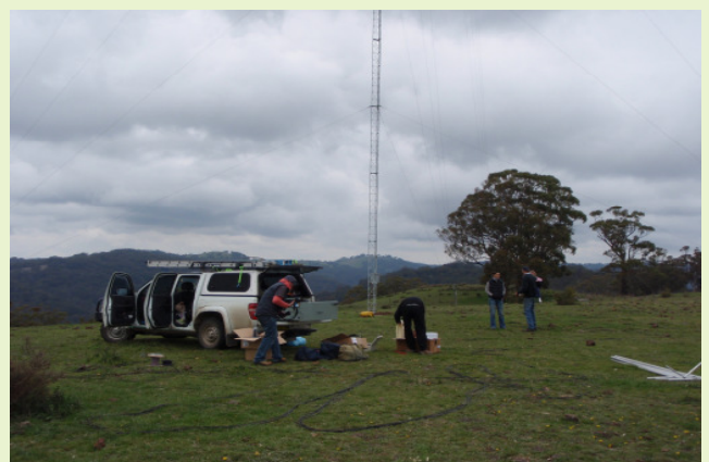
Installation of new site wind monitoring mast
