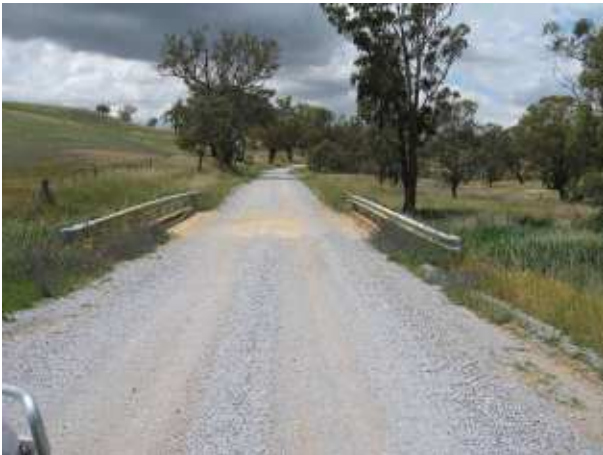
PLATE 99 Garry Owen Road culvert at 8.28km.
