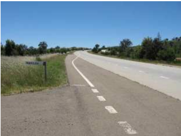
PLATE 29 Marilba Access/Hume highway at 23.0km.
