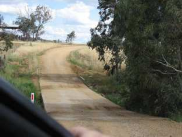
PLATE 103 Westbourne Road at 0.05km.
