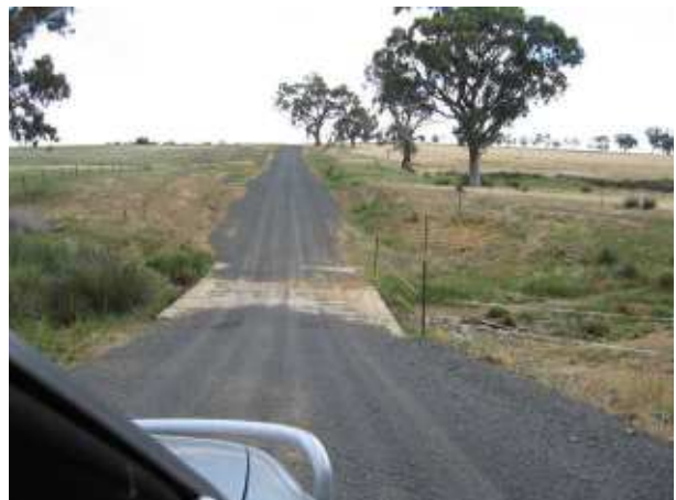
PLATE 72 Coppabella Road causeway at 12.50km.
