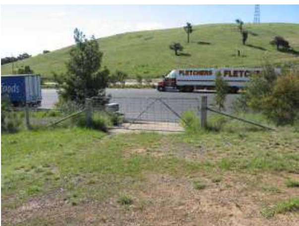
PLATE 41 Westbound rest area Conroy's Gap.
