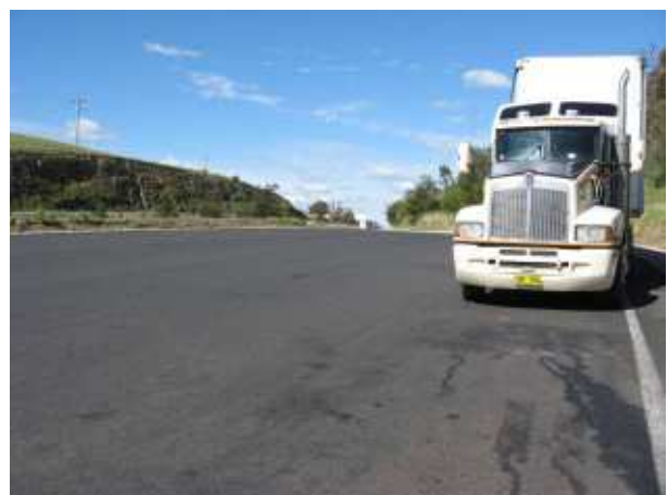
PLATE 42 Westbound rest area Conroy's Gap.
