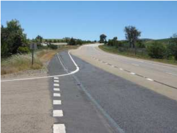
PLATE 31 Marilba Access/Hume highway at 23.0km.
