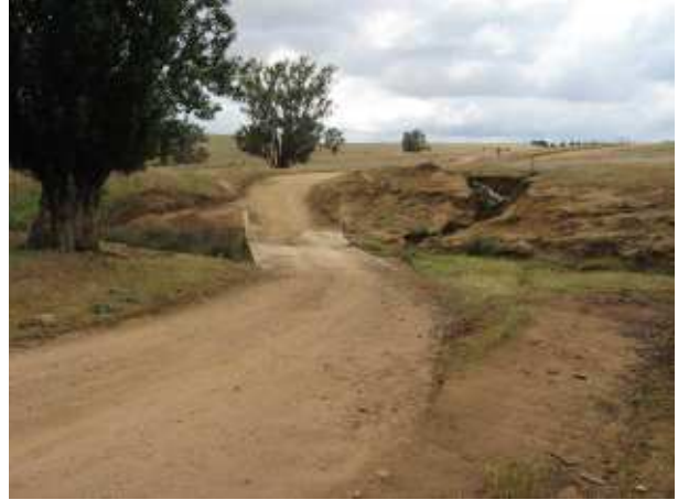
PLATE 86 Cumbamurra Road causeway at 3.64km.
