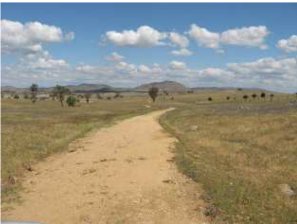
PLATE 69 Coppabella Road at 7.83km.
