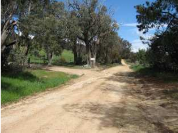
PLATE 25 Waterview Road access on left at 14.6km.
