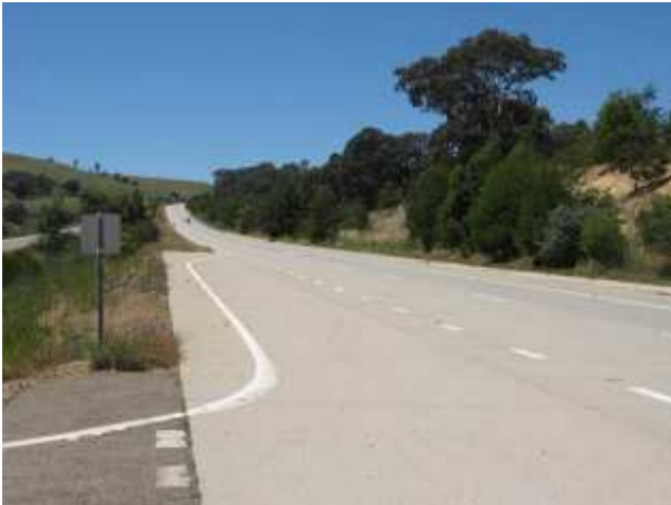
PLATE 37 Marilba Access/Hume highway at 25.2km.
