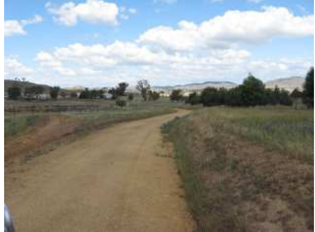
PLATE 68 Coppabella Road at 7.3km.
