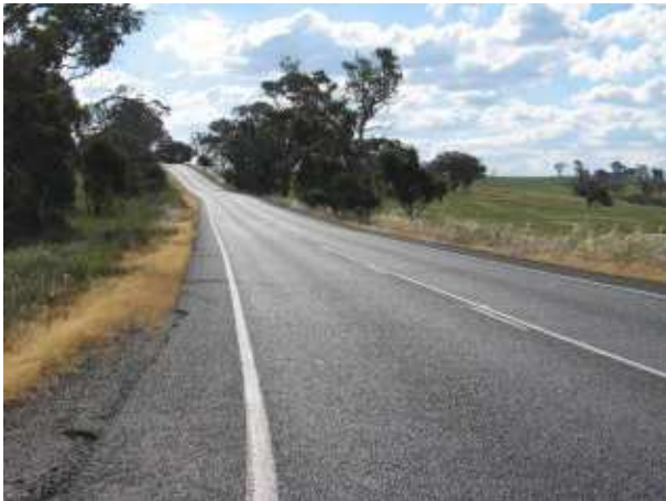
PLATE 2 Burley Griffin Way at 6.5km.
