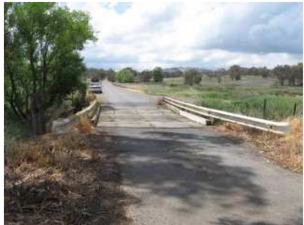
PLATE 96 Garry Owen Road Bridge at 0.69km.
