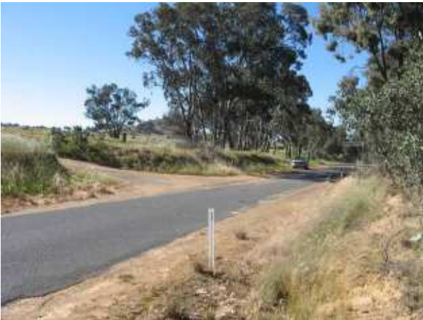
PLATE 9 Illalong Rd/ Cambbells Road at 8.5km.
