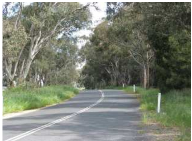
PLATE 18 Burrinjuck Road Trees over road.
