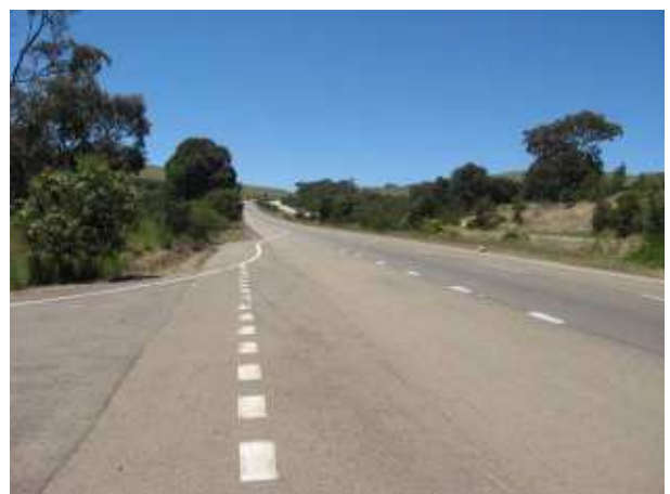
PLATE 36 Marilba Access/Hume highway at 25.2km.
