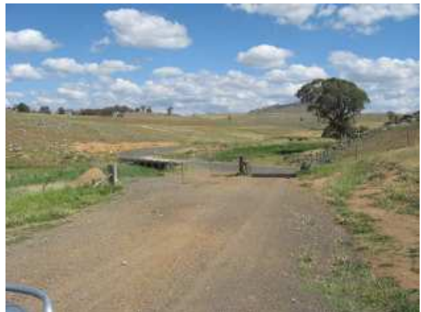
PLATE 70 Coppabella Road low level bridge ahead.
