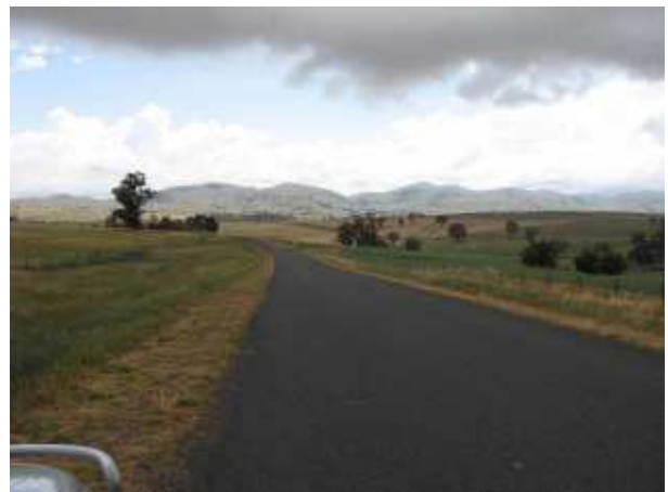
PLATE 78 Berramangra Road at 1.1 km.
