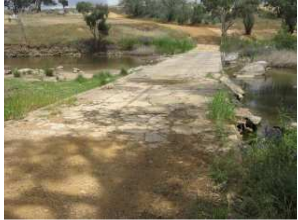
PLATE 92 Coppabella Road Nth causeway at 1.0km.
