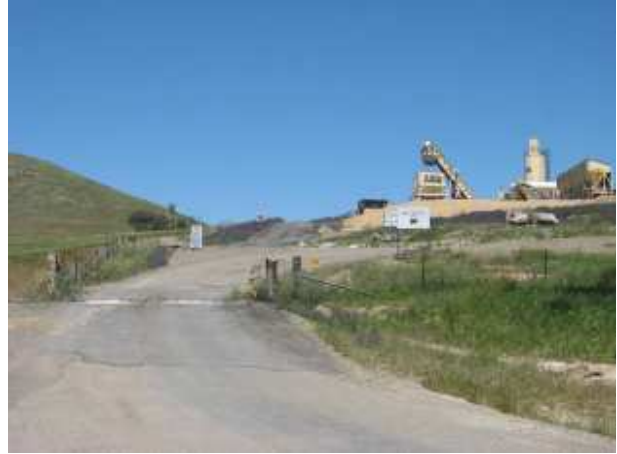
PLATE 14 Paynes Rd/Quarry Entrance.
