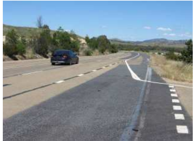
PLATE 32 Marilba Access/Hume highway at 23.0km.
