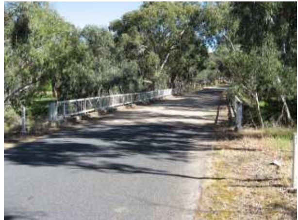
PLATE 10 Illalong Road Conc. Bridge at 10.27.
