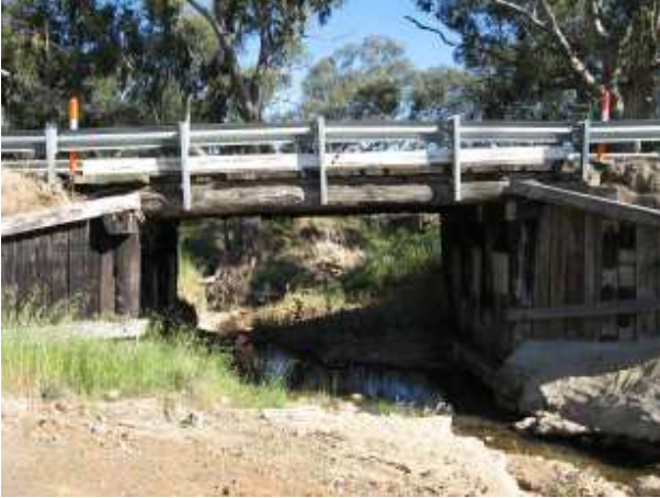
PLATE 7 Illalong Road Bridge at 3.13km.
