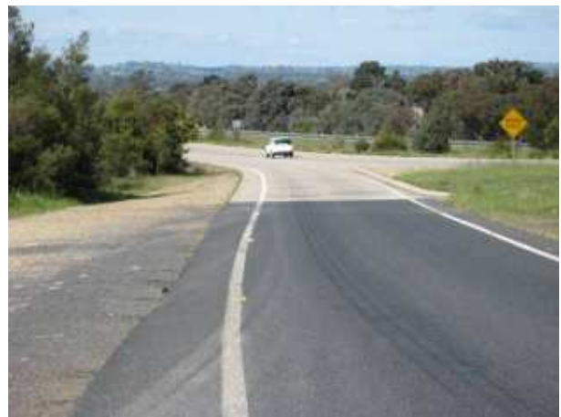
PLATE 40 Eastbound rest area Conroy's Gap.
