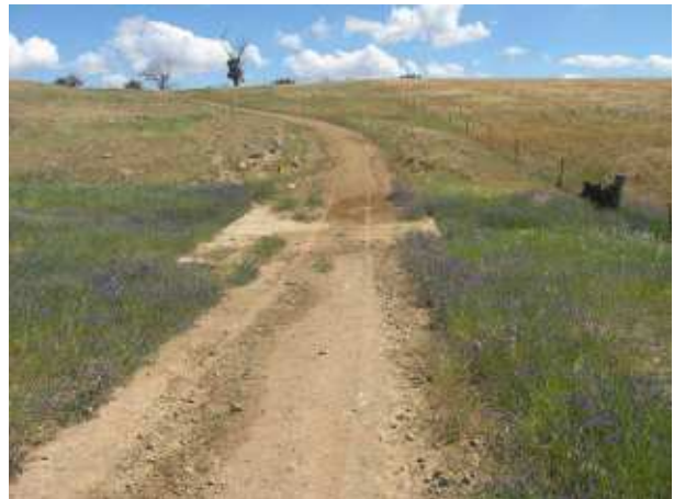
PLATE 66 Coppabella Road stream crossing 5.93km.
