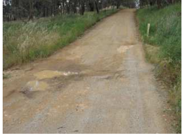
PLATE 98 Garry Owen Road causeway at 3.54km.
