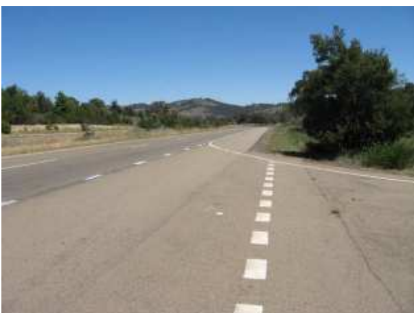
PLATE 35 Marilba Access/Hume highway at 25.2km.
