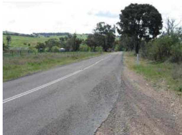
PLATE 22 Burrinjuck Road Junction with Waterview Rd.
