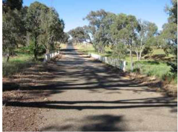
PLATE 8 Illalong Road Bridge at 6.09 km
