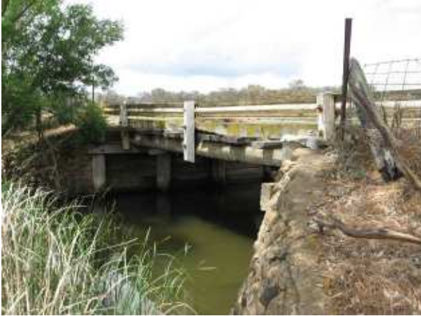
PLATE 97 Garry Owen Road Bridge at 0.69km.
