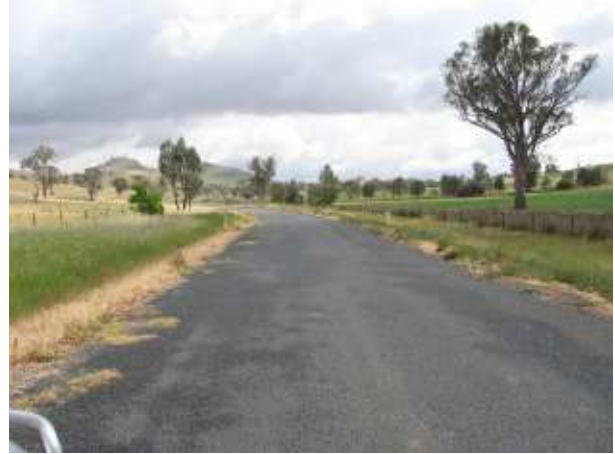
PLATE 80 Berramangra Road at 4.32km.
