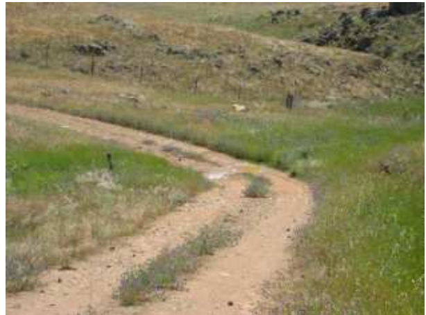
PLATE 64 Coppabella Road at 3.60km.
