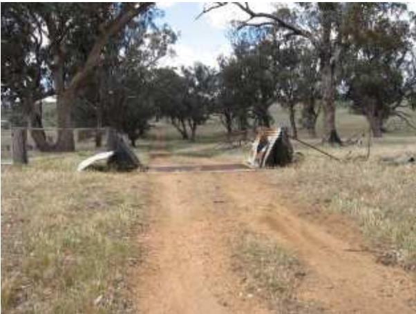
PLATE 63 Coppabella Road at 3.34km.
