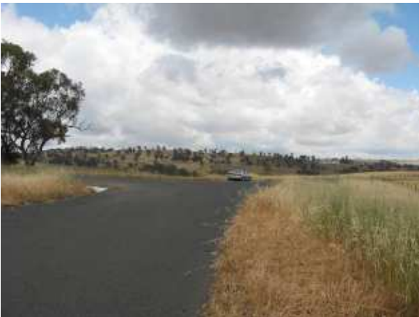
PLATE 83 Berramangra Rd/Westbourne Road junct.
