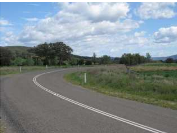
PLATE 23 Burrinjuck Road Junction with Waterview Road
