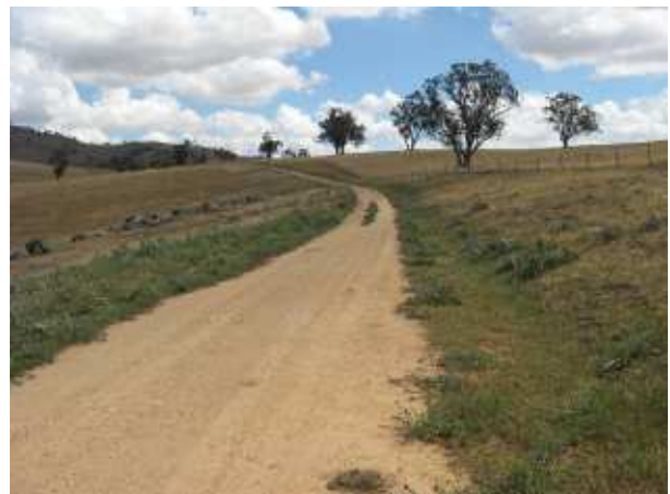
PLATE 60 Coppabella Road at 0.30km.
