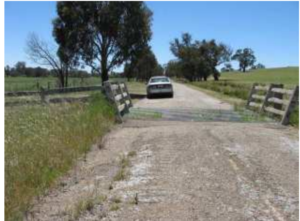
PLATE 38 Marilba Access/Grid at 0.19km looking Nth.
