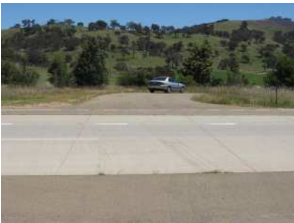
PLATE 33 Marilba Access/Hume highway at 23.0km.
