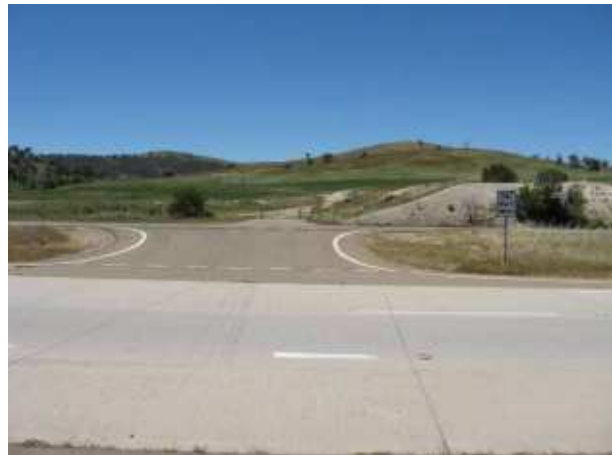
PLATE 30 Marilba Access/Hume highway at 23.0km..
