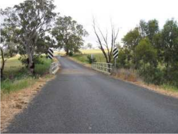
PLATE 79 Berramangra Road Bridge at 3.59km.
