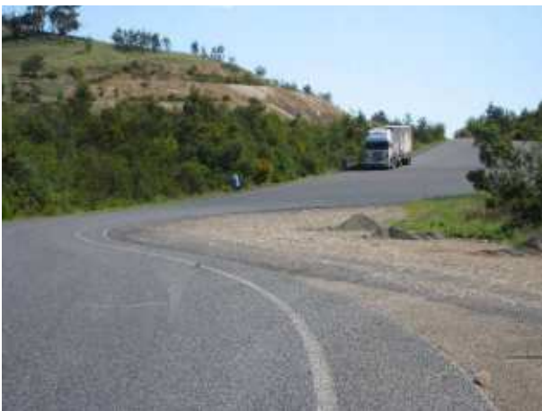
PLATE 39 Eastbound rest area Conroy's Gap.
