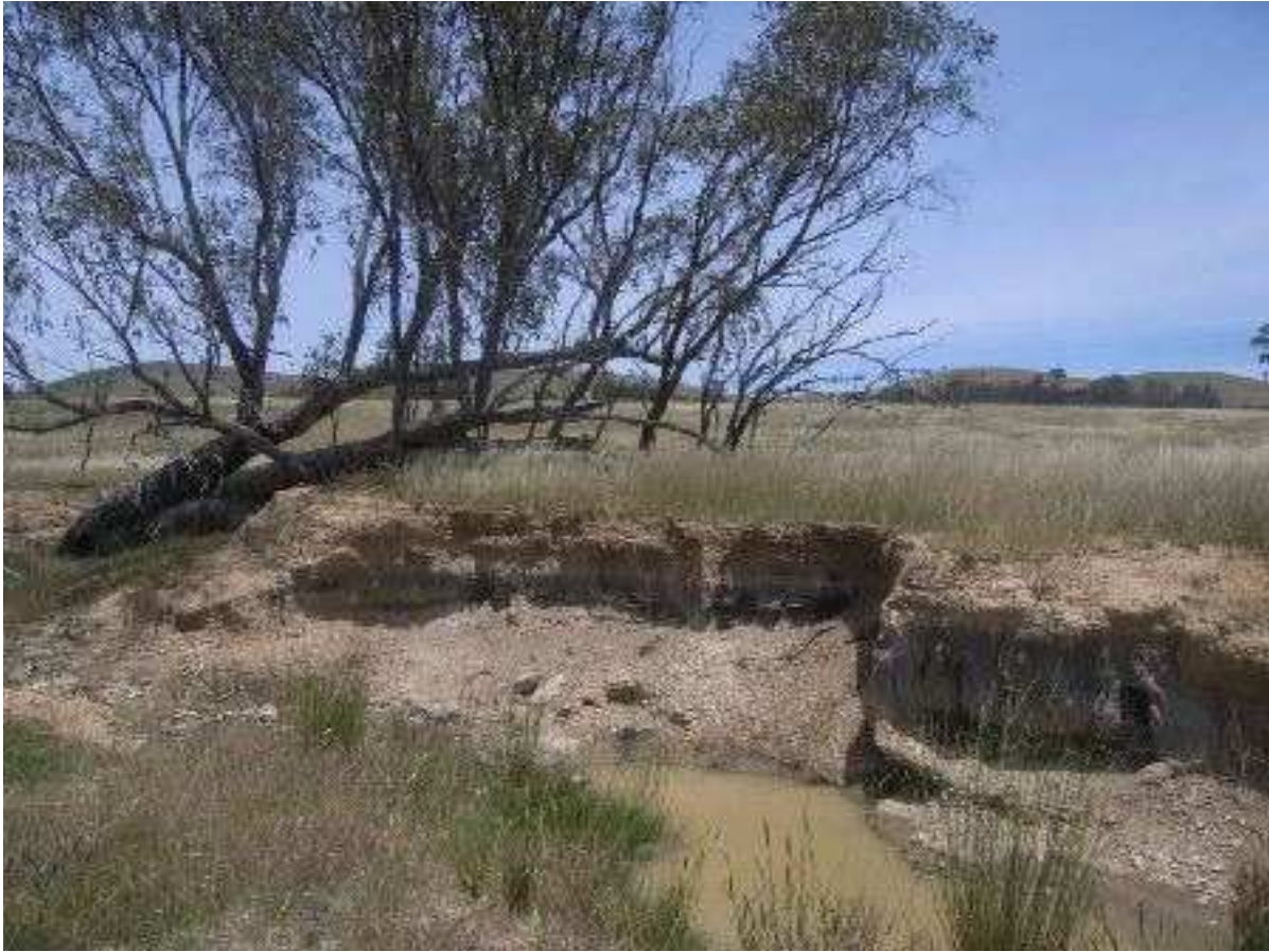
Plate 2. Channel incision in a drainage depression on the 'Marilba' property. This erosion is almost certainly a post European phenomenon. Note also the top yellow-brown soil layer visible in the channel section which is probably Post Settlement Alluvium deposited after the erosion of hillslopes.
