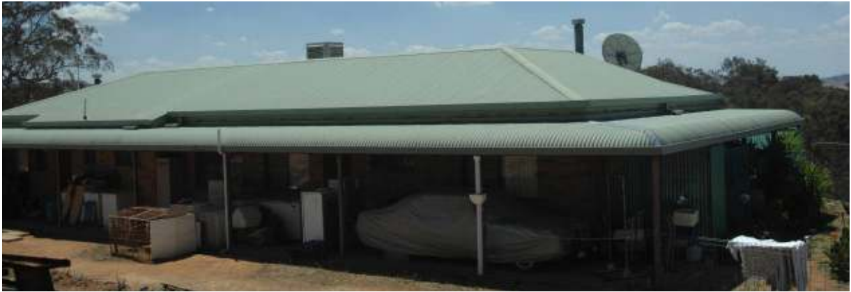
Figure 9.34 The rear of the house
