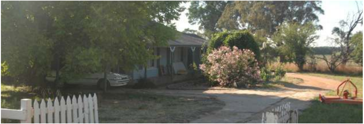
Figure 9.3 “Tullyvale Hall”, view of front of house
