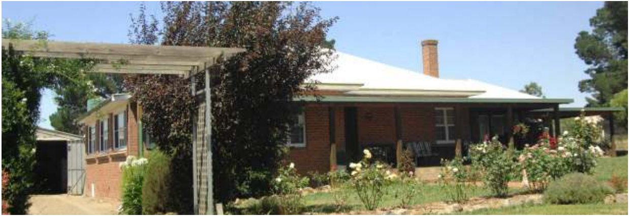
Figure 9.21 “Fairview”, view of front of house
