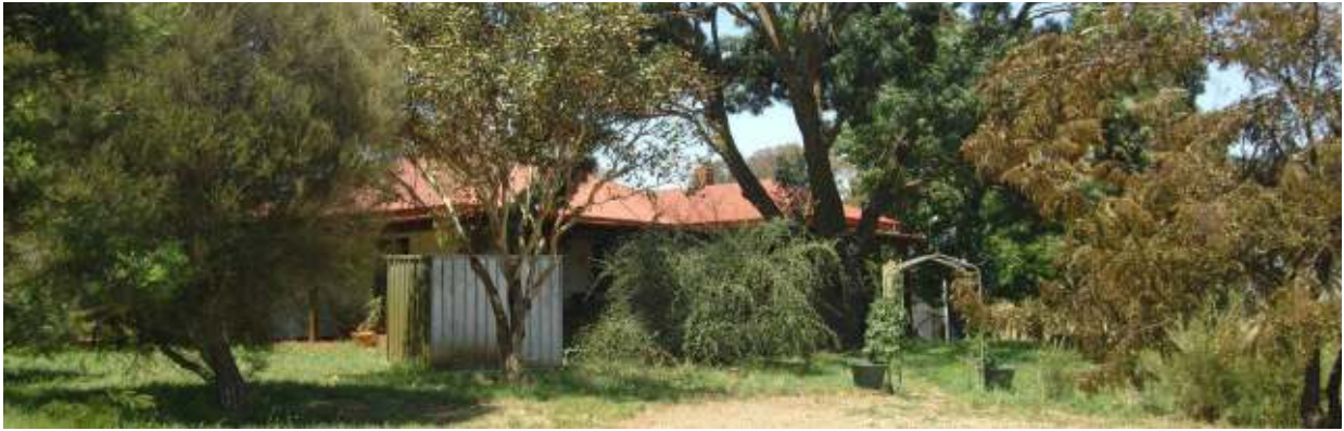
Figure 9.30 “Deepwater”, view of front of house
