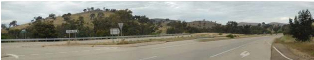
Figure 7.24 View looking north-east across the Hume Highway
