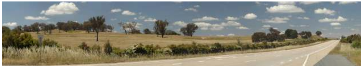
Figure 7.40 View looking north and east along the Hume Highway
