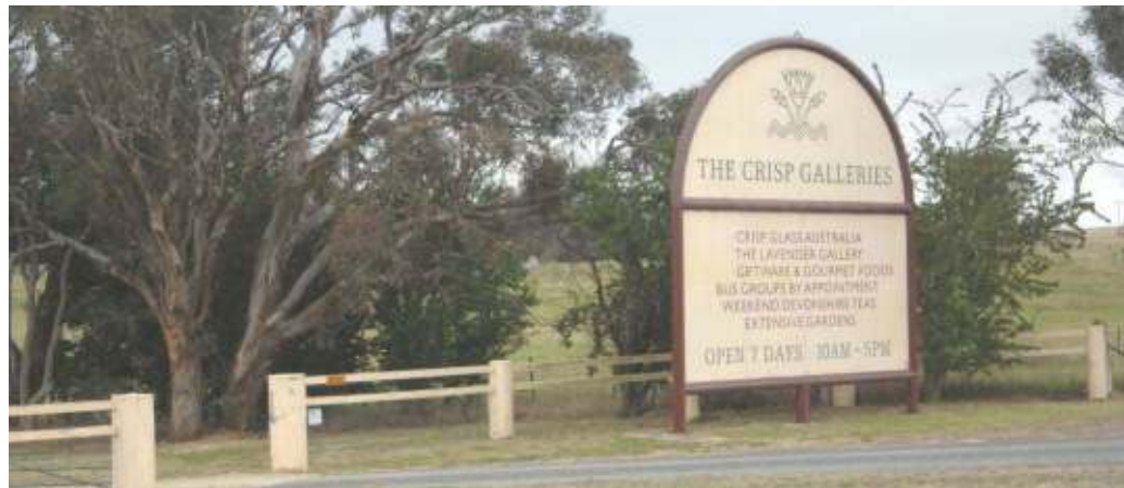
Figure 7.8 Entrance to "Crisp Galleries"
