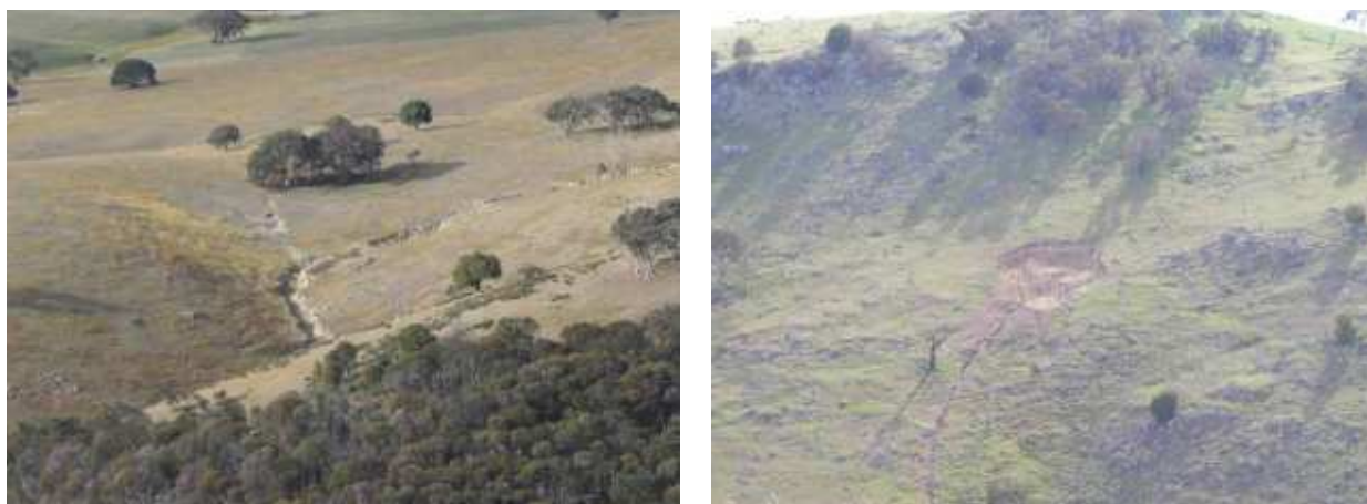
Erosion gully in the foothills of the Coppabella Hills Precinct Erosion on side slope within Coppabella Hills Precinct
