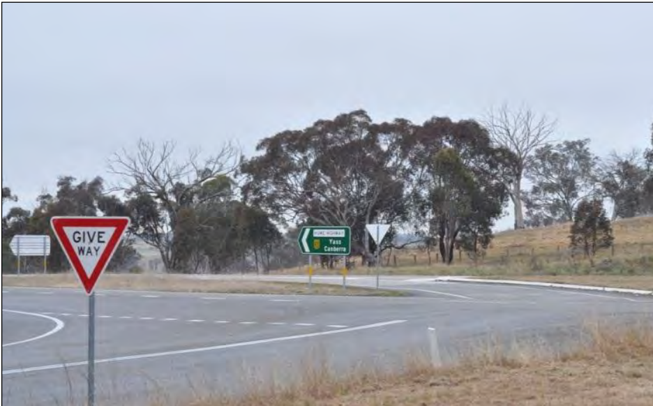
Figure 4-9 Exit from Hume Highway to Lachlan Valley Way
