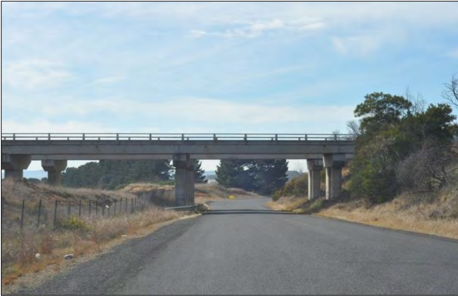
Figure 4-4 Hume Highway underpass on Faulder Avenue
