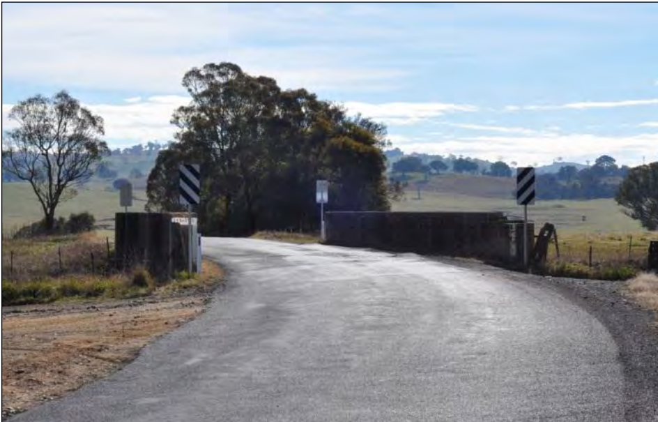
Figure 4-5 Railway overpass on Cooks Hill Road
