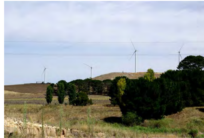
Photo 3 - View toward operational Capital wind farm turbines
