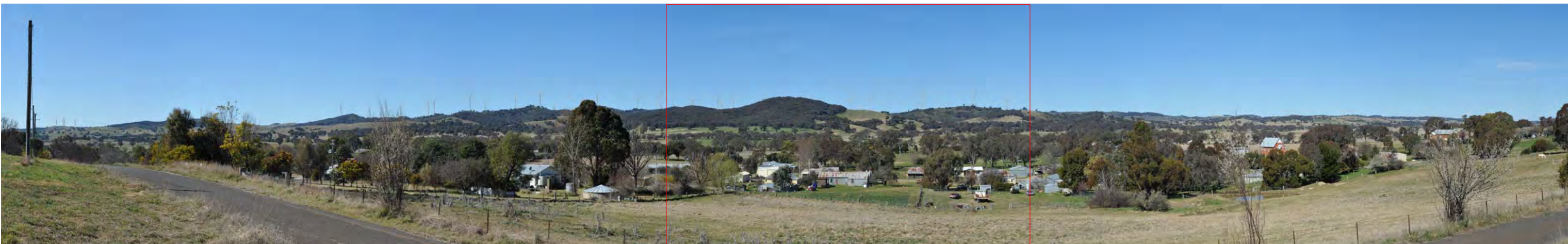
Public view location PM6 Kershaw Street, Rye Park- Proposed view through 120°. Approximate distance to closest visible wind turbine 3,900 m
