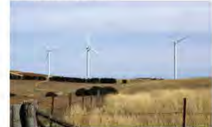
Photo 4 - View toward operational Capital wind turbines.
