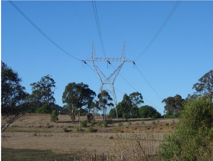
Example of 330kV transmission line tower structure
