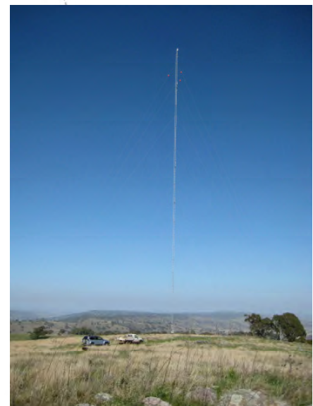
Figure 2 Mast onsite at Liverpool Range
