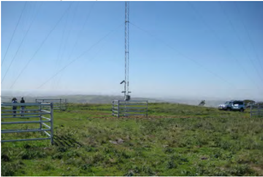
Epuron's wind monitoring at Liverpool Range
