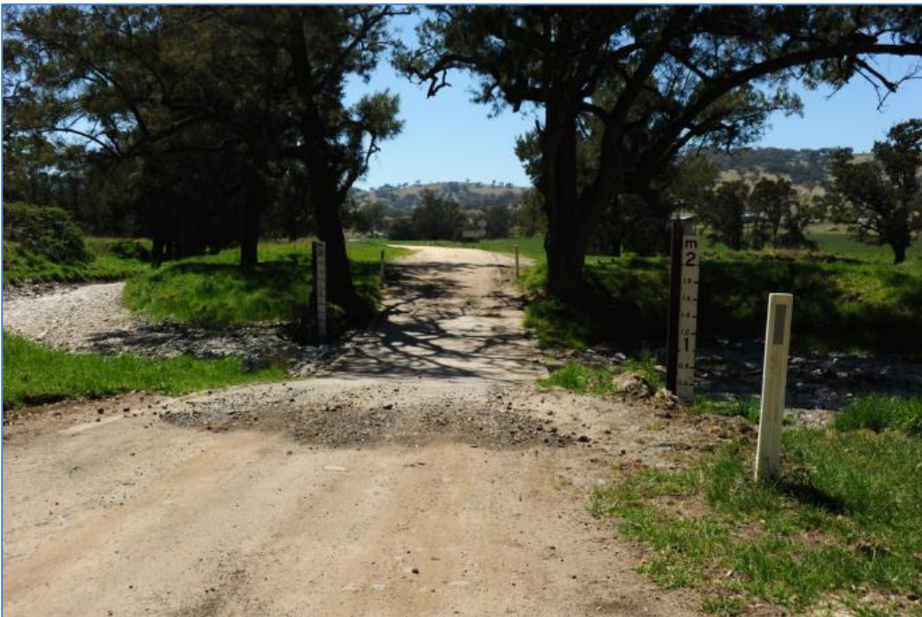
Figure 4-11 River crossing on Turee Road after Sherwood main gate
