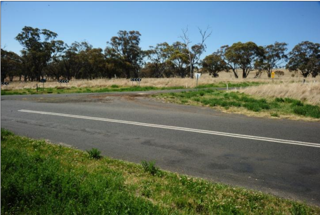
Figure 4-4 Intersection of Warrumbungles Way & Coolah Road
