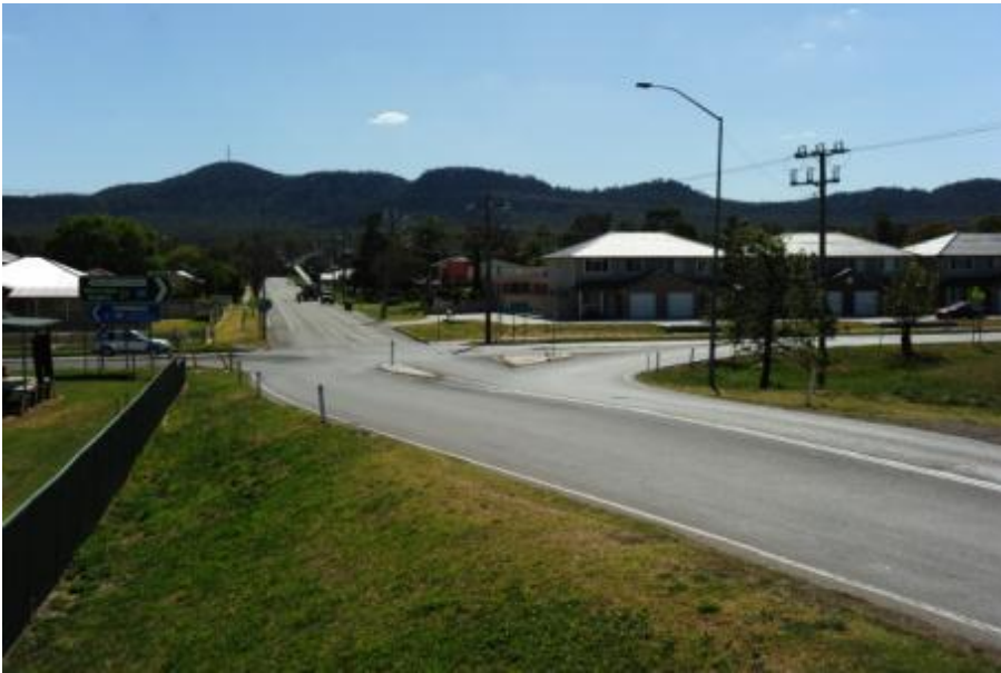
Figure 4-2 Right-hand bend on Golden Highway in Denham
