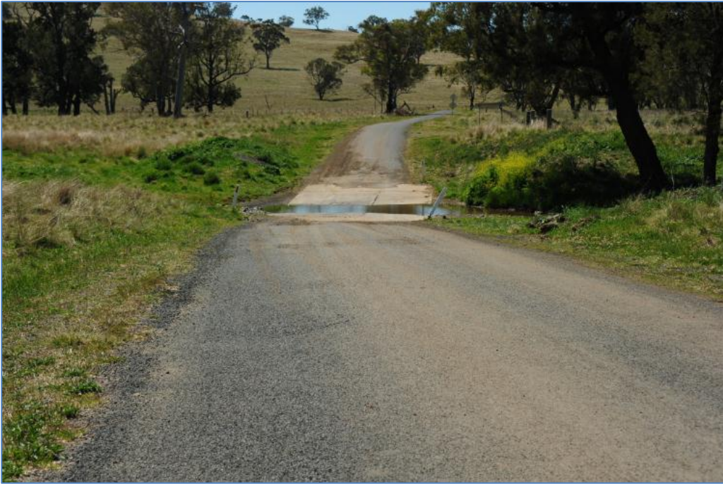
Figure 4-6 Creek crossing on Rotherwood Road
