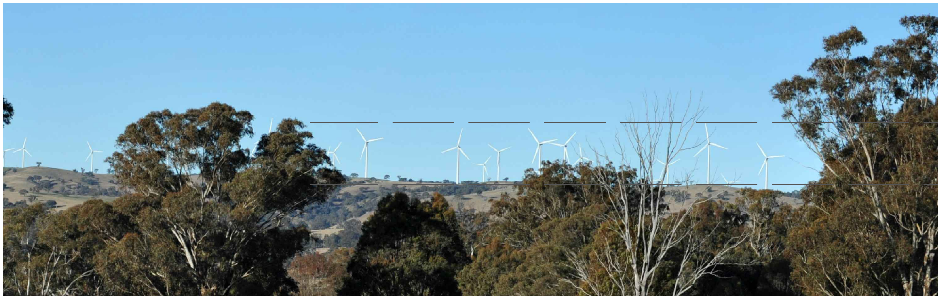
Existing view toward the operational Gunning wind farm from Gunning Road.
