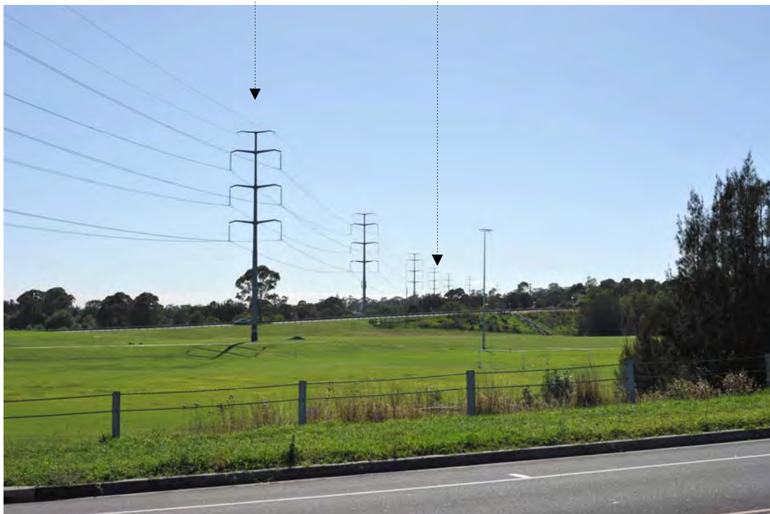
Plate 16 Existing 330 kV double circuit powerline
