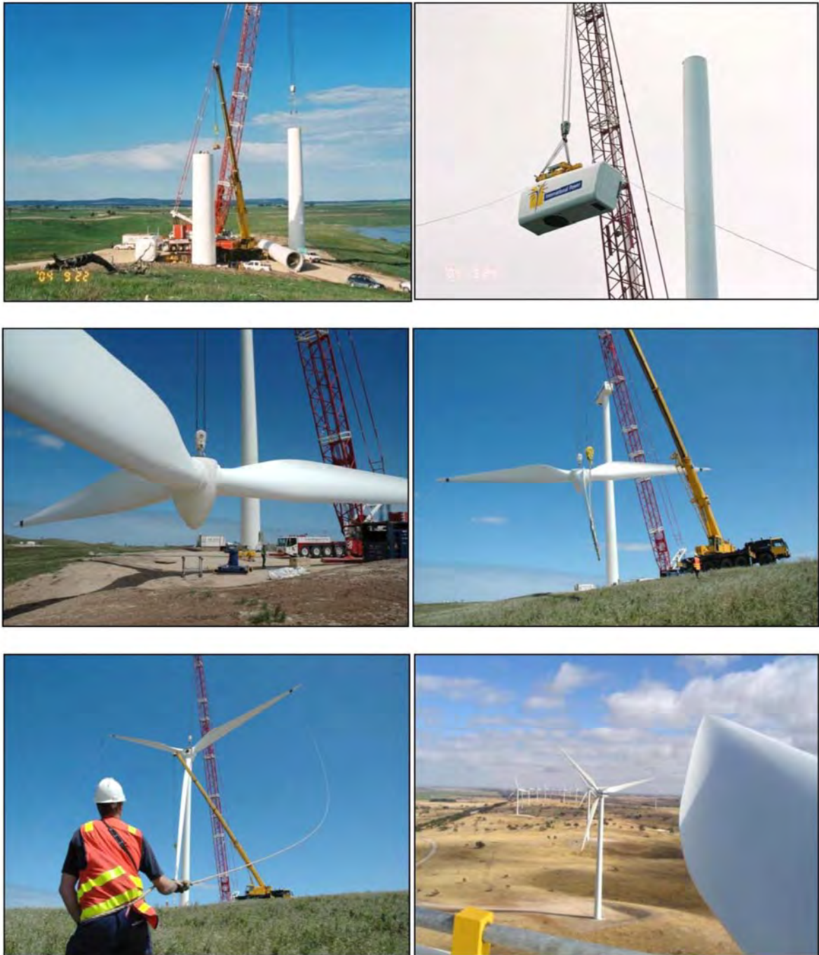
Plate 18 Illustrating typical activities during wind farm construction and installation.
