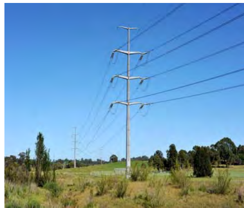
Plate 12 –Typical illustration of a 330 kV supporting structure
