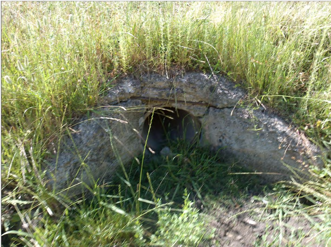
S140 – 375mm Pipe Culvert
