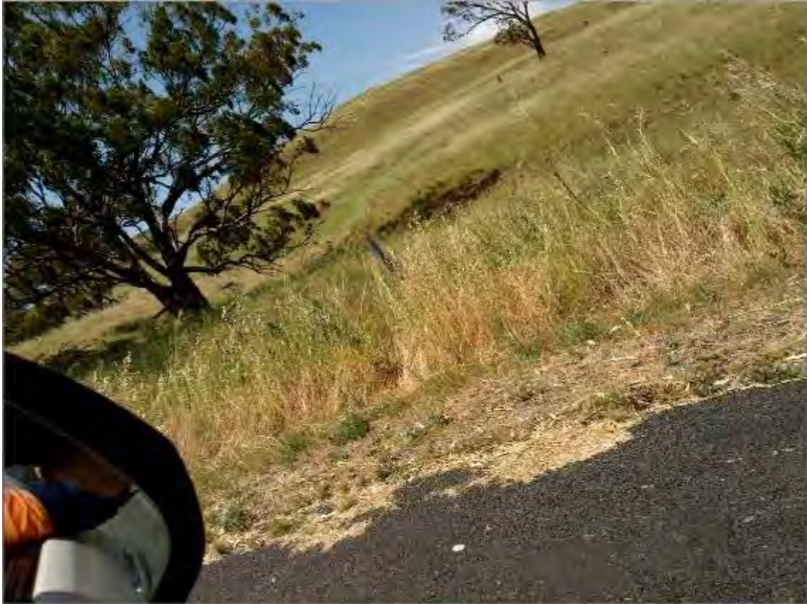
S181 – View towards Culvert
