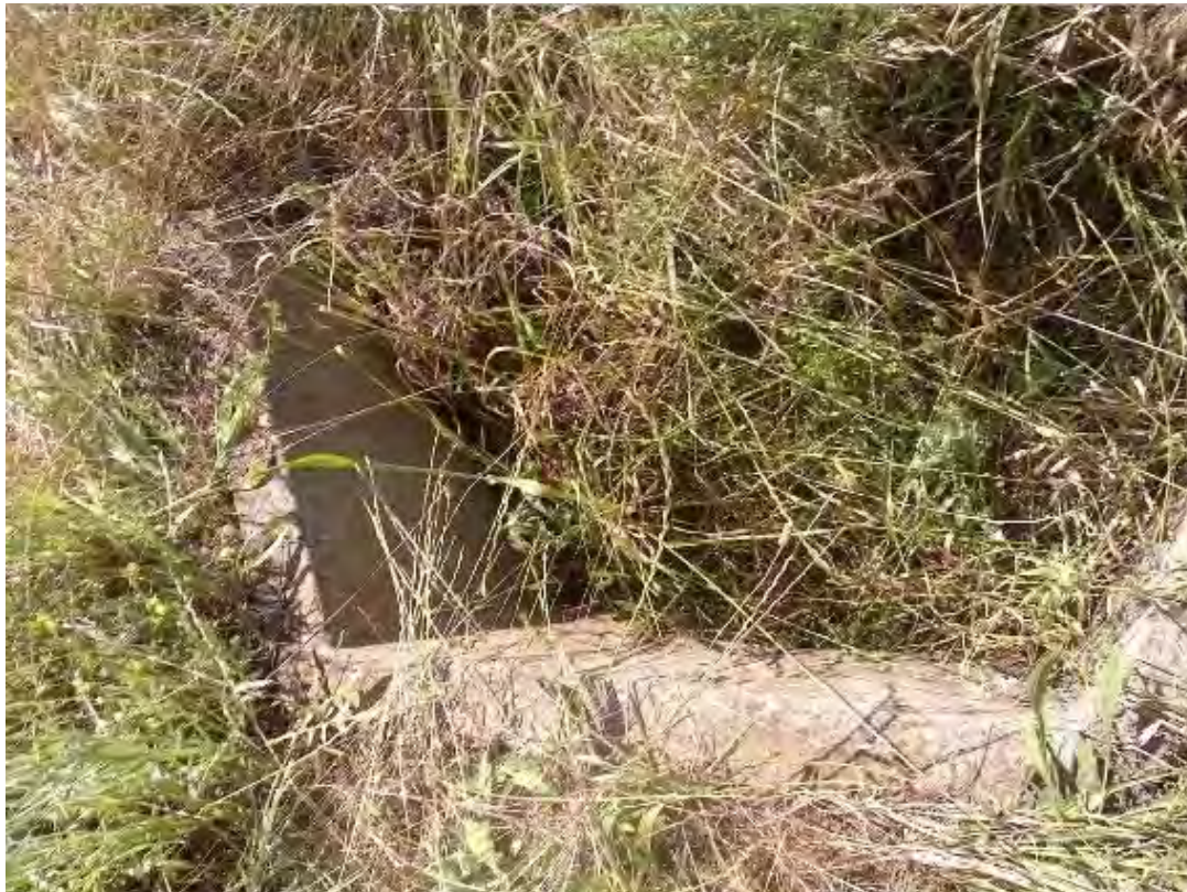
S174 – Top View of Culvert 450mm Pipe Culvert
