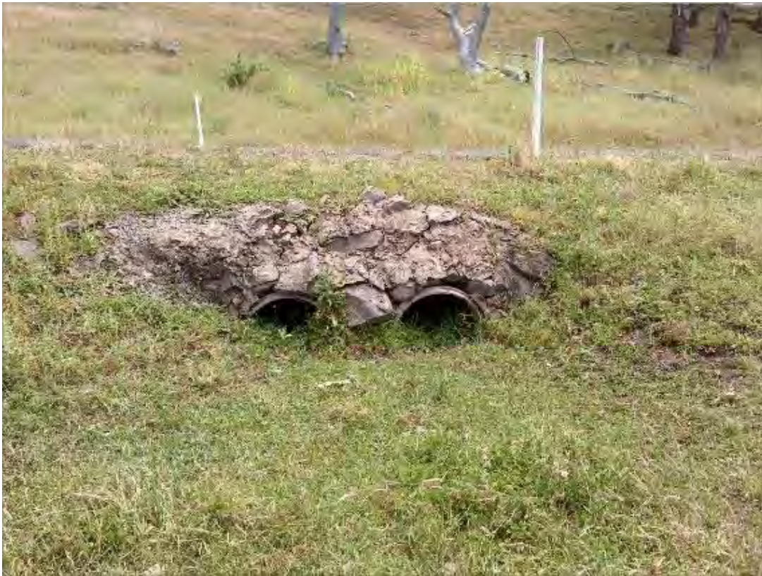
S196 – Dual -525mm Pipe Culvert
