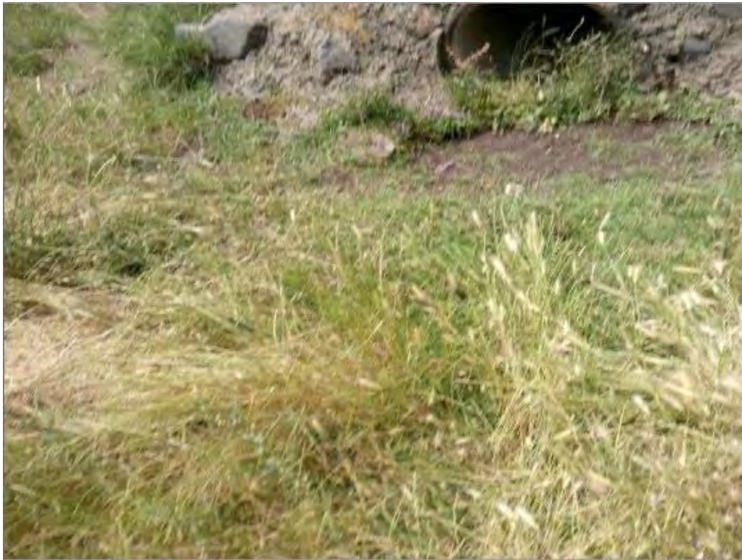
S193a - 675mm Pipe Culvert
