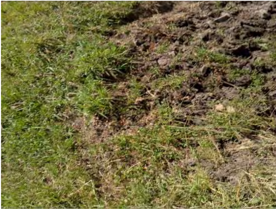
S155 – View over 450mm Pipe Culvert
