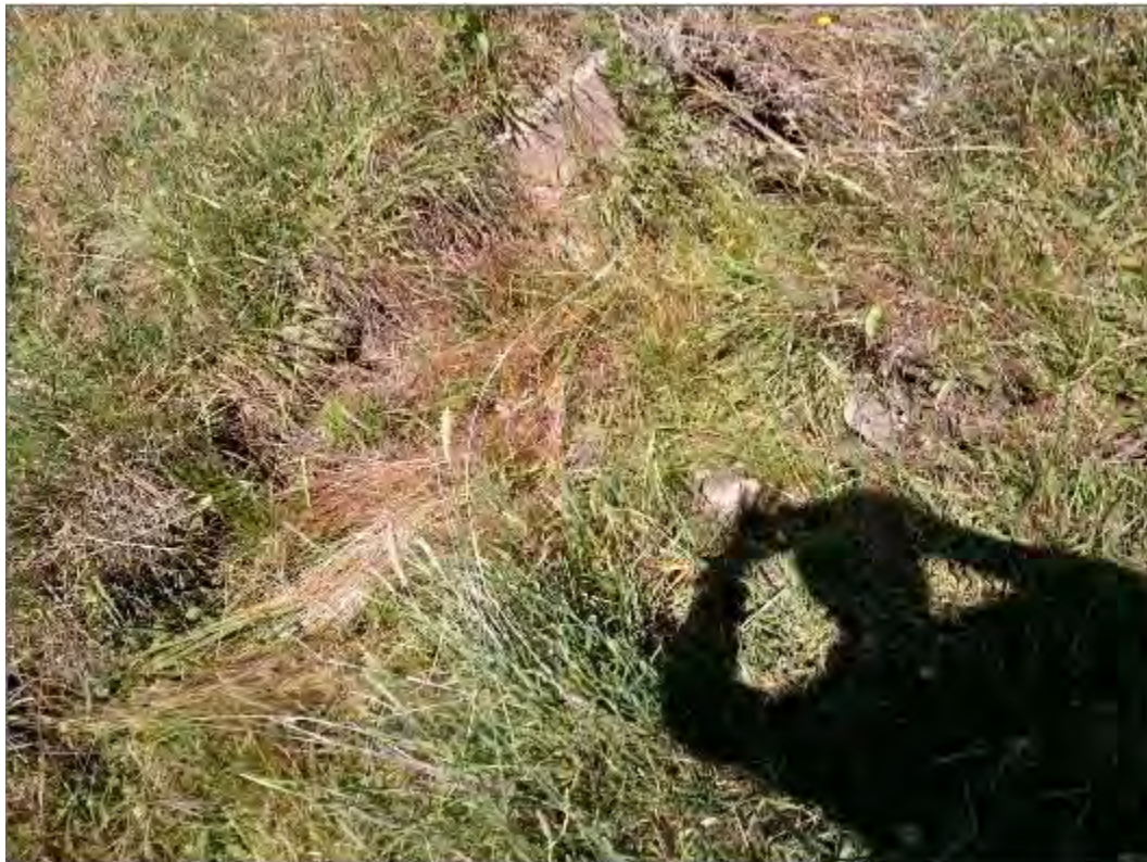
S145 - 600mm Pipe Culvert at top of Image
