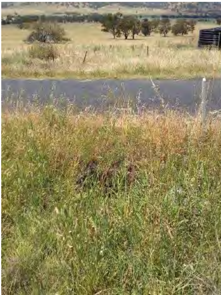
S193 – 450mm pipe culvert
