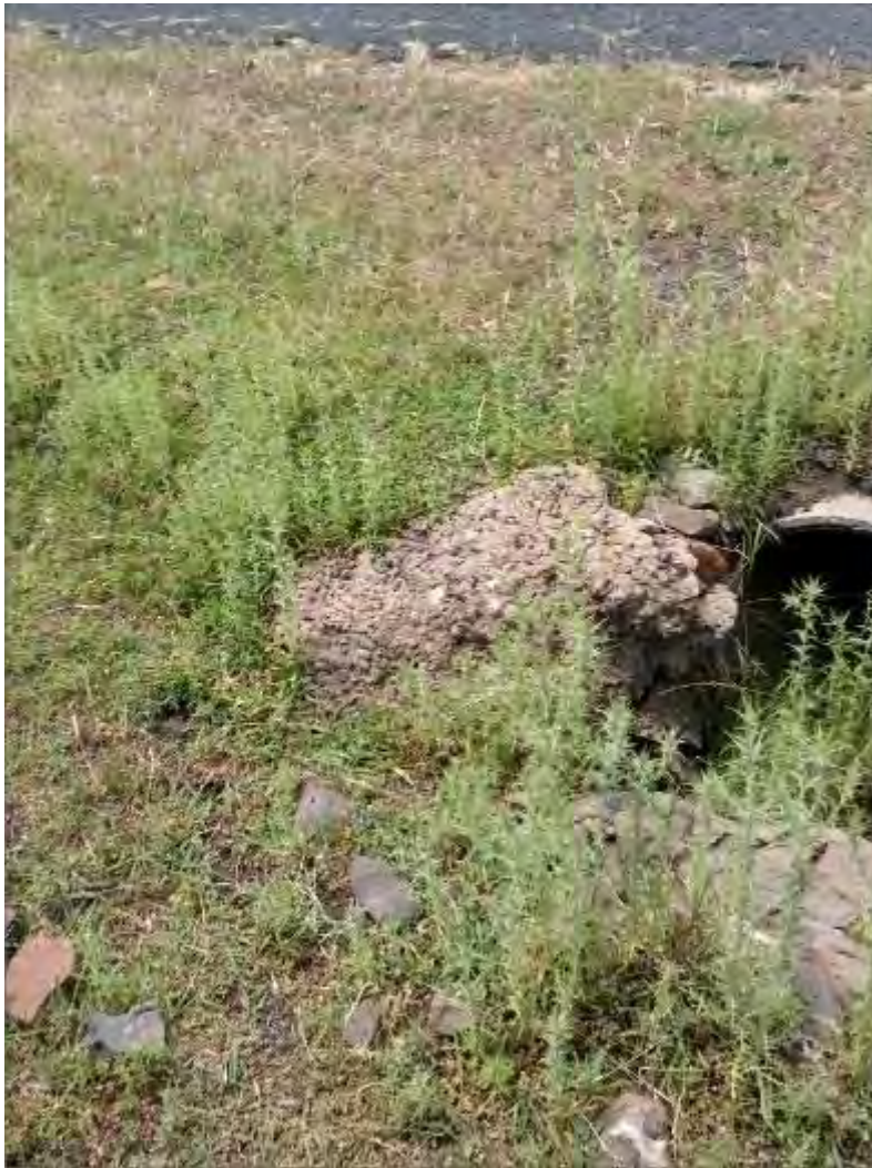
S195 – 600mm Pipe Culvert
