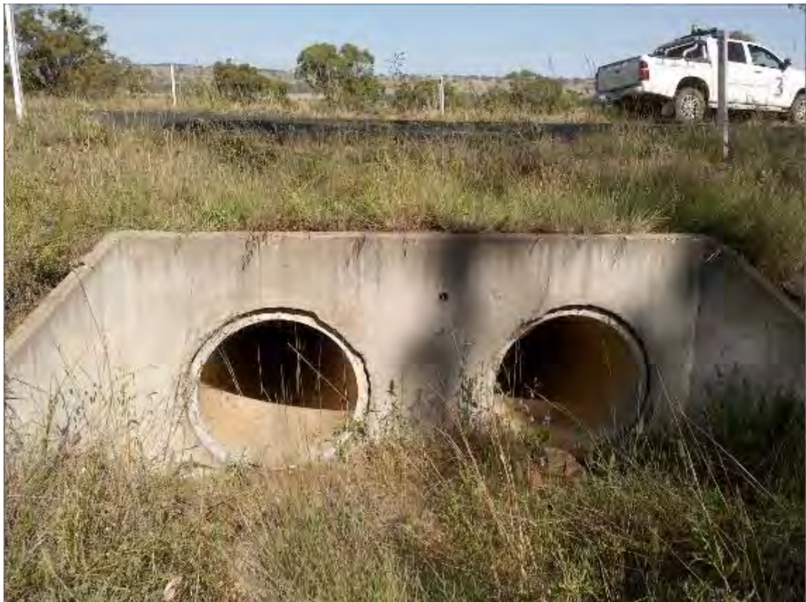
S171 – Dual 750mm Pipe Culvert
