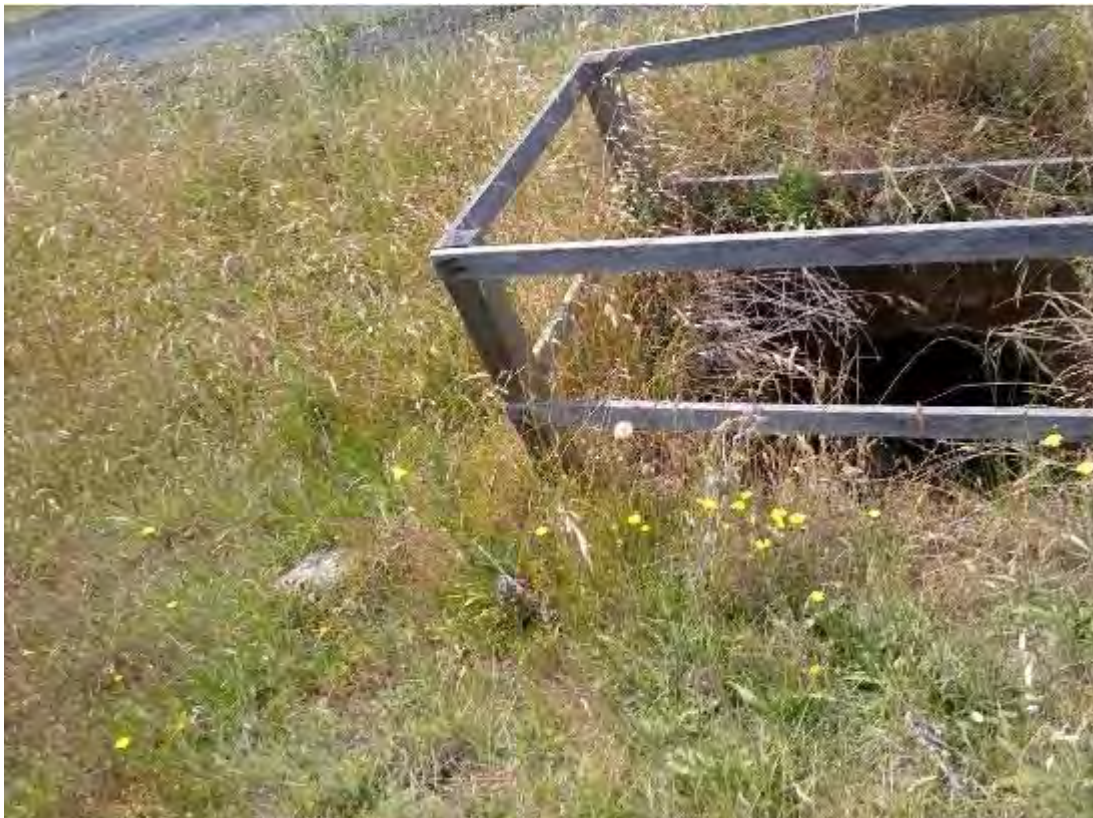
S184 – 750mm Pipe Culvert
