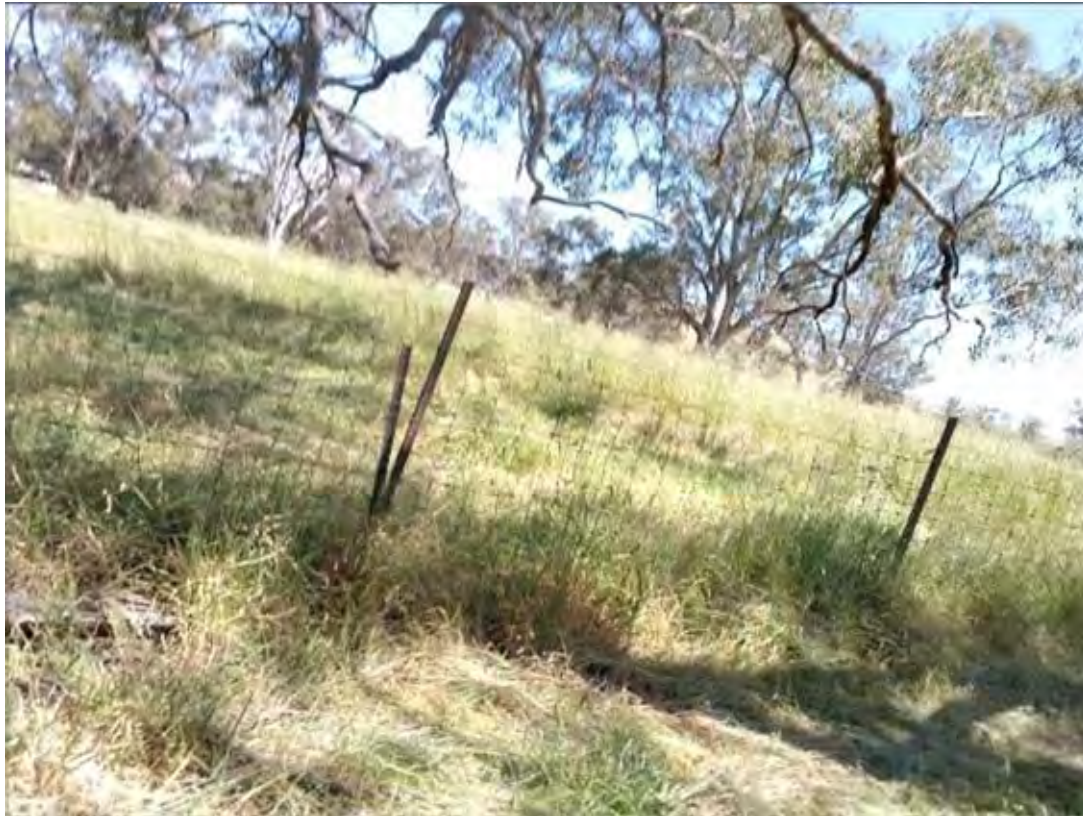
S145a – View towards 525mm Pipe Culvert
