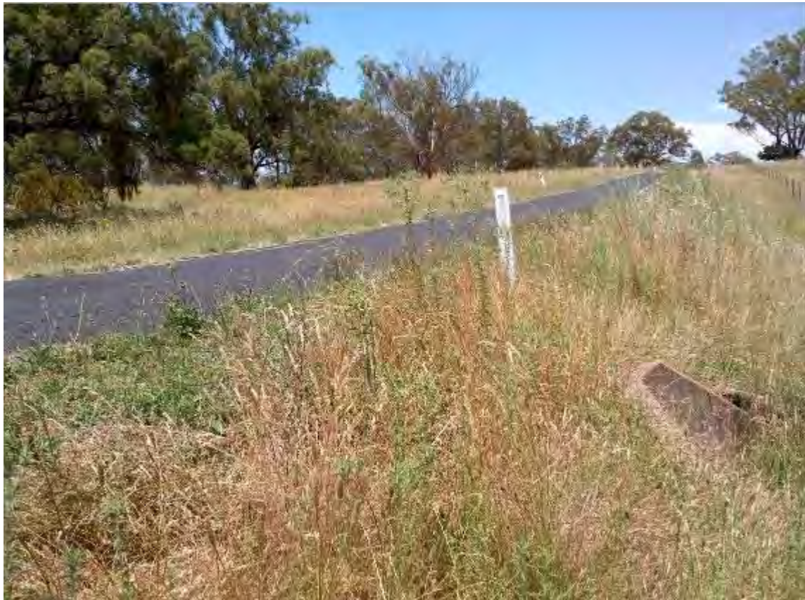
S187 - 750mm Pipe Culvert
