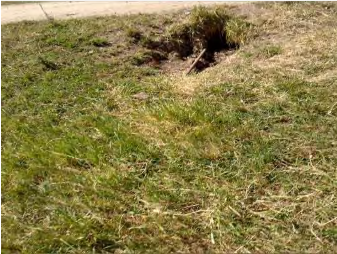
S153 – 600mm Pipe Culvert
