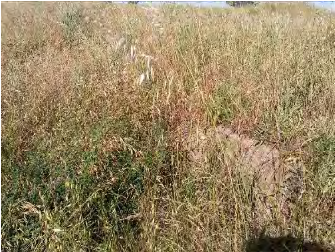
S174 – 450mm Pipe Culvert
