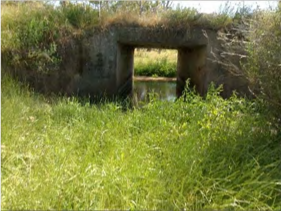
S161 - 1500mm Square Reinforced Concrete Box Culvert
