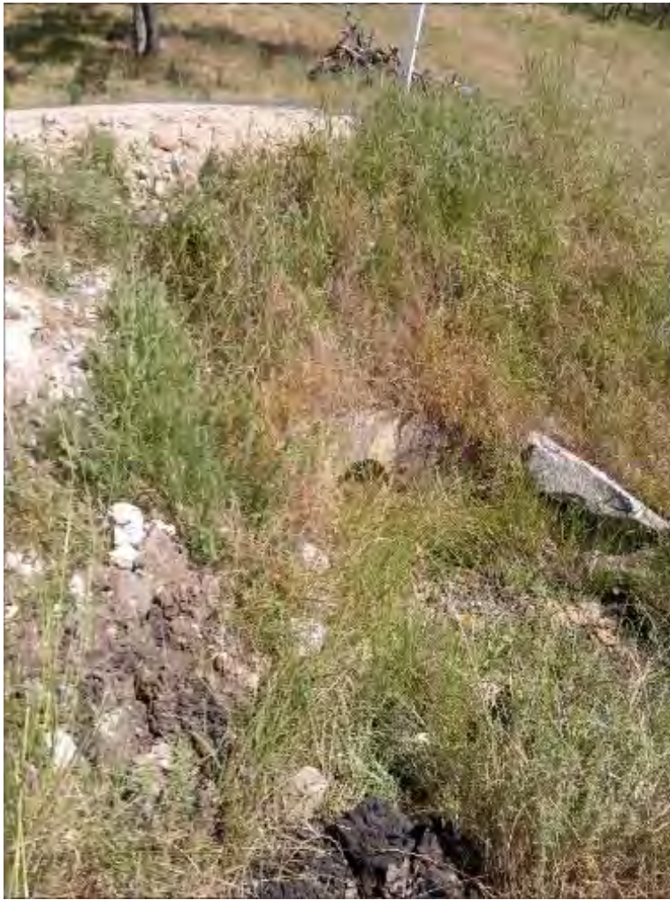
S142 - 450mm Pipe Culvert
