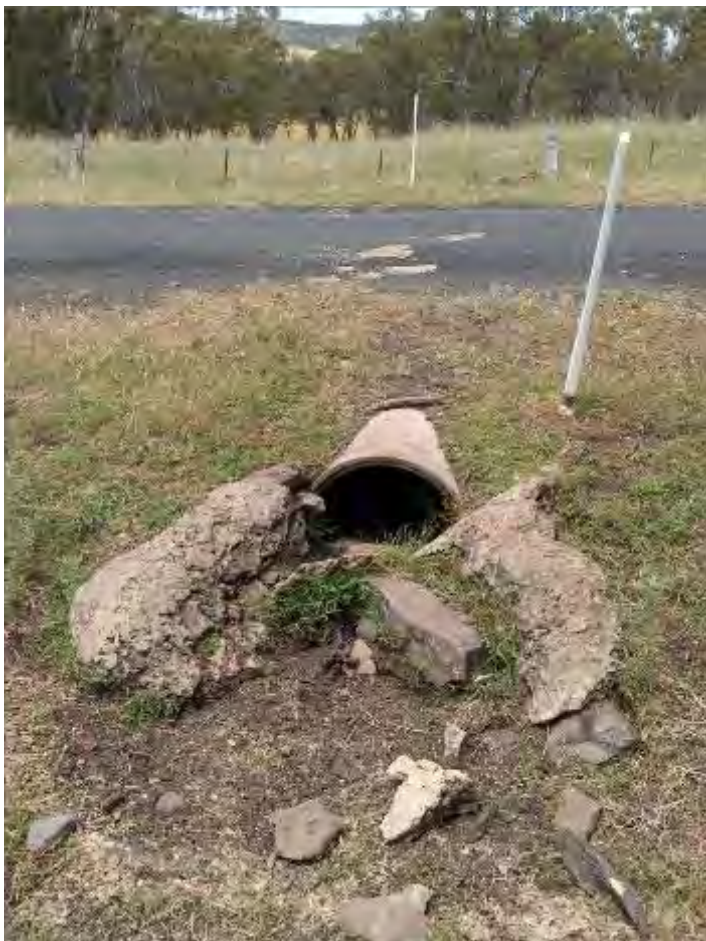
S194 – 600mm Pipe Culvert
