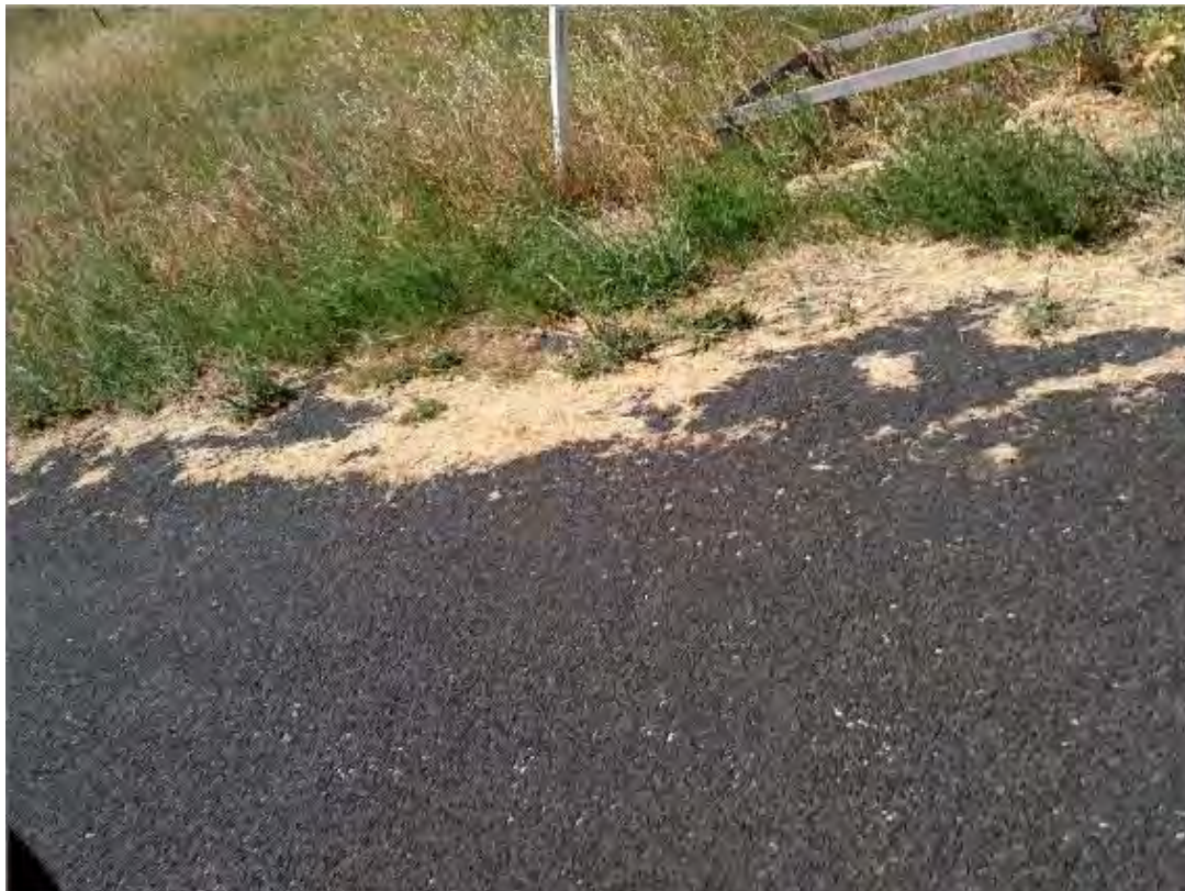
S180 – View of Culvert
