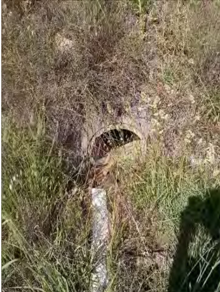
S168 - 450mm Pipe Culvert
