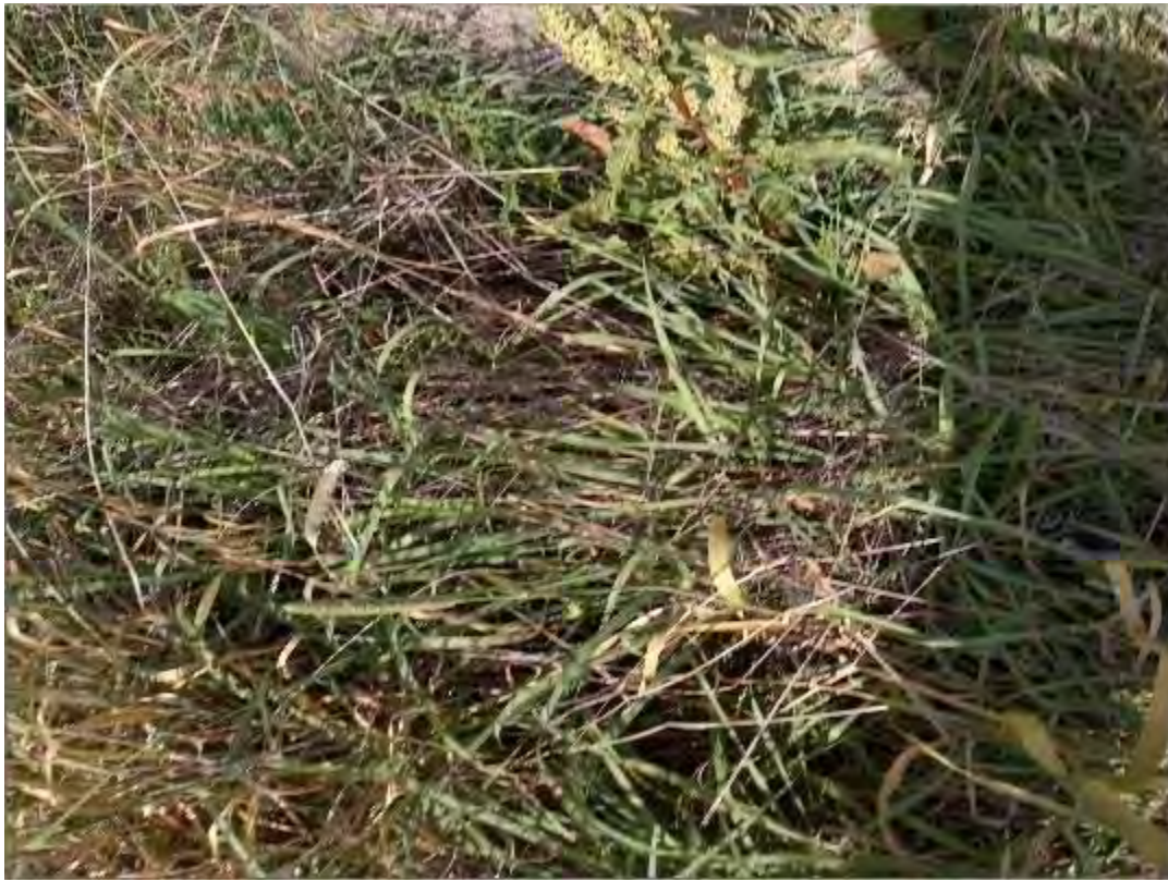
S087 – View of Hidden Culvert
