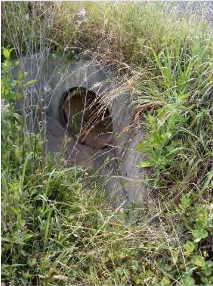
S083 - 450mm Pipe Culvert
