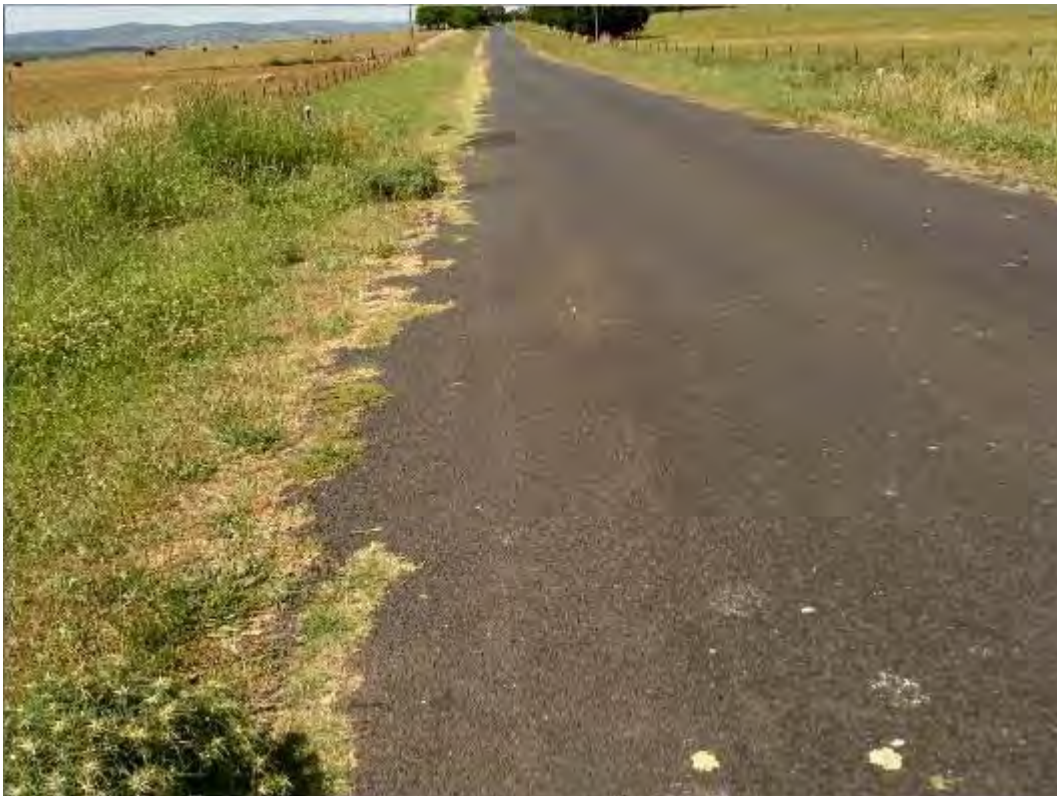
S014 – View to North
