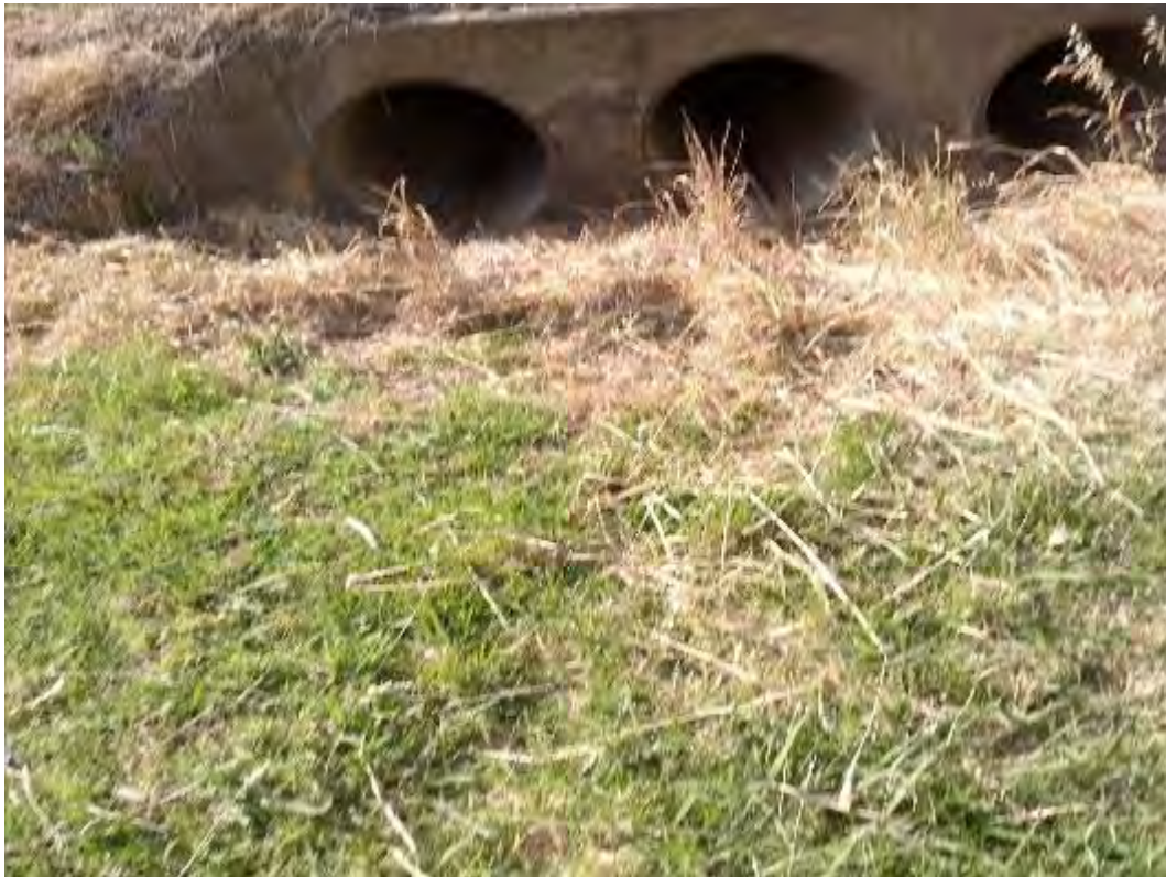
S077 – 3-900mm Pipe Culvert
