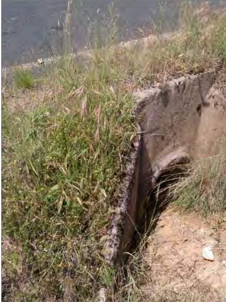
S107 – View to North perpendicular to Culvert
