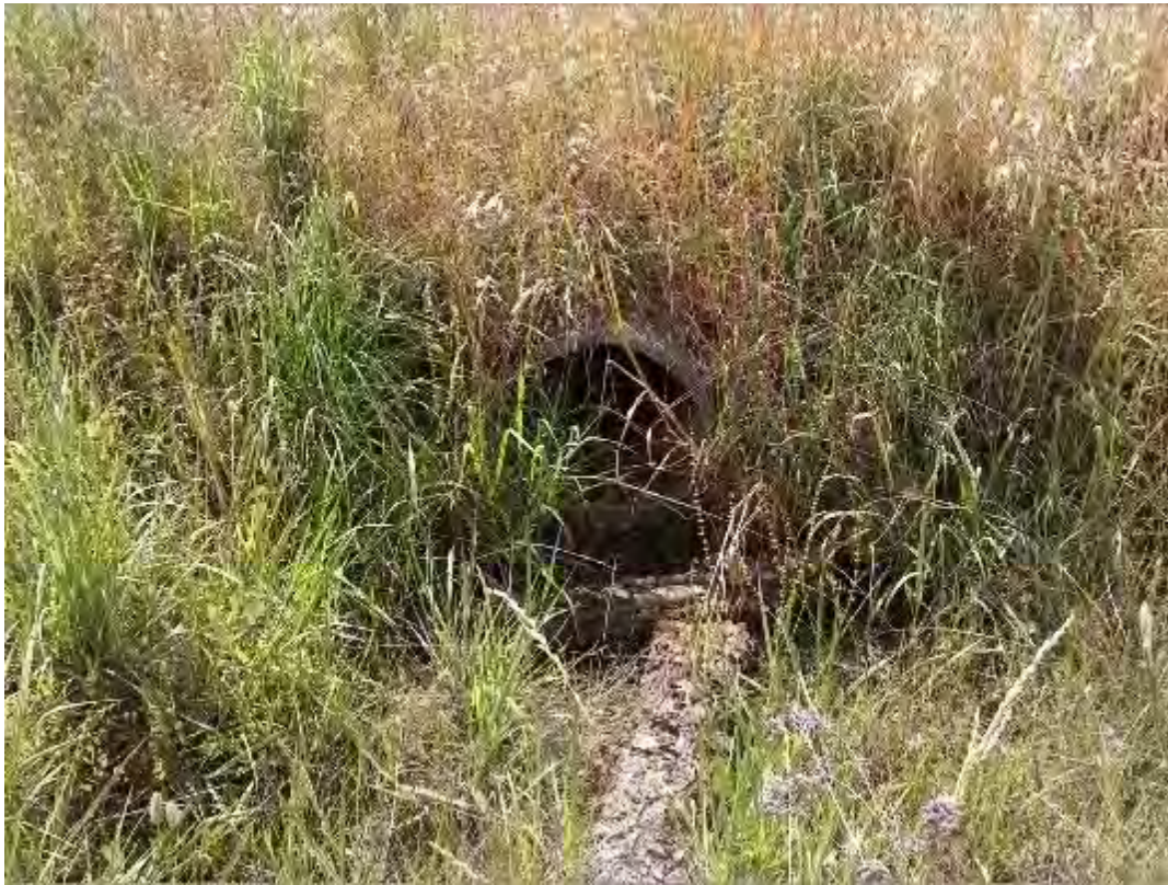
S103 – 600m Pipe Culvert
