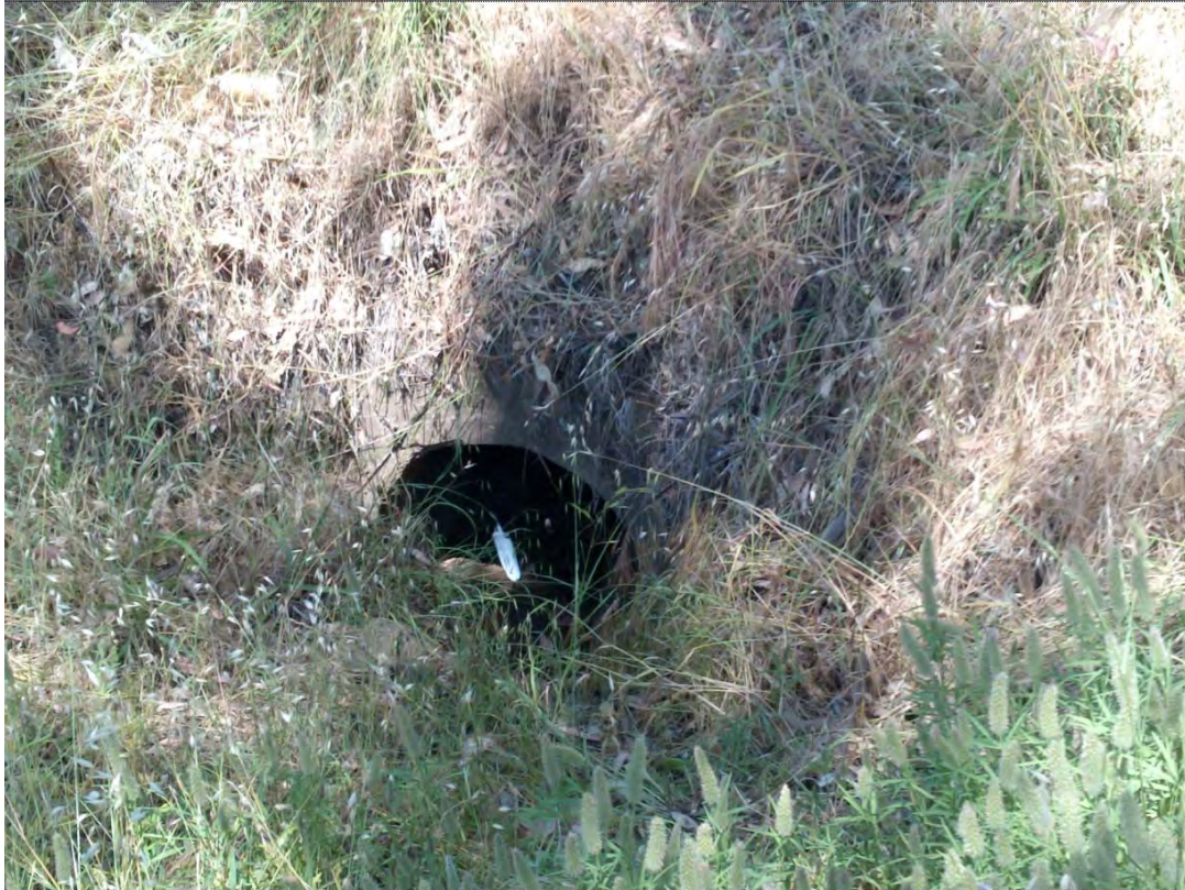
S120 - 750mm Pipe Culvert
