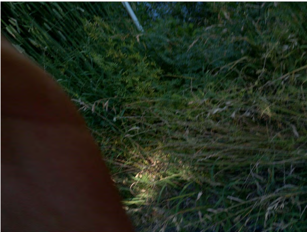
S126 – Hidden Culvert
