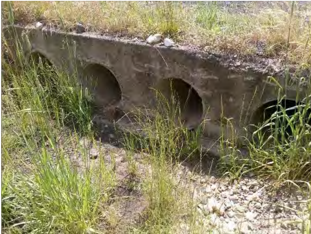
S099 - 4-450mm Pipe Culvert
