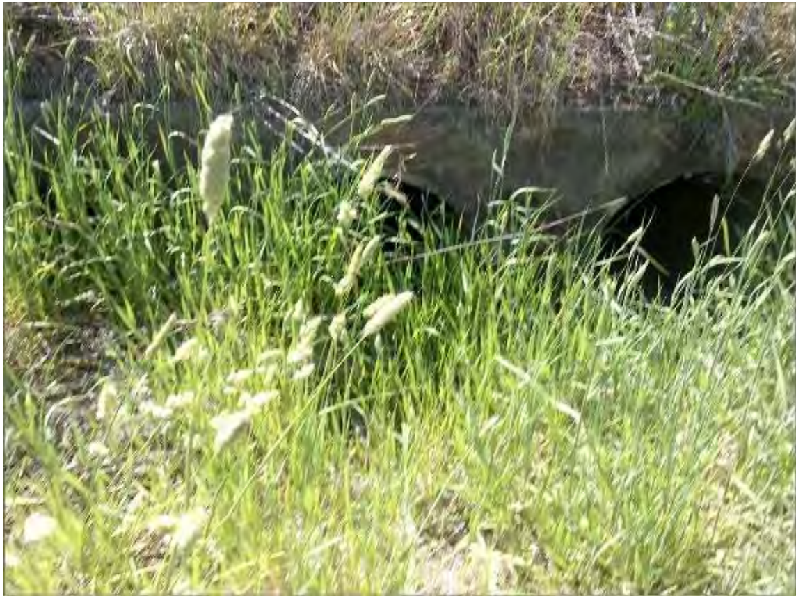
S116 - 3-750mm Pipe Culvert
