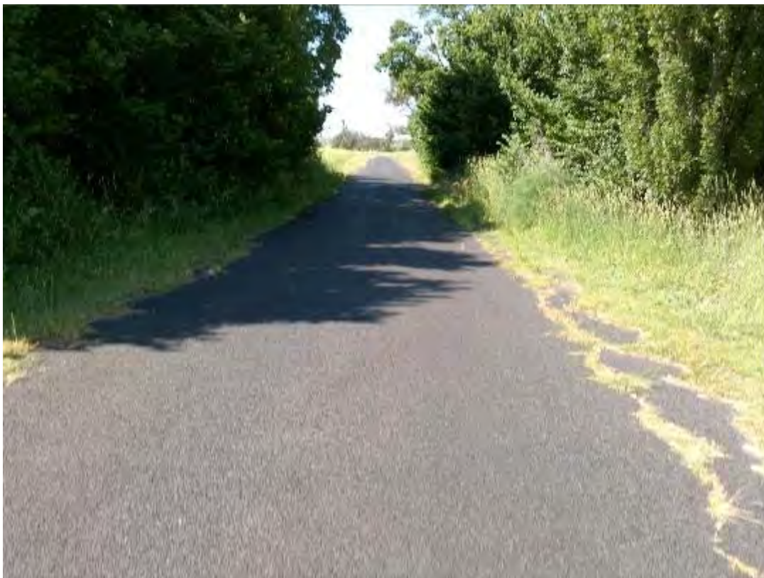
S126 – View to North
