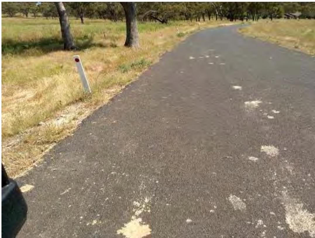
S135 – View to North
