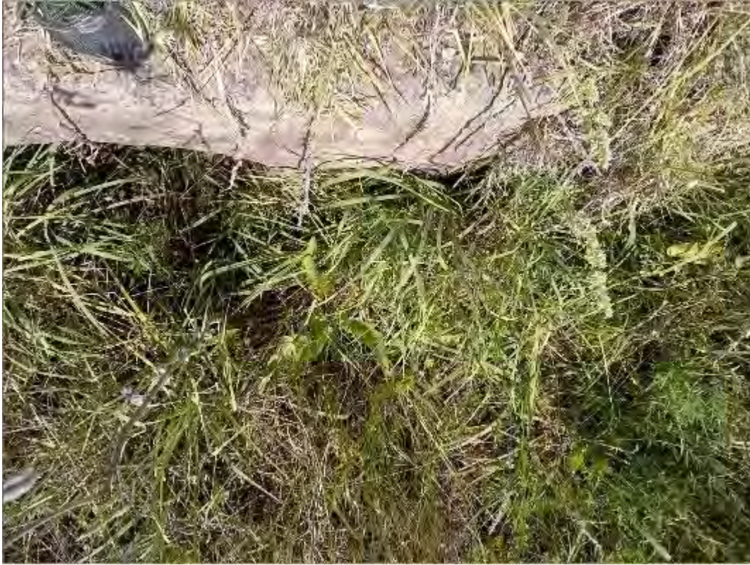
S088 - Dual 600mm Pipe Culvert
