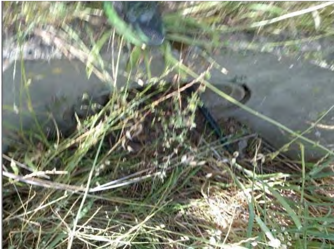
S081 - 600mm Pipe Culvert
