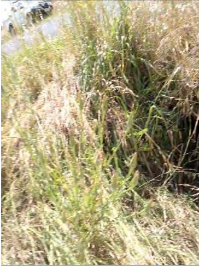
S104 – 525mm Pipe Culvert
