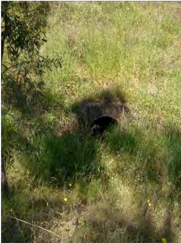
S123 – 1050mm Pipe Culvert
