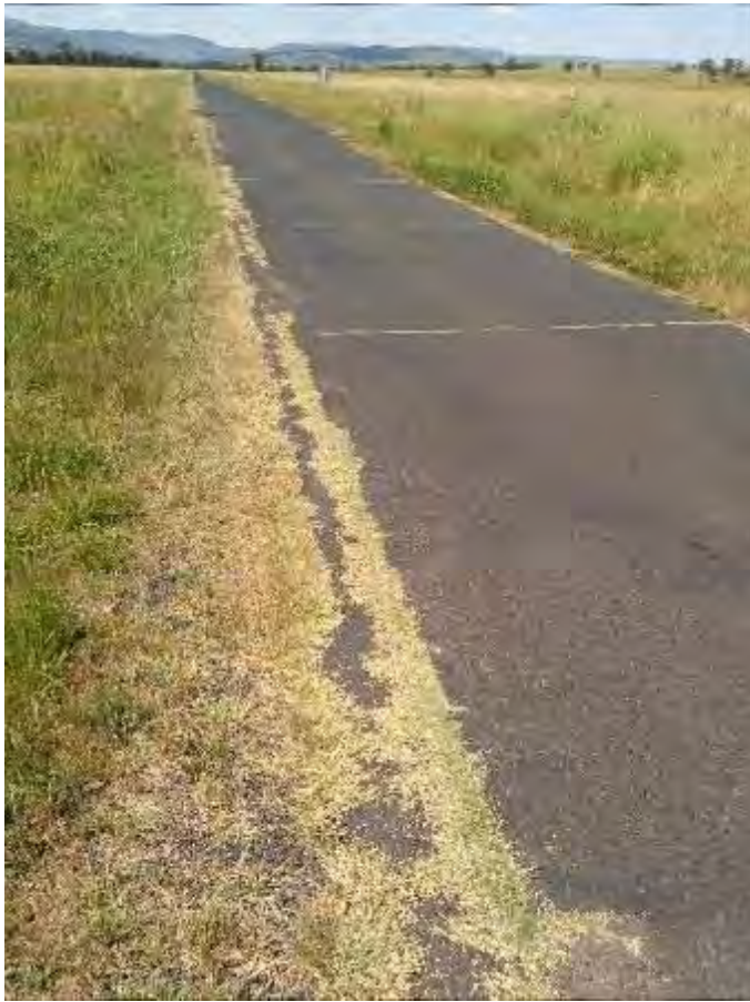
S102 – View to North
