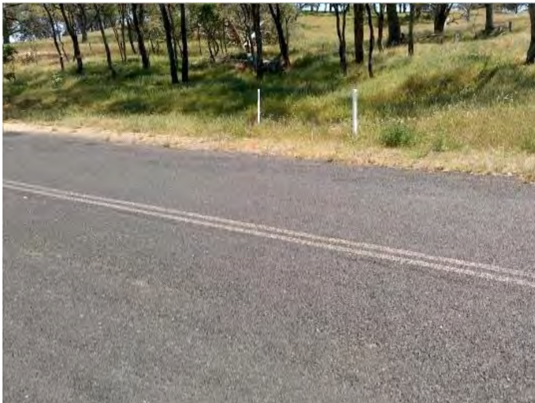
S122 – View to North
