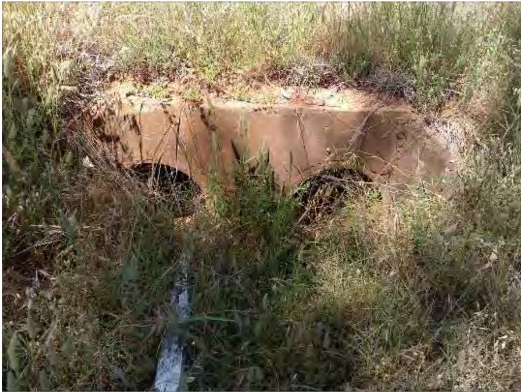
S122 – Dual 450mm Pipe Culvert
