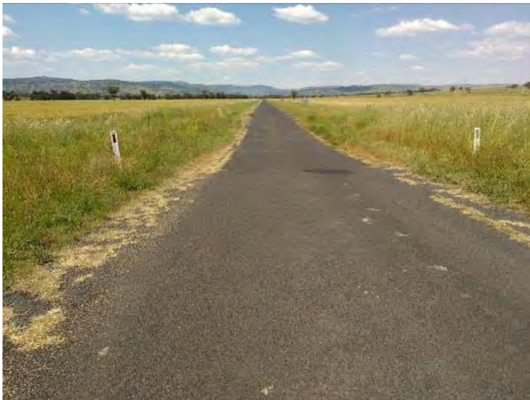
S102 – View to North
