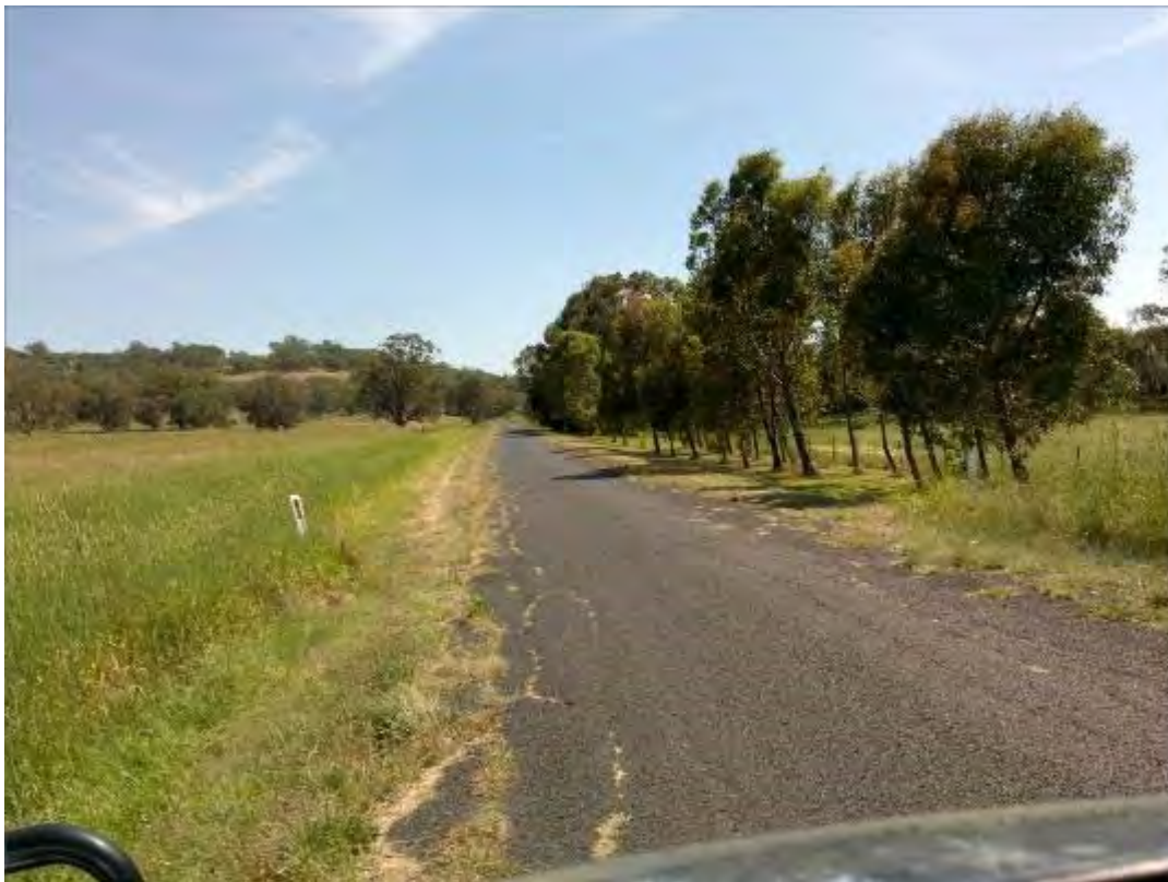
S133 – View to North
