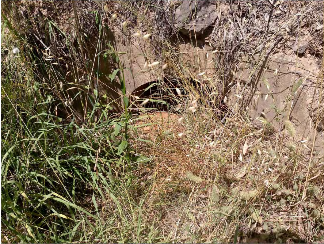
S121 - 600mm Pipe Culvert
