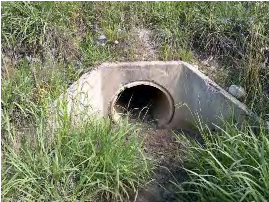
S082 – 600mm Pipe Culvert
