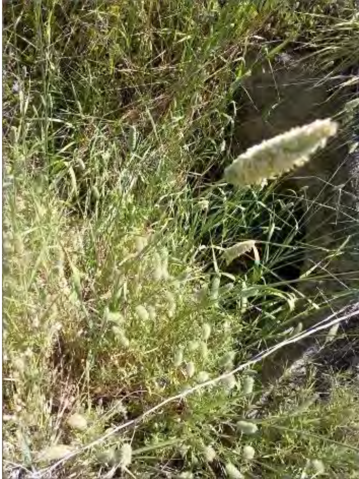
S114 – 600mm Pipe Culvert
