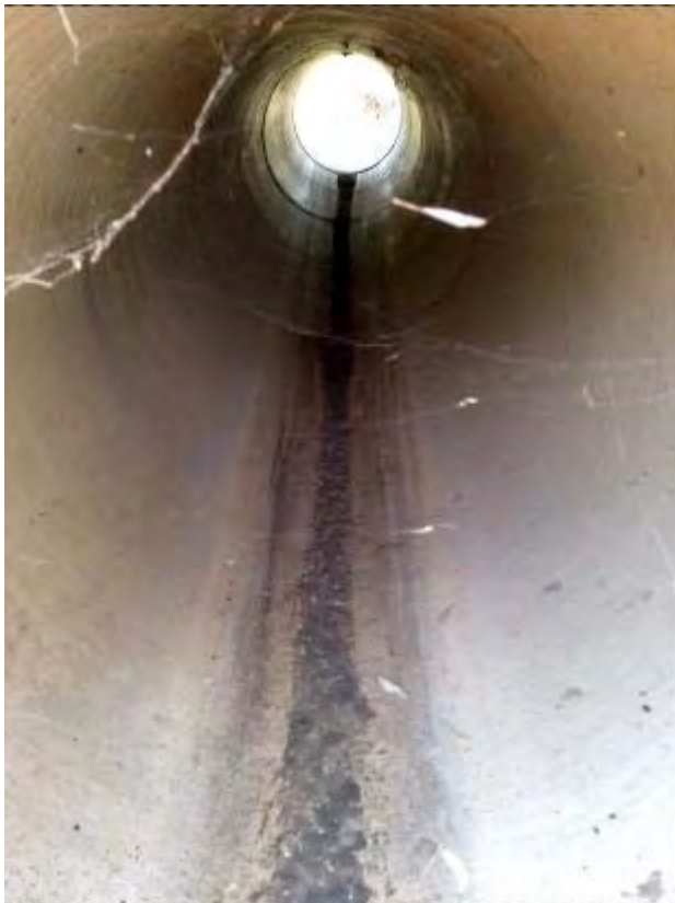
S077 – Internal View
