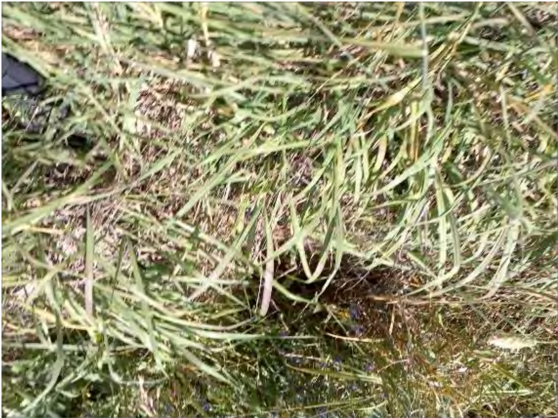
S127 – View looking to Pipe Culvert
