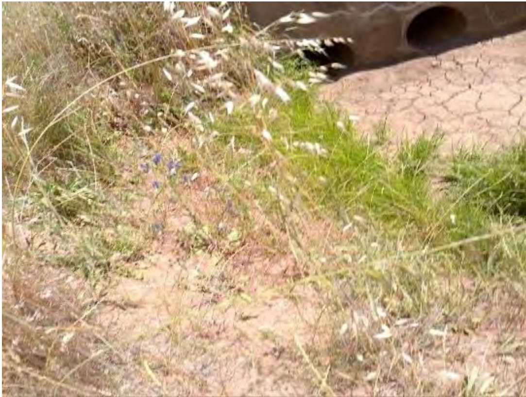
S106 - 3-450mm Pipe Culvert
