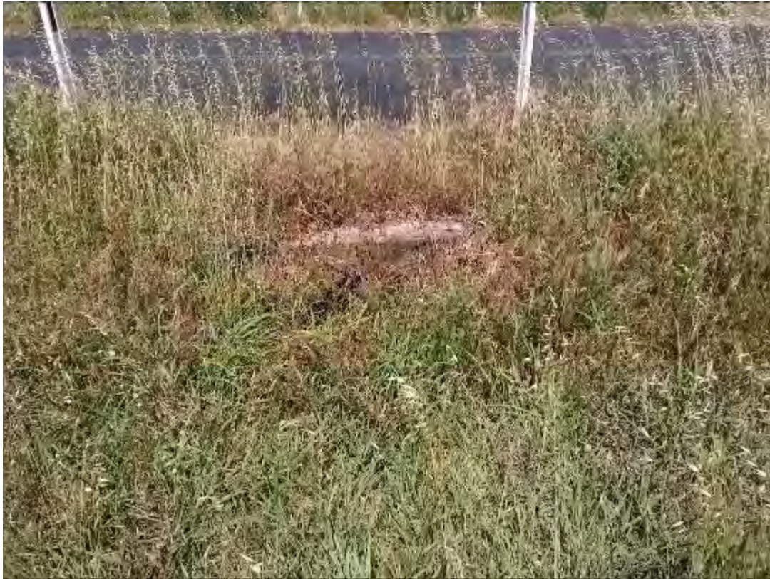
S119 - 600mm Pipe Culvert
