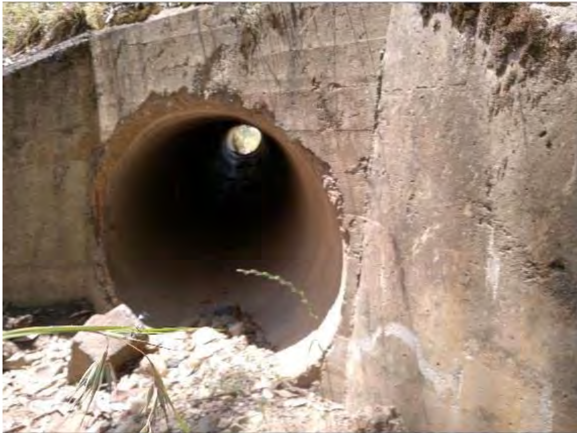
S108 – Skewed 1050mm Pipe Culvert showing Interior Condition
