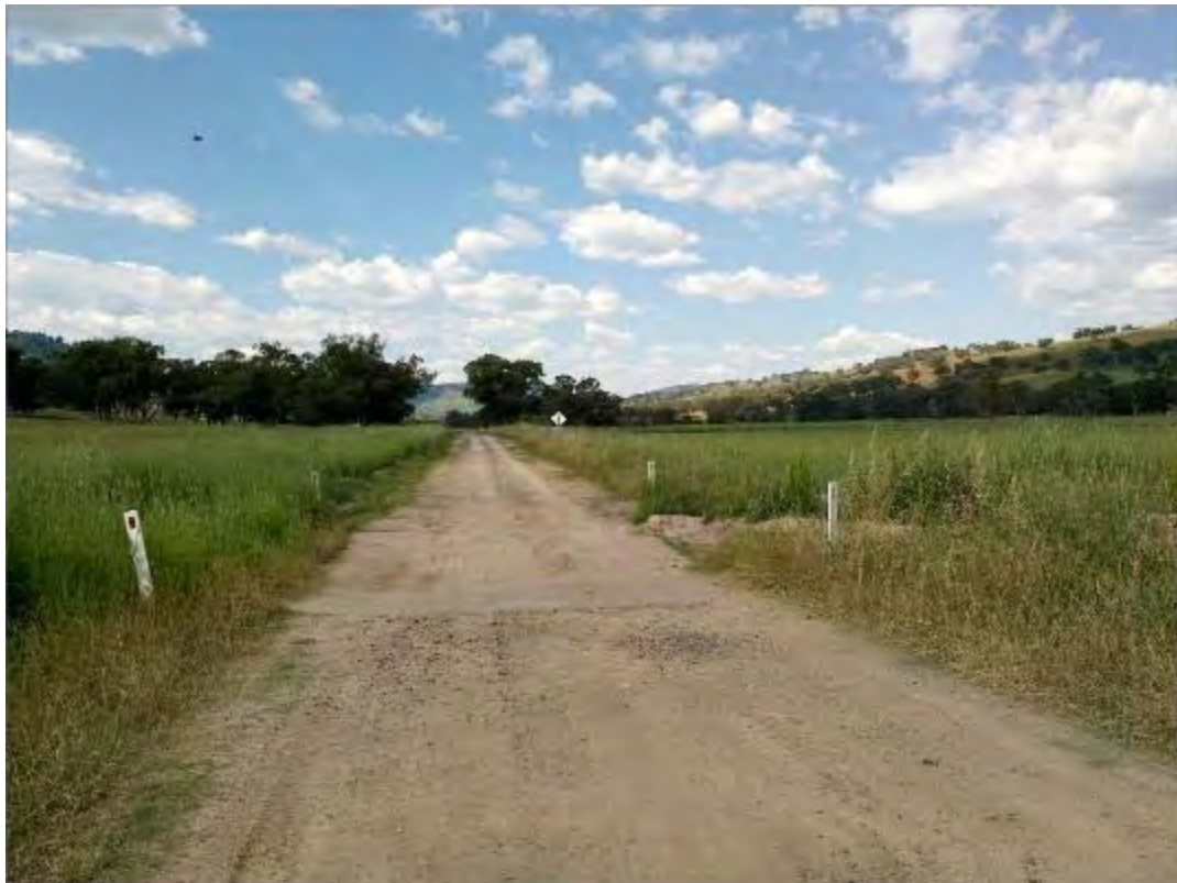
S095 – View to North
