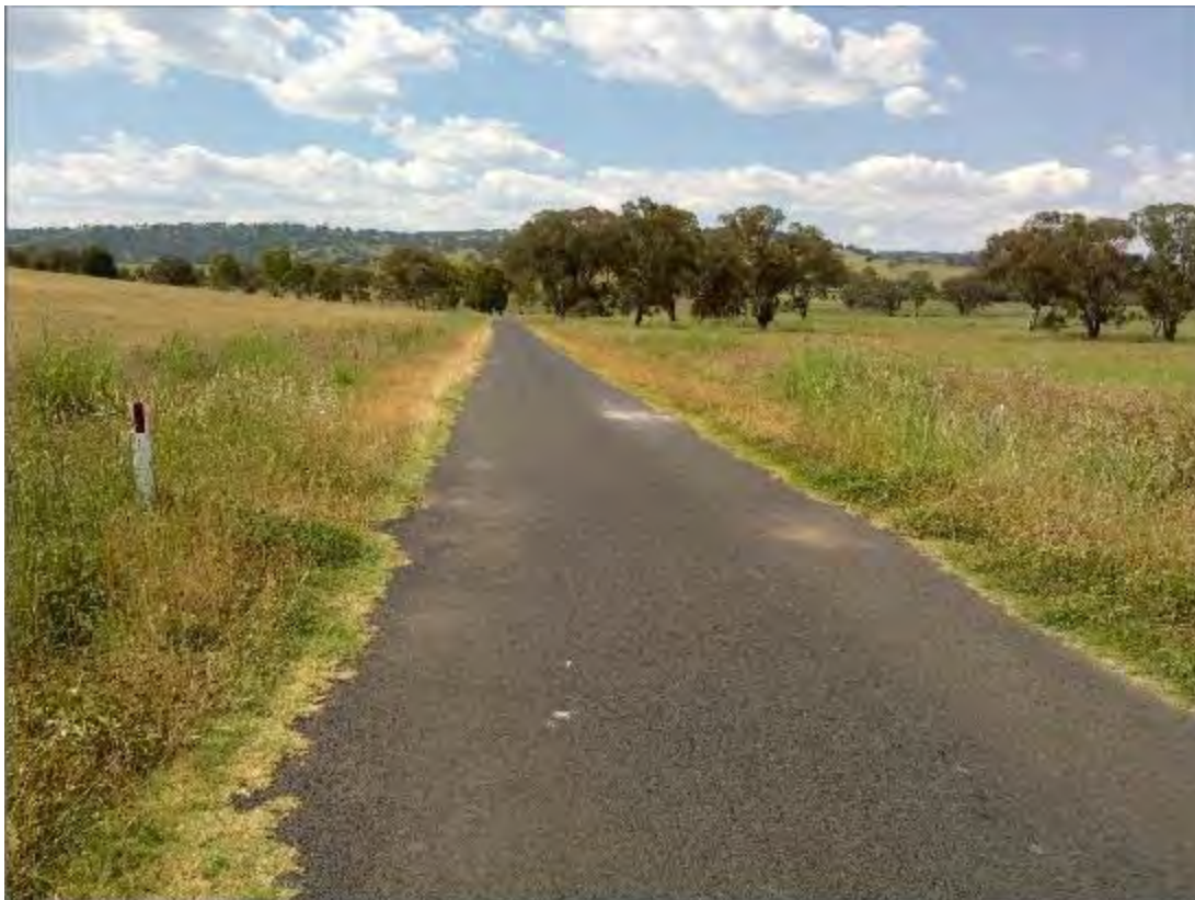
S088 – View to North
