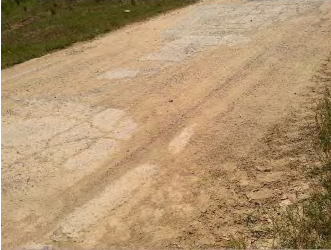
S233 – View to North
