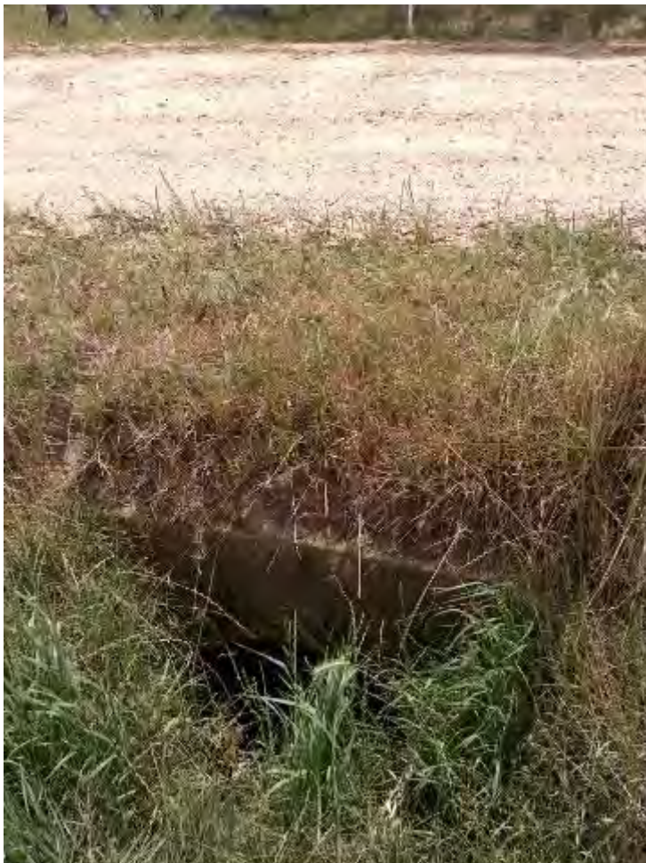
S235 - 600mm Pipe Culvert
