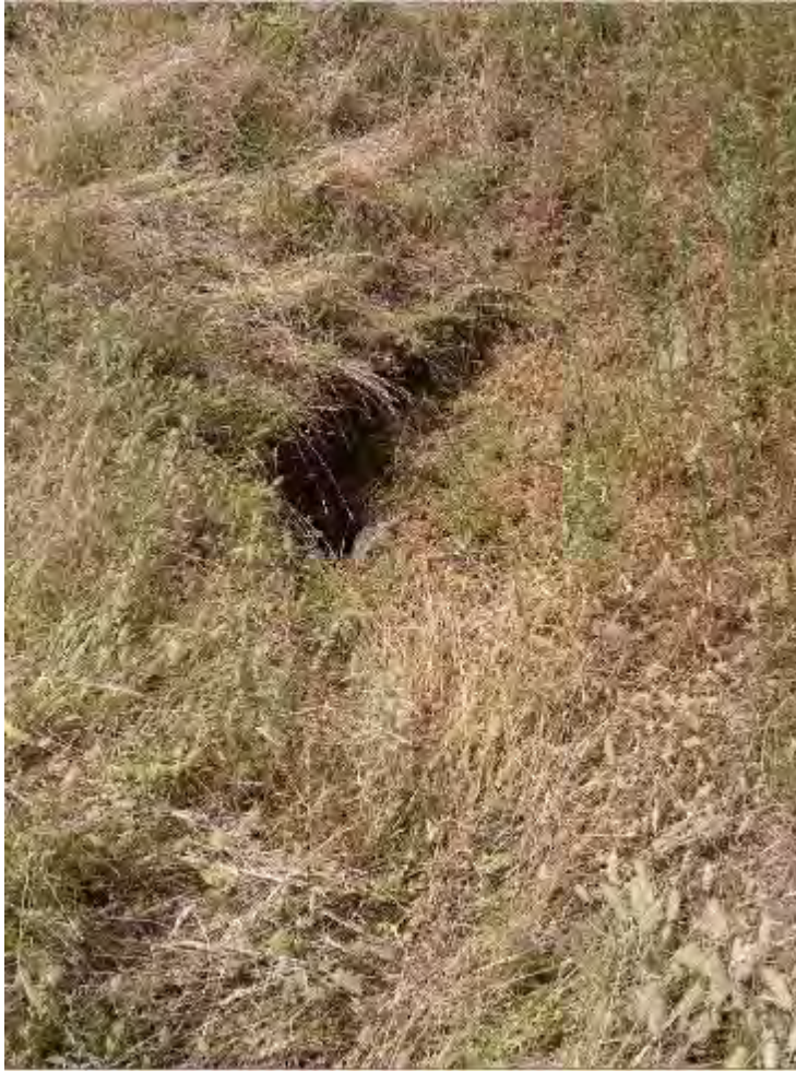
S221 - 450mm Pipe Culvert
