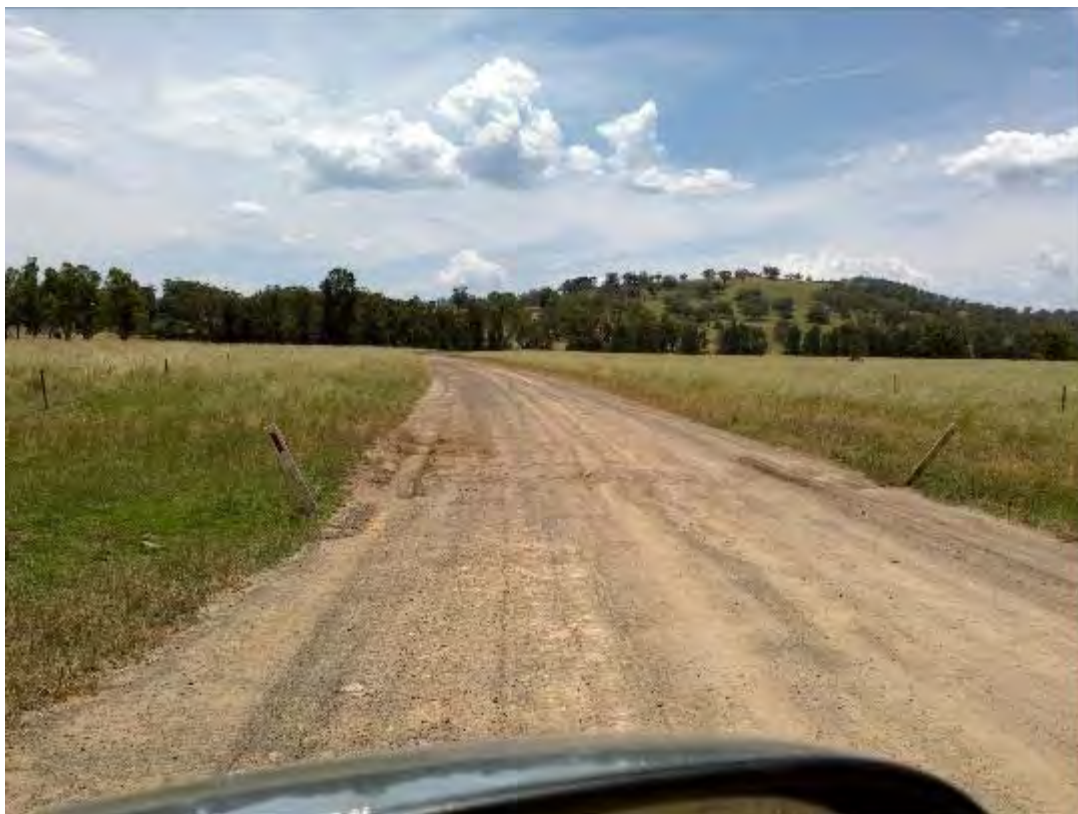
S214 – View to North
