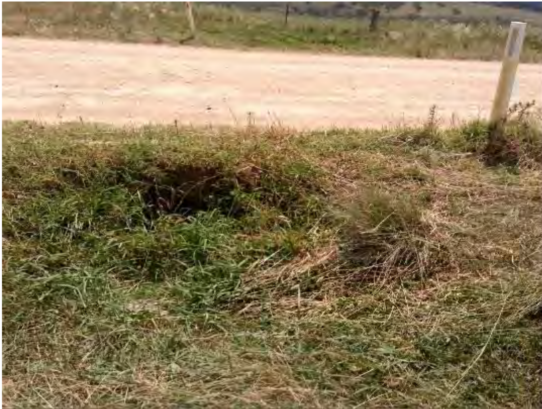
S247 – 450mm Pipe Culvert
