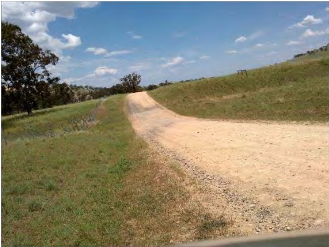
S232 – View to North and towards Location
