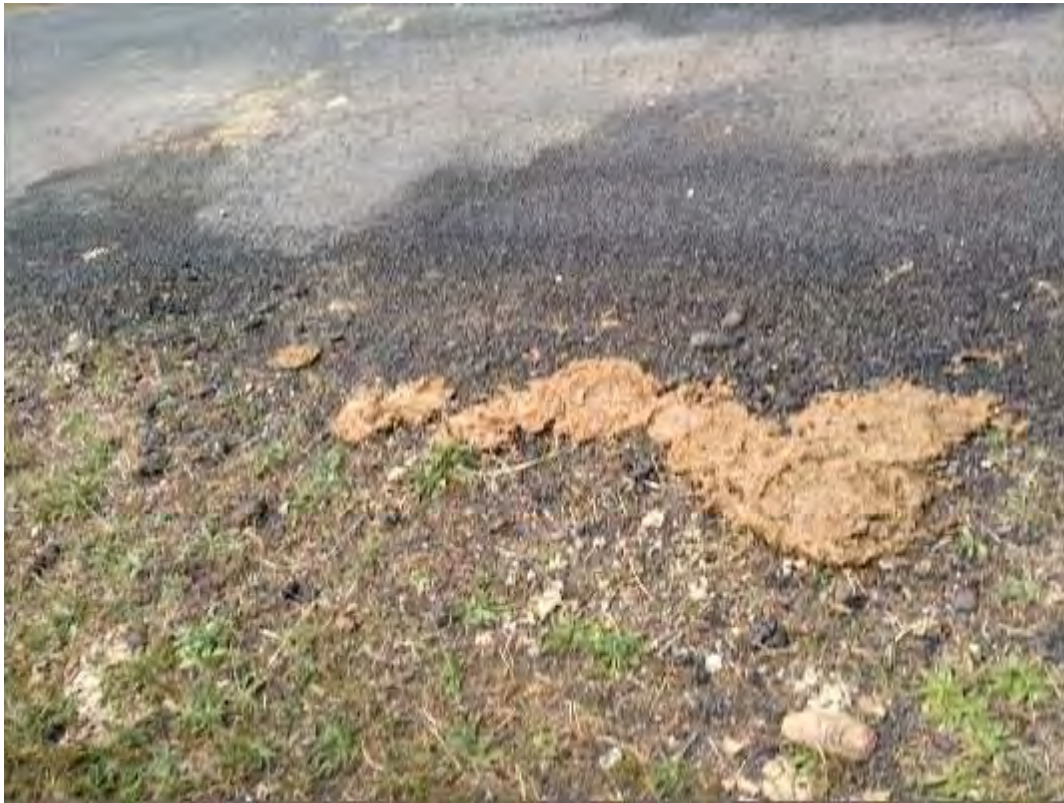
S202 – Evidence of Floodway
