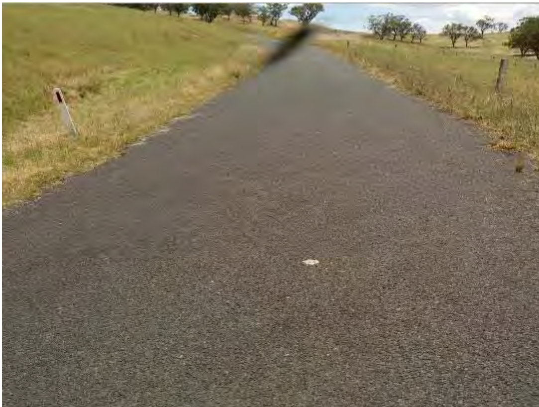
S221 – View to North
