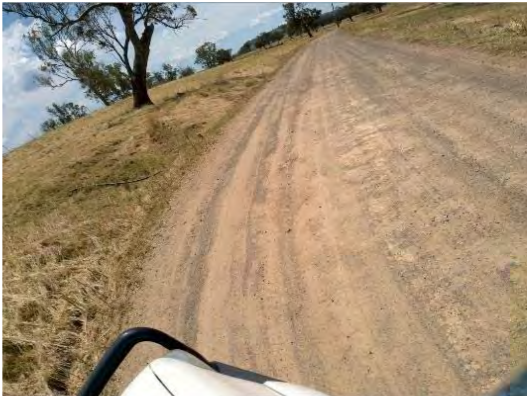
S211 – View to North
