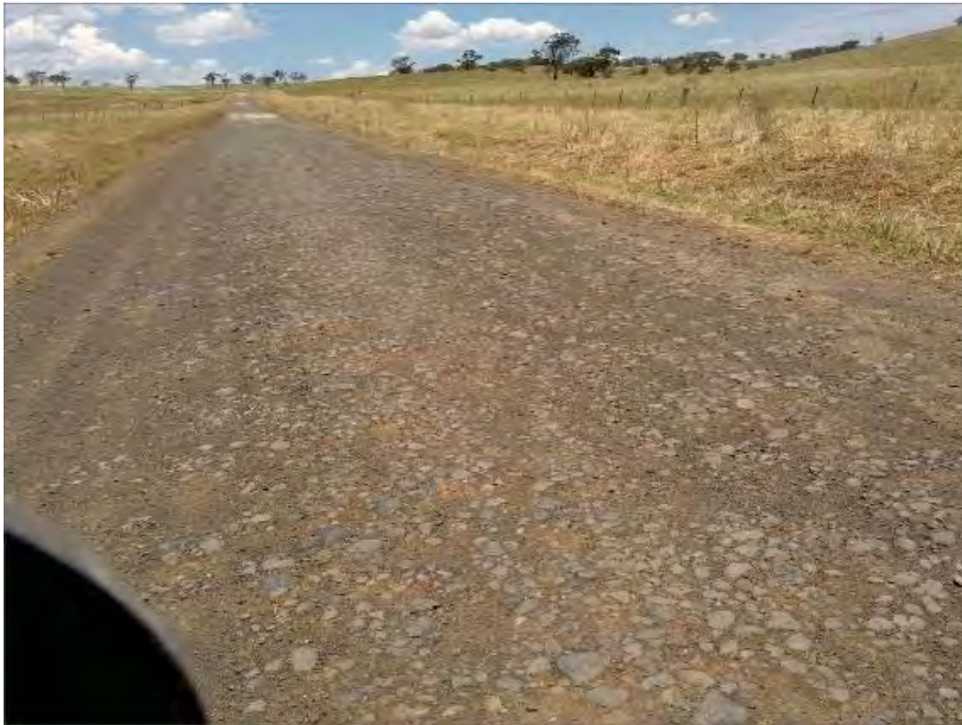
S216 – View to South, Causeway down to Sub-Base Material
