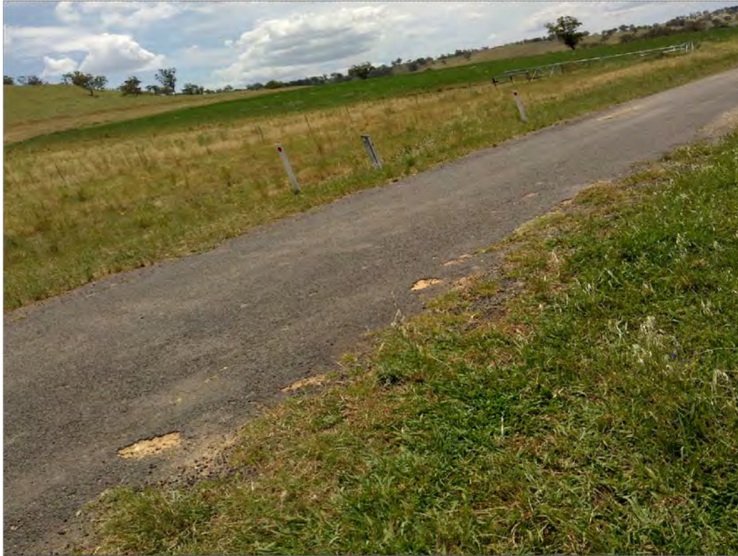
S227 – View to North
