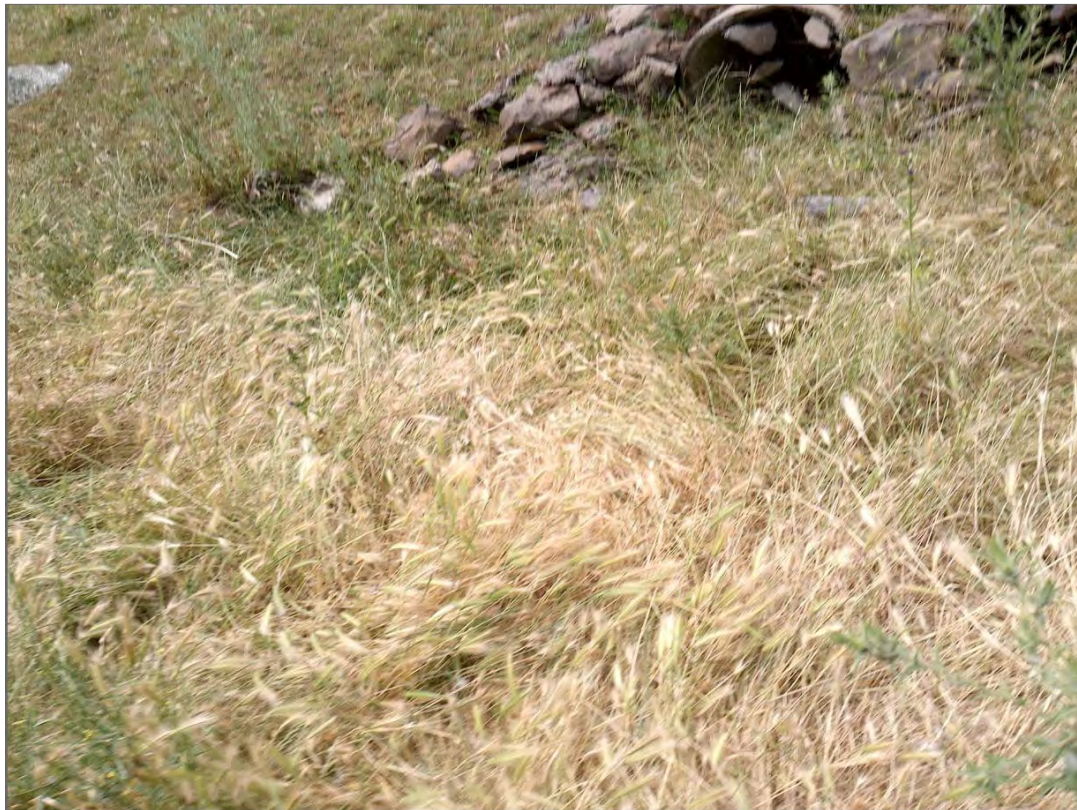
S199 - 600mm Pipe Culvert broken
