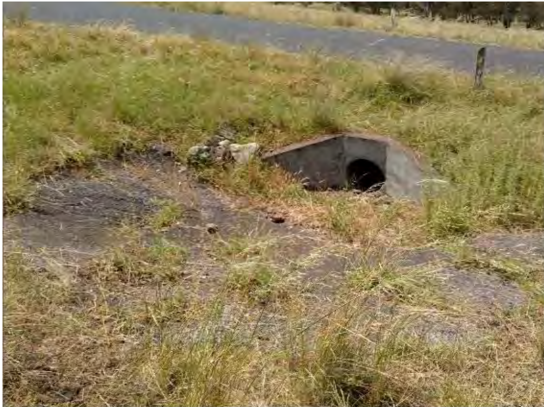
S224 - 450mm Pipe Culvert
