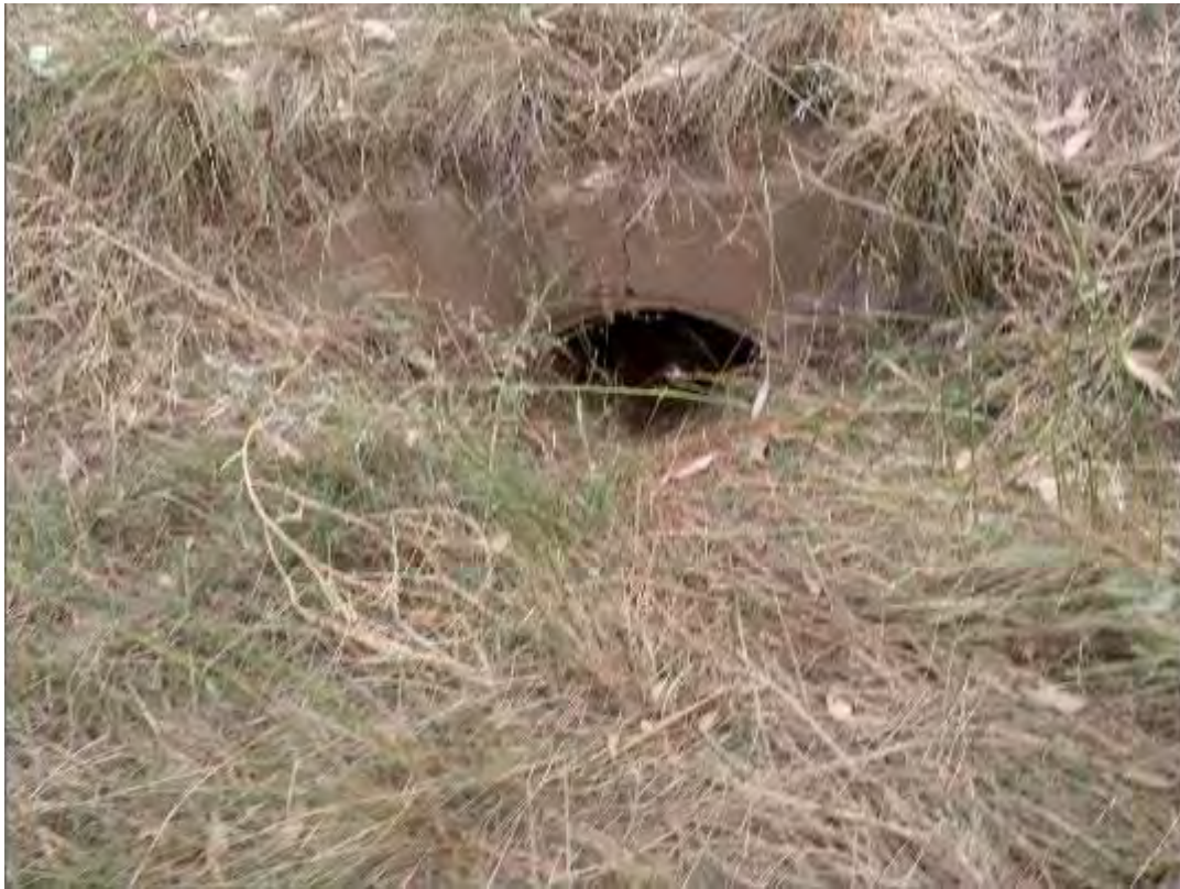
S239 – 525mm Pipe Culvert
