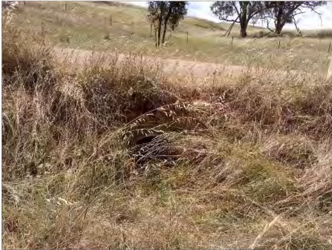
S254 - 675mm Pipe Culvert
