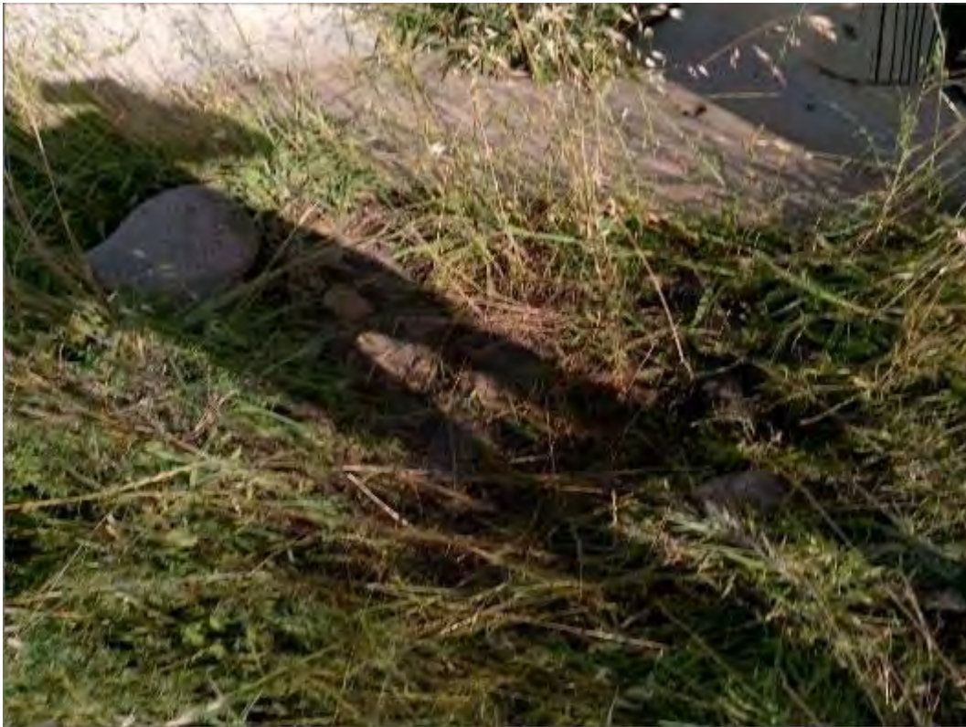
S067 – 600mm Pipe Culvert on top of image
