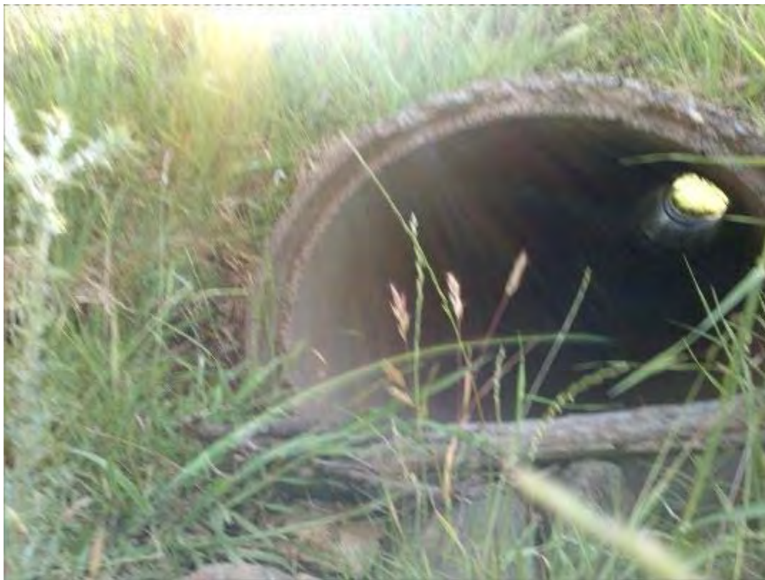
S057 – Internal View Level 2, 39 Sherwood Road Toowong QLD 4066
