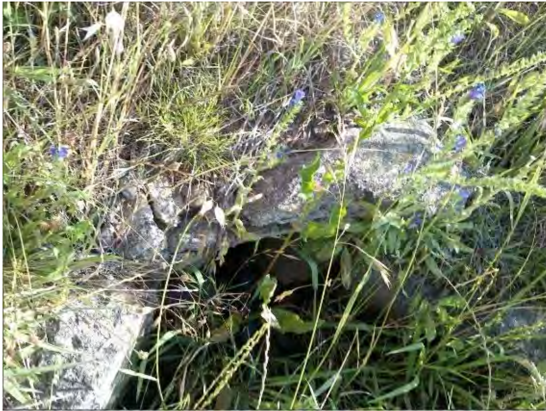
S068 – 450mm Pipe Culvert
