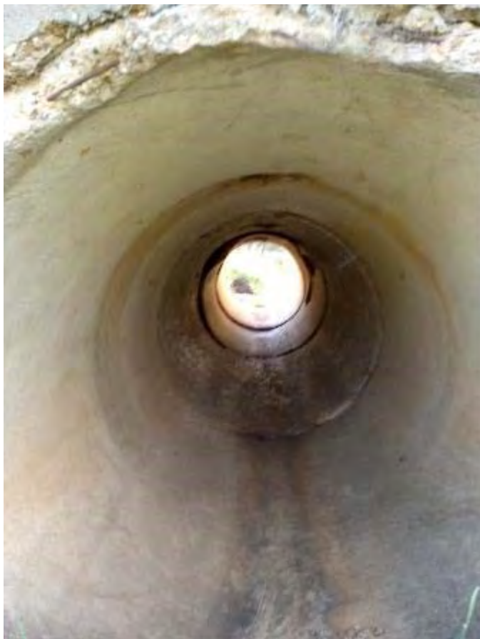
S053 – Internal View
