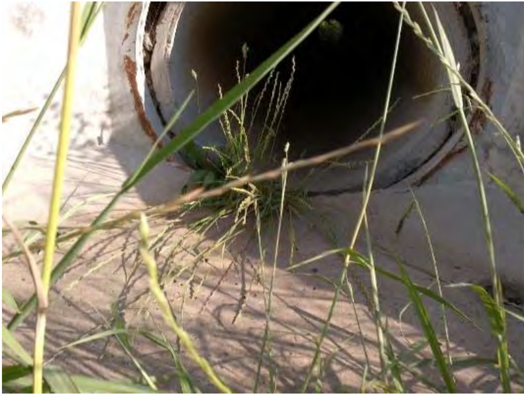
S066 – Internal View
