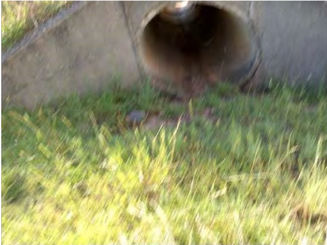
S053 – View of 1200 Pipe Culvert
