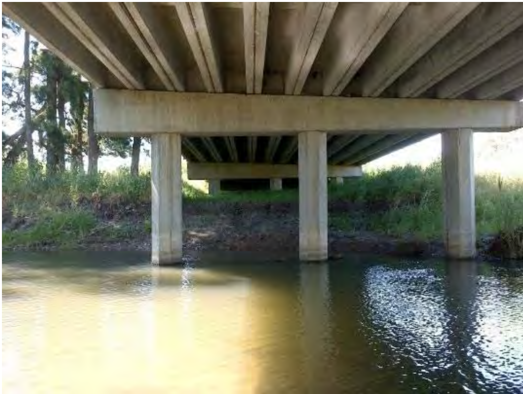
S045 – Soffit View
