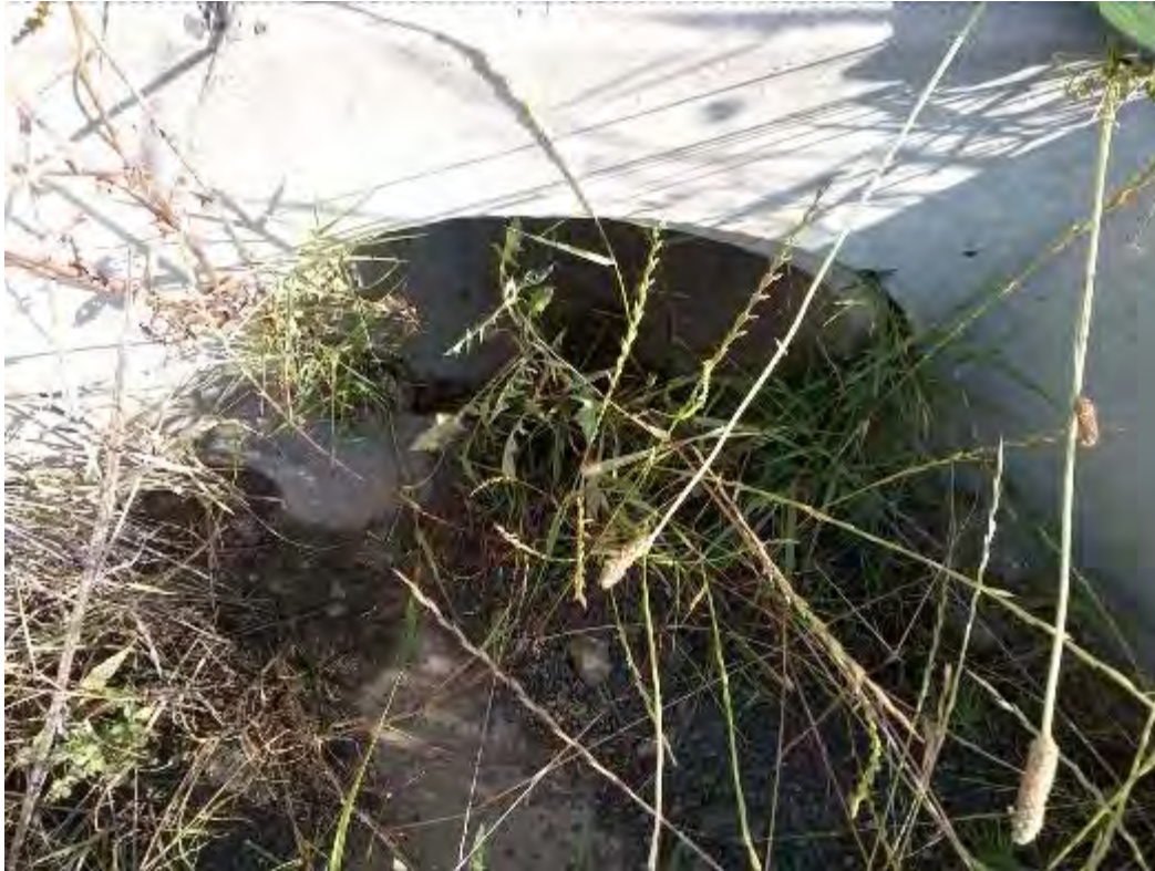
S070 - 450mm Pipe Culvert
