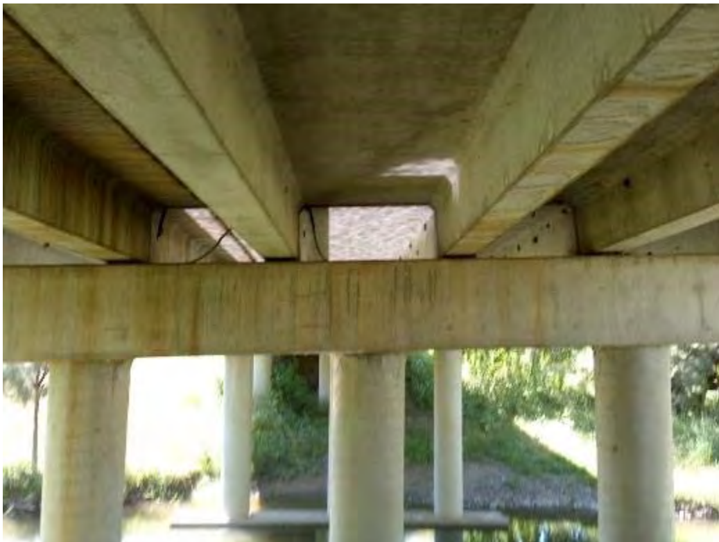
S042 – Soffit View
