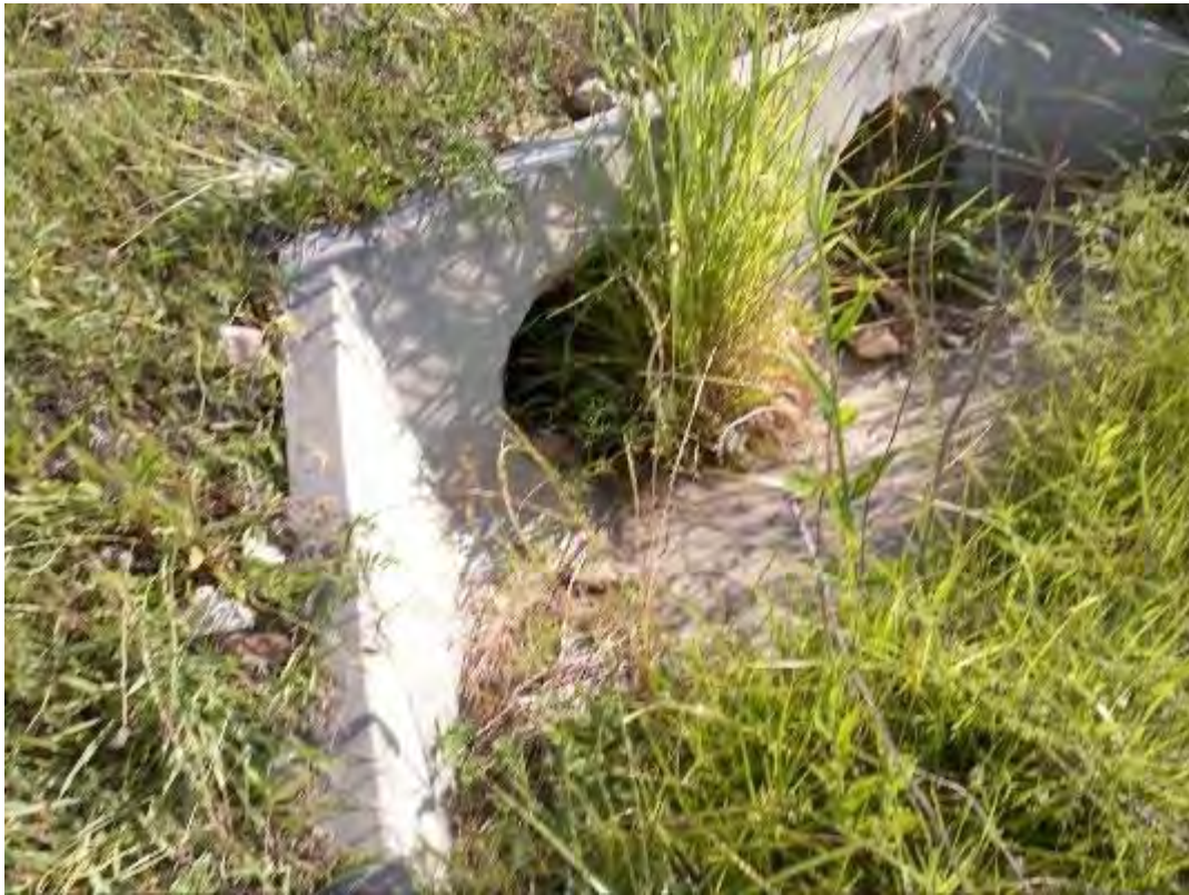
S069 - Dual 450mm Pipe Culvert
