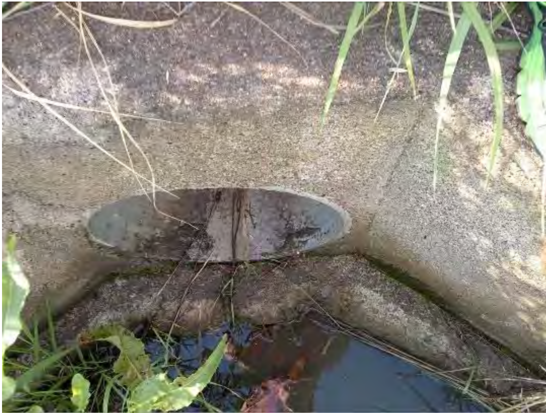
S071 - 450mm Pipe Culvert
