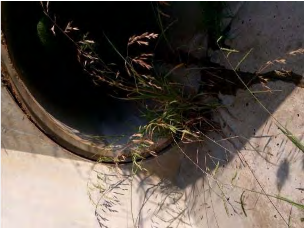
S065 – Internal View
