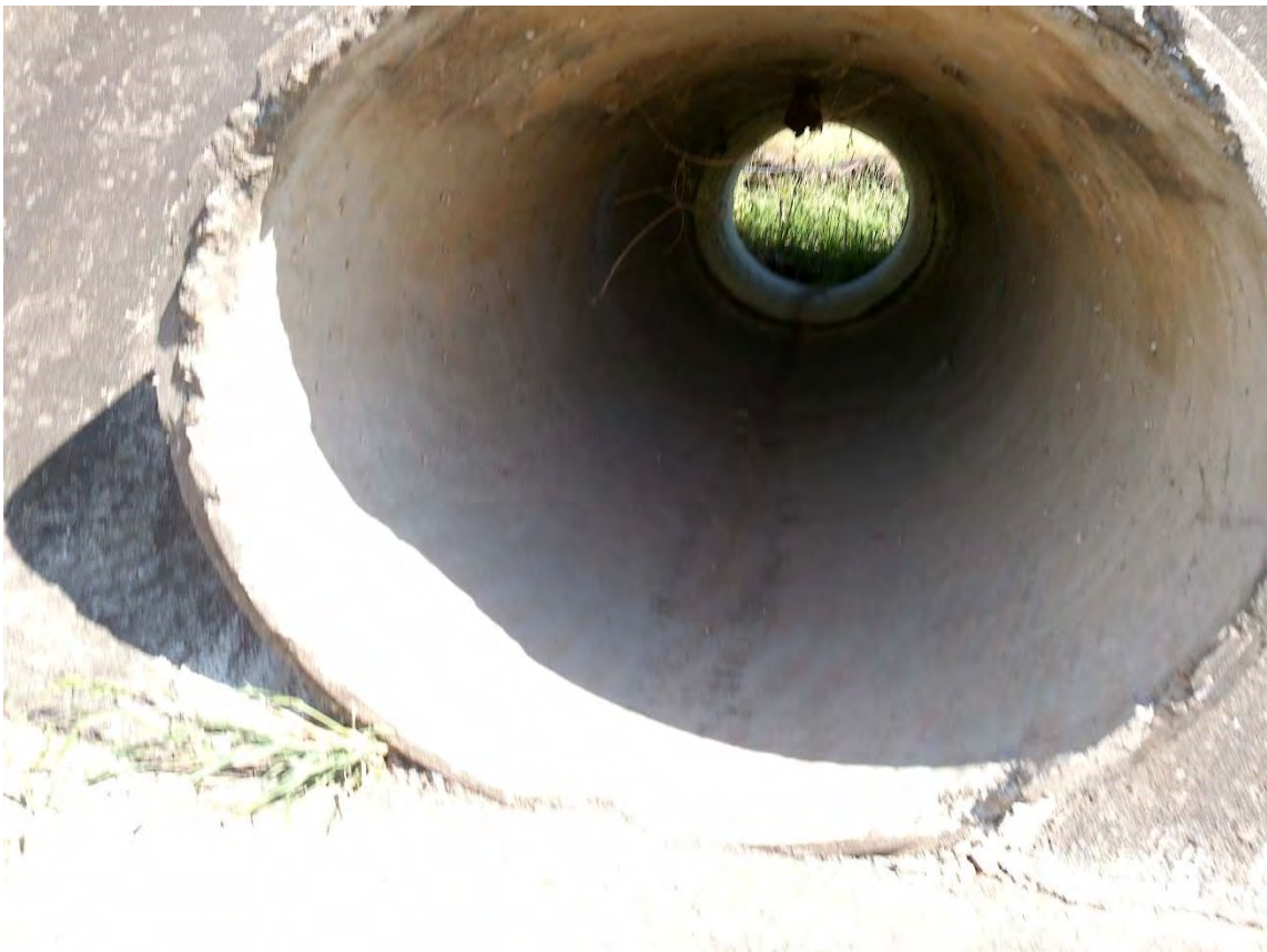
S038 – Interior View
