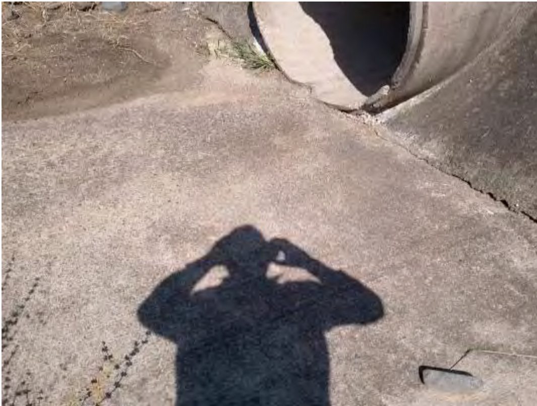
S038 - 1200mm Pipe Culvert
