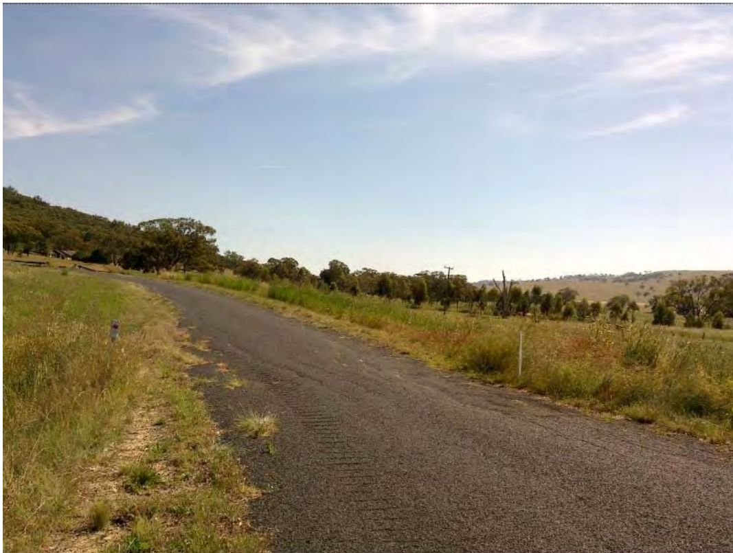
S019 – View to North
