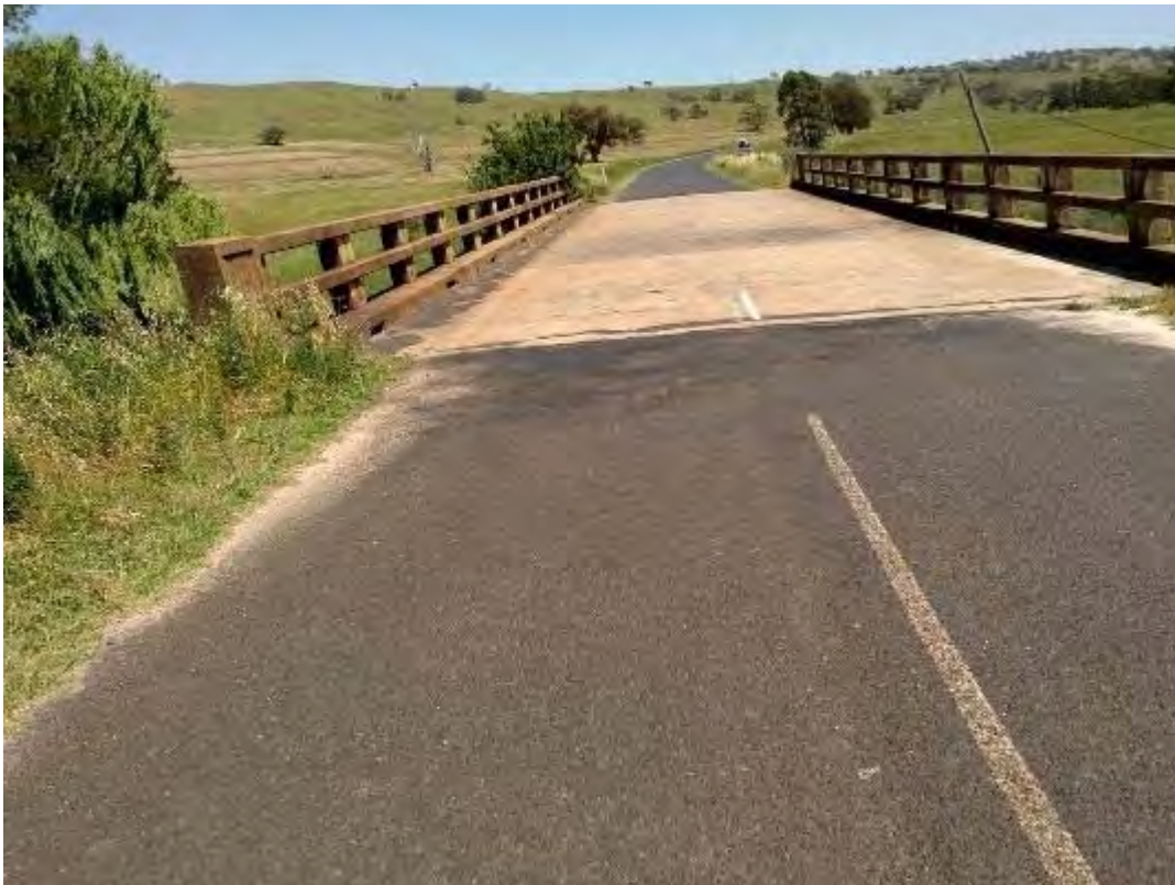
S036 – View to North
