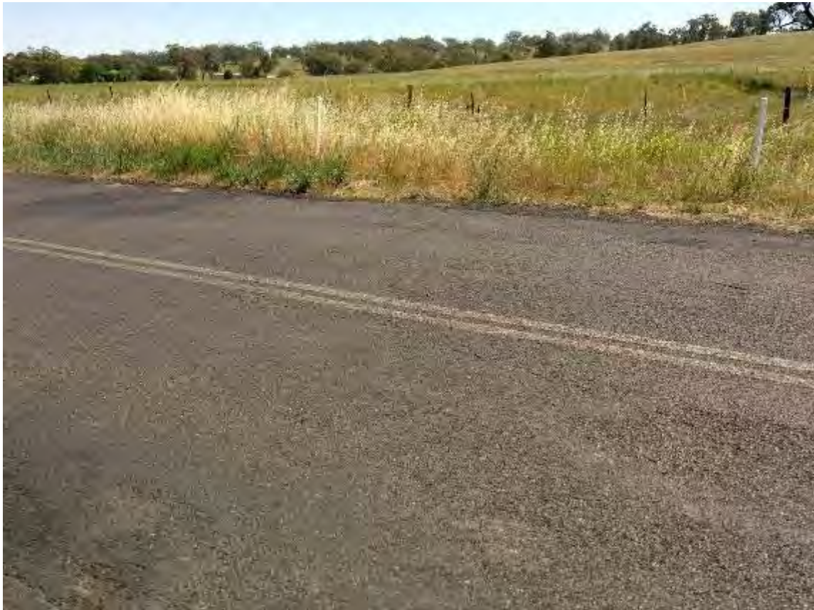
S016 – View North
