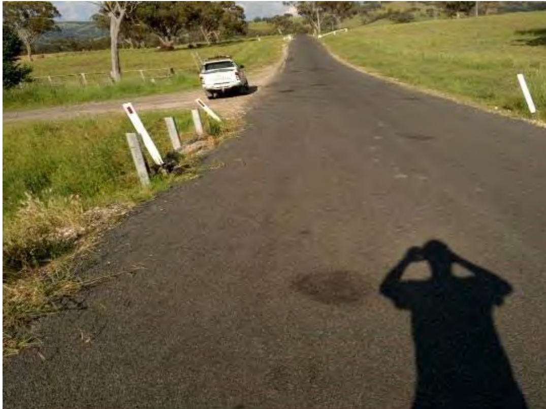
S002 - View to North
