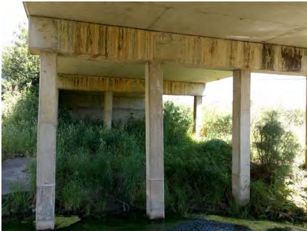
S036 – Soffit View
