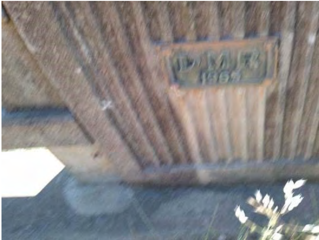
S036 – Bridge Label
