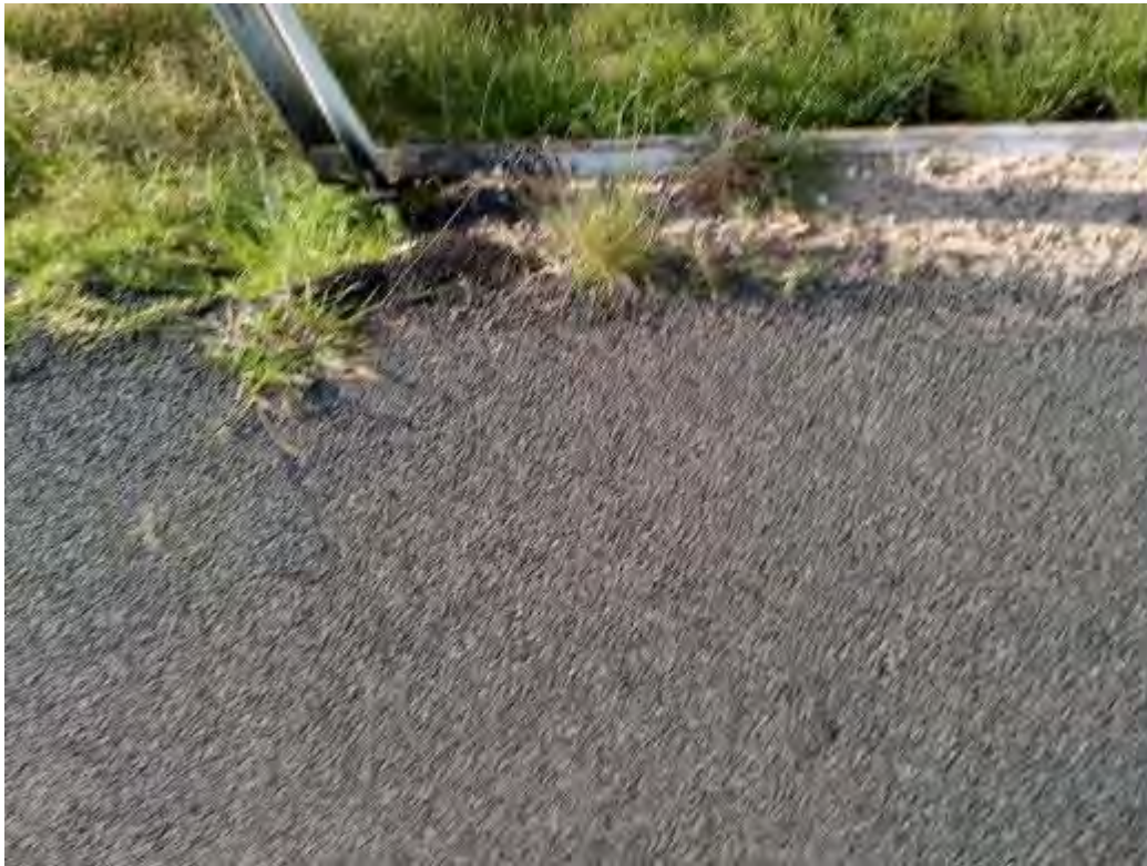
S002 – Edge View of Road
