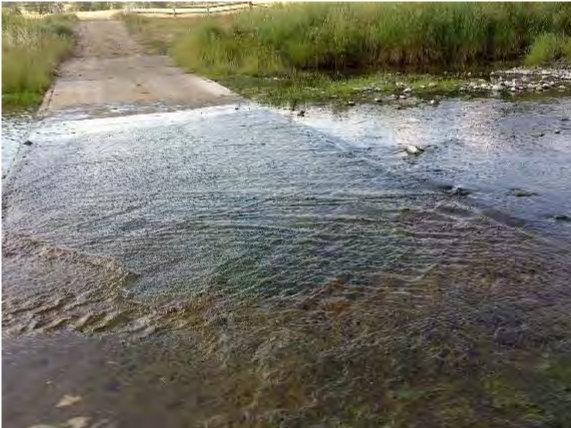
S004 – Top View of Causeway, Slippery Mossy Surface as Shown
