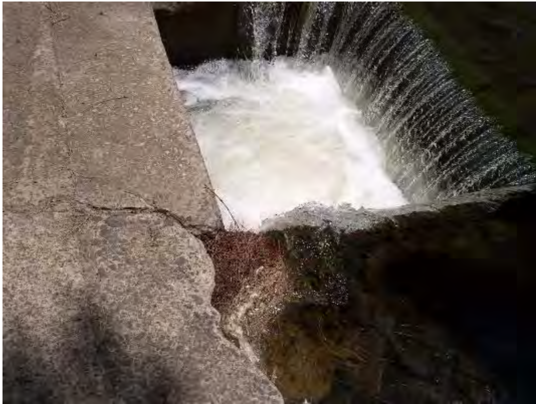
S025 – Invert Culvert
