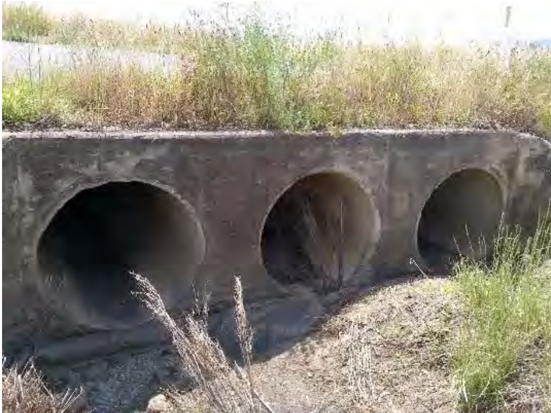
S011 –3-1050 Pipe Culvert
