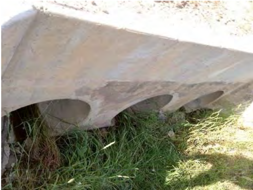
S003 – 3 - 900mm Pipe Culvert
