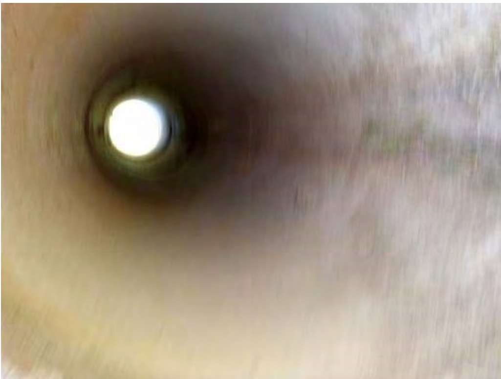
S002 – Internal View Good Condition
