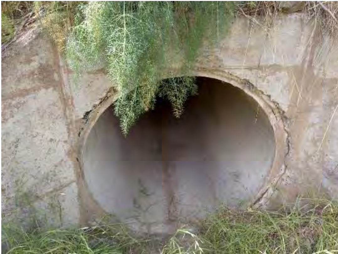
S013 – Single 1200mm Pipe Culvert
