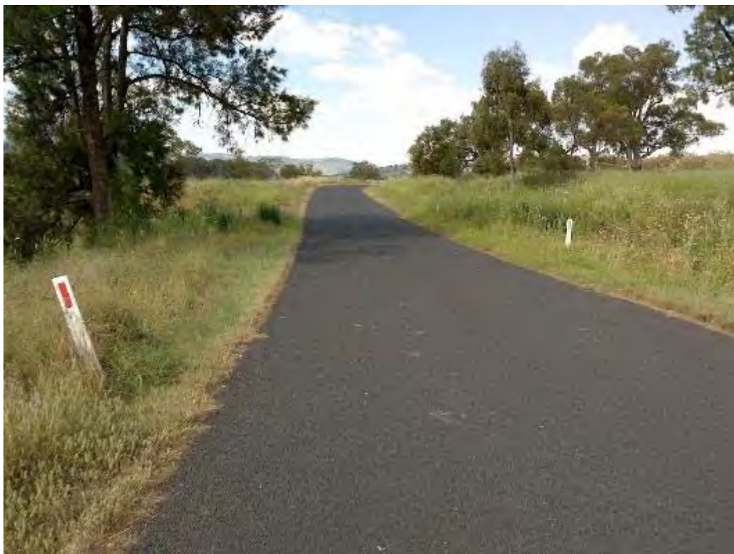
S008 – View to North
