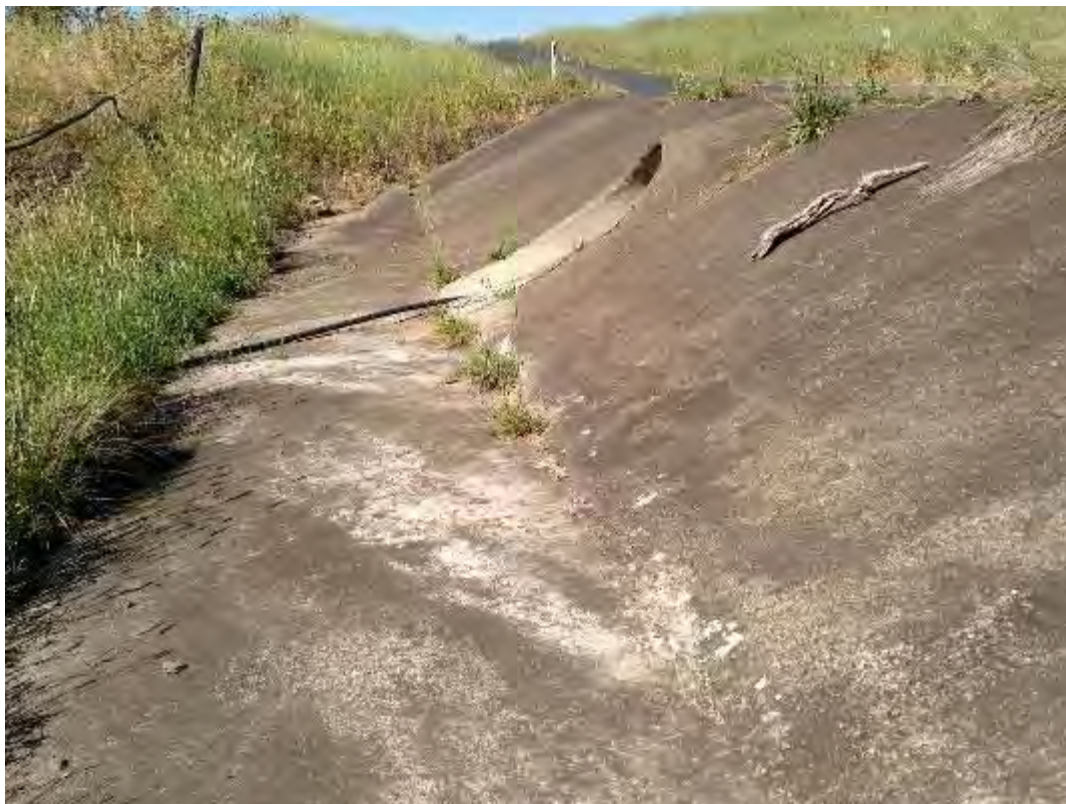
S037 – 1250mm Pipe Culvert
