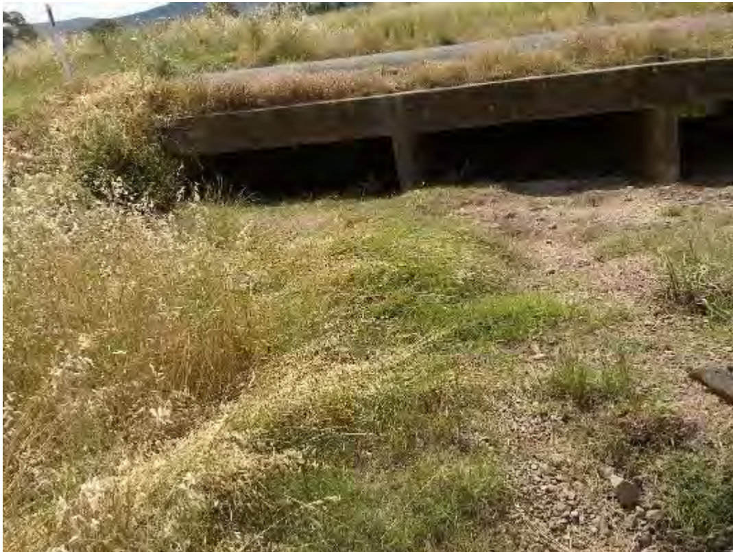
S012 – 3-750mm high-2400mm long reinforced concrete box culvert
