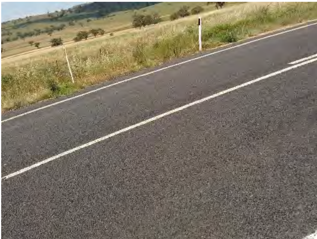
S013 – View to North
