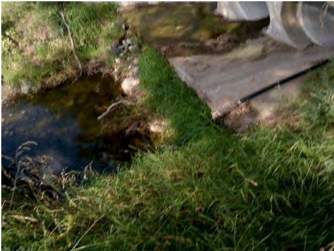
S008 – 3 × 1200mm Pipe Culvert
