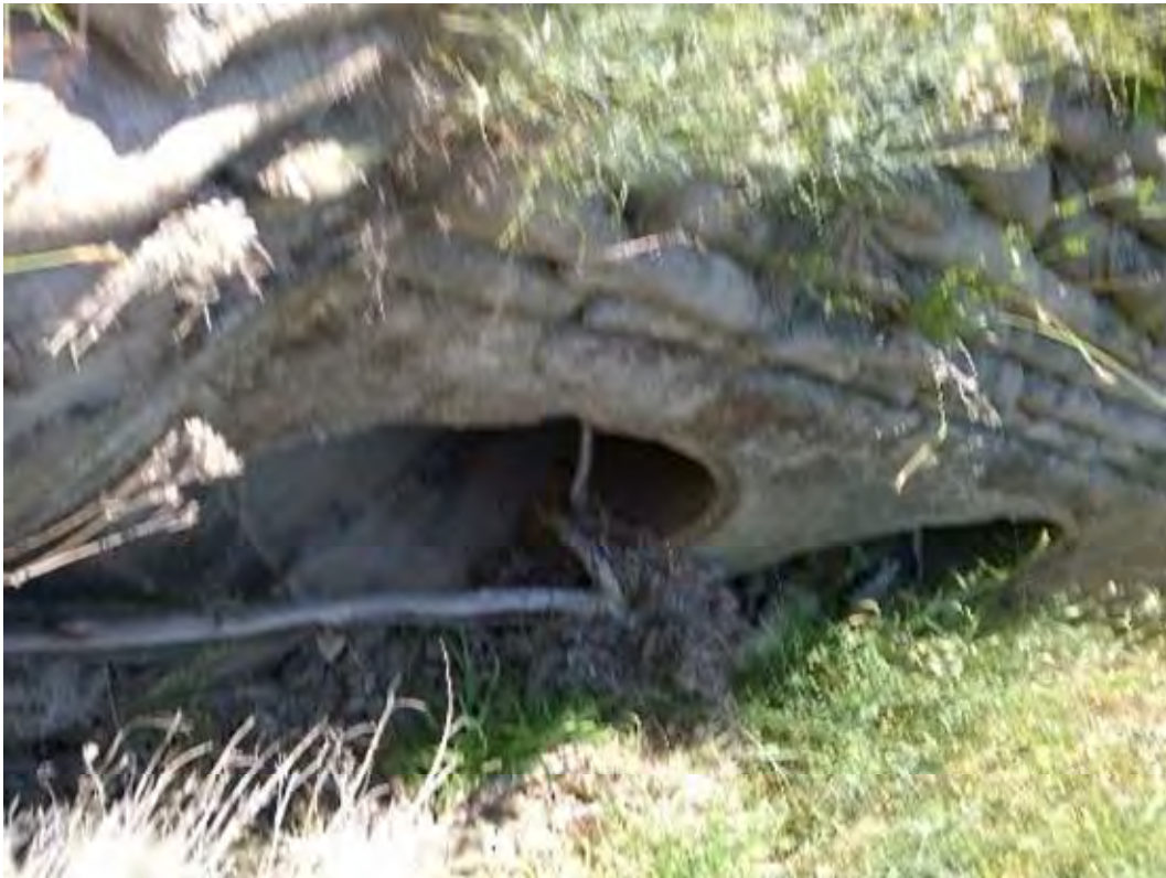
S014 – Dual 1200mm Pipe Culvert
