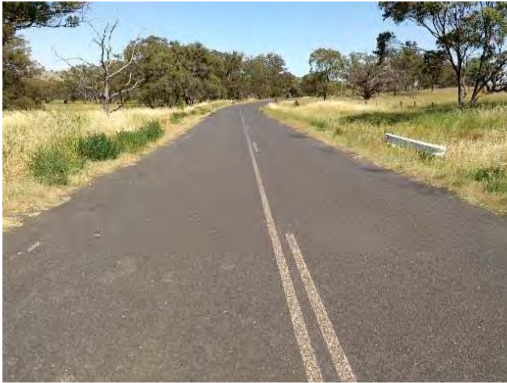
S017 – View to North-West
