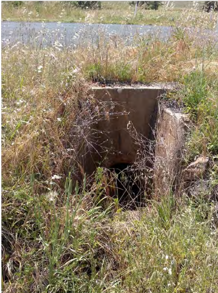
S015 – 450mm Pipe Culvert
