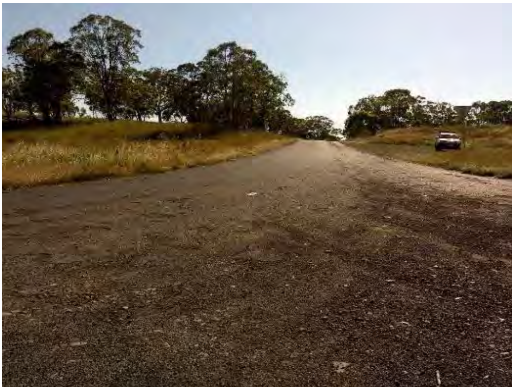
Figure 4.2.3 – View perpendicular to intersection towards Coolah Road
