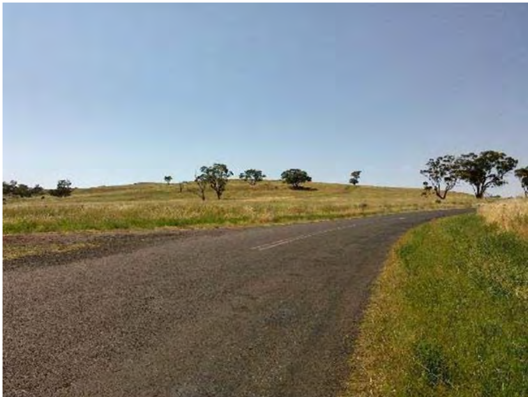
Figure 4.3.2 – View to South towards Vinegaroy Road
