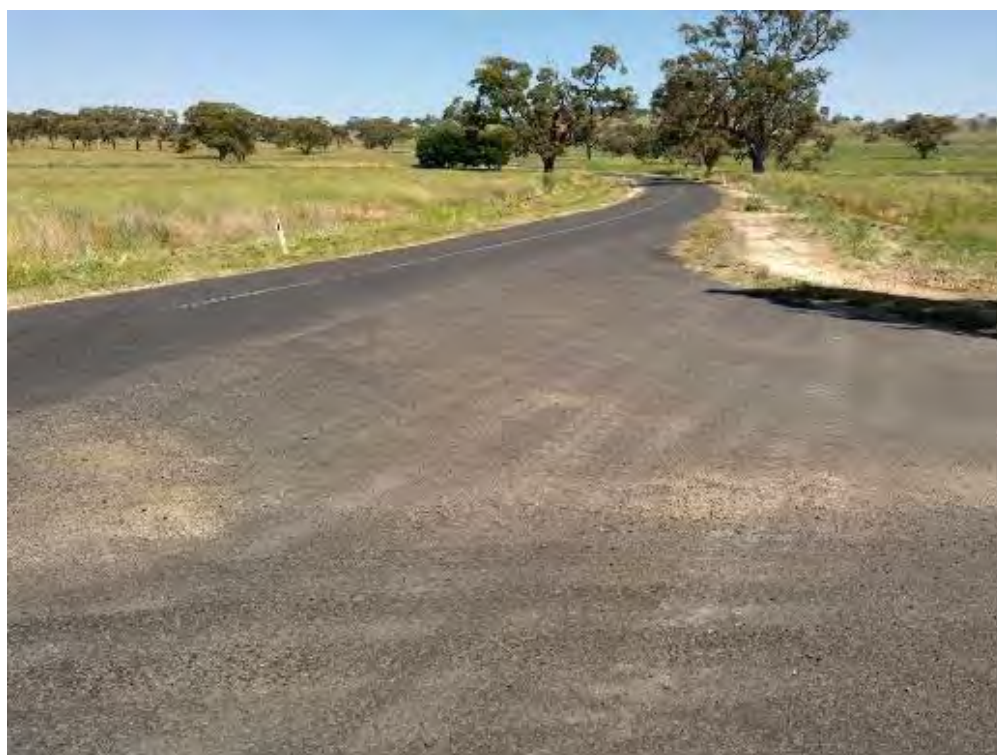
Figure 4.4.3 – View to North-West towards Vinegaroy Road
