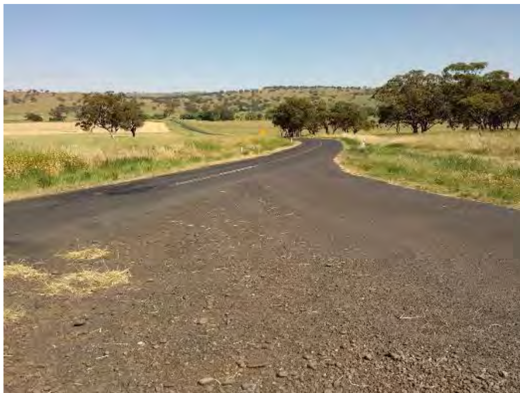
Figure 4.3.4 – View to North-West towards Vinegaroy Road
