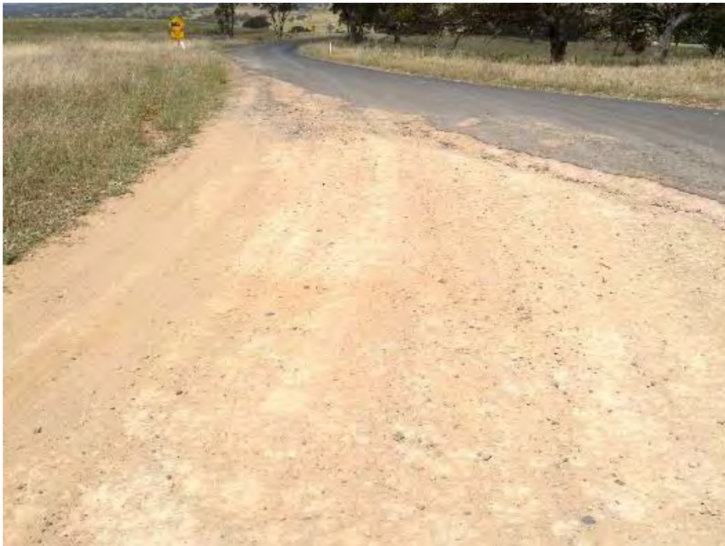
Figure 4.10.1 – View to East towards Coolah Road
