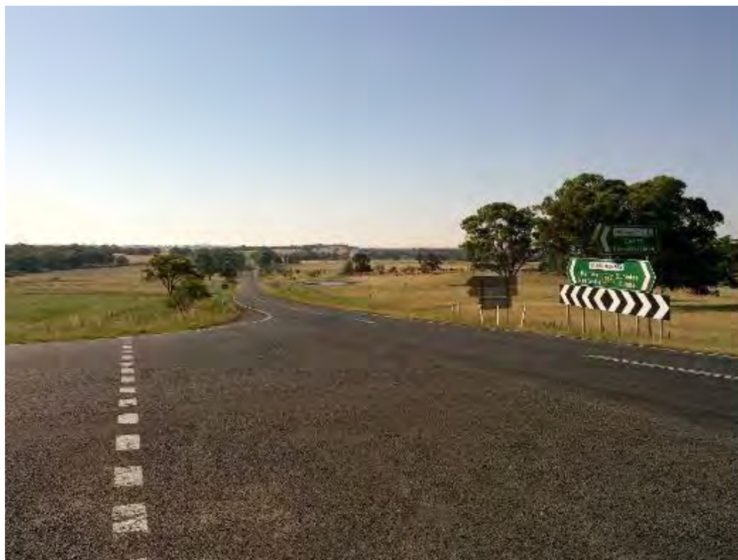
Figure 4.1.3 – View to East towards Golden Highway
