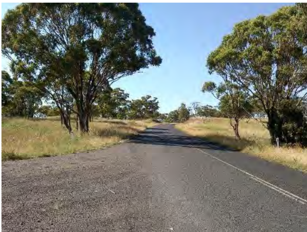
Figure 4.2.1 – View to South towards Vinegaroy Road
