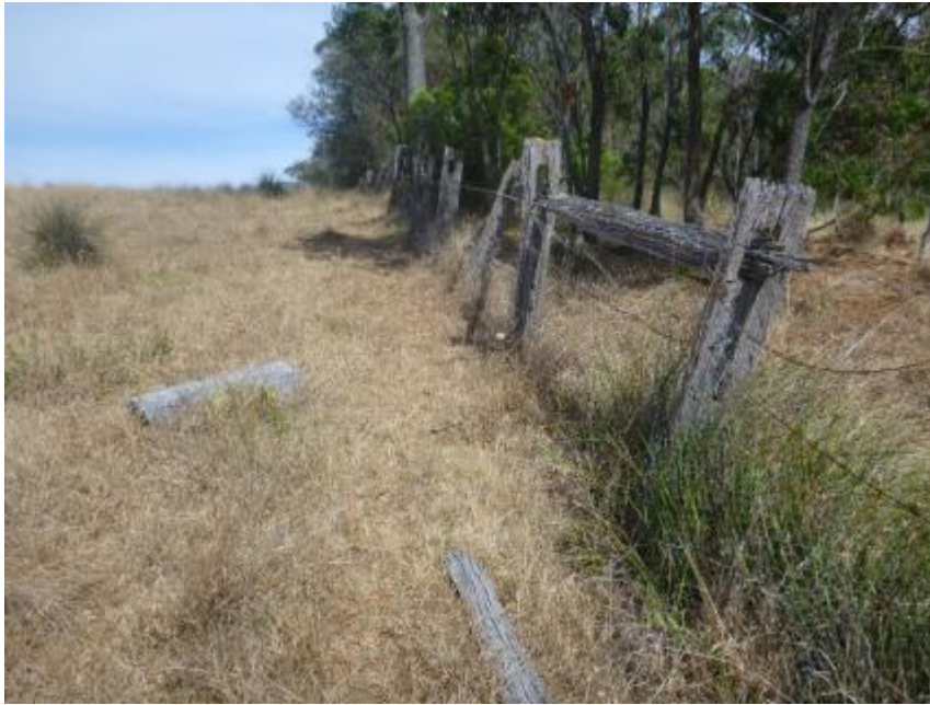
Plate 92 TL LU1/H1 looking west.
